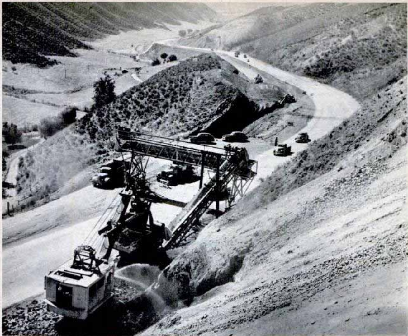
"BELT LINE" FOR GRAVEL. With an overhead conveyor spanning the road, traffic on a busy California highway moves along as usual while the road is being widened and straightened. The belt conveyor carries dirt and rock 20 feet above the four-lane pavement, permitting autos to pass beneath. Scene of the $763,000 project is the Ridge Route across the Tehachapi Mountains between Los Angeles and the San Joaquin Valley. Dirt is removed by a Diesel-electric shovel from one side of the road, and then deposited in trucks across the highway
