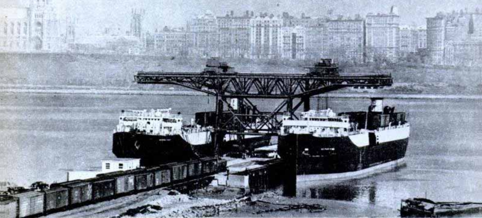
Steel framework at Edgewater, N. J., terminal supports two 125-ton cranes which load freight cars into seatrains
