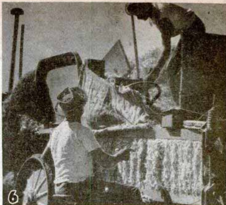
5.—Thresher operator sits atop machine. Large wheel is clutch. 6.—Threshed vines are baled for use as stock feed
