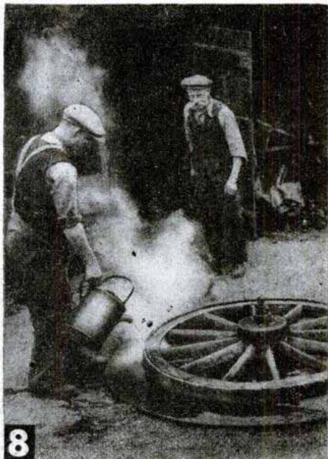
This is called "marking out fellies." Rim segments meet at center point between spokes After tire is fitted and hammered while hot, quenching with water makes it contract and fit
