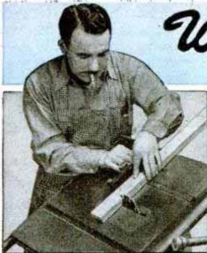
1 CUTTING A MITER
