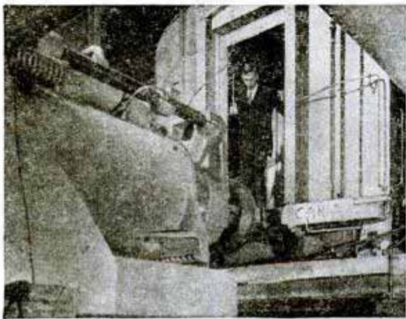
Diagram shows how a car 95 feet long is installed in the ram for a strength test. Below, the ram power unit exerts pressure against end of car. Right, engineer checks car during the test
