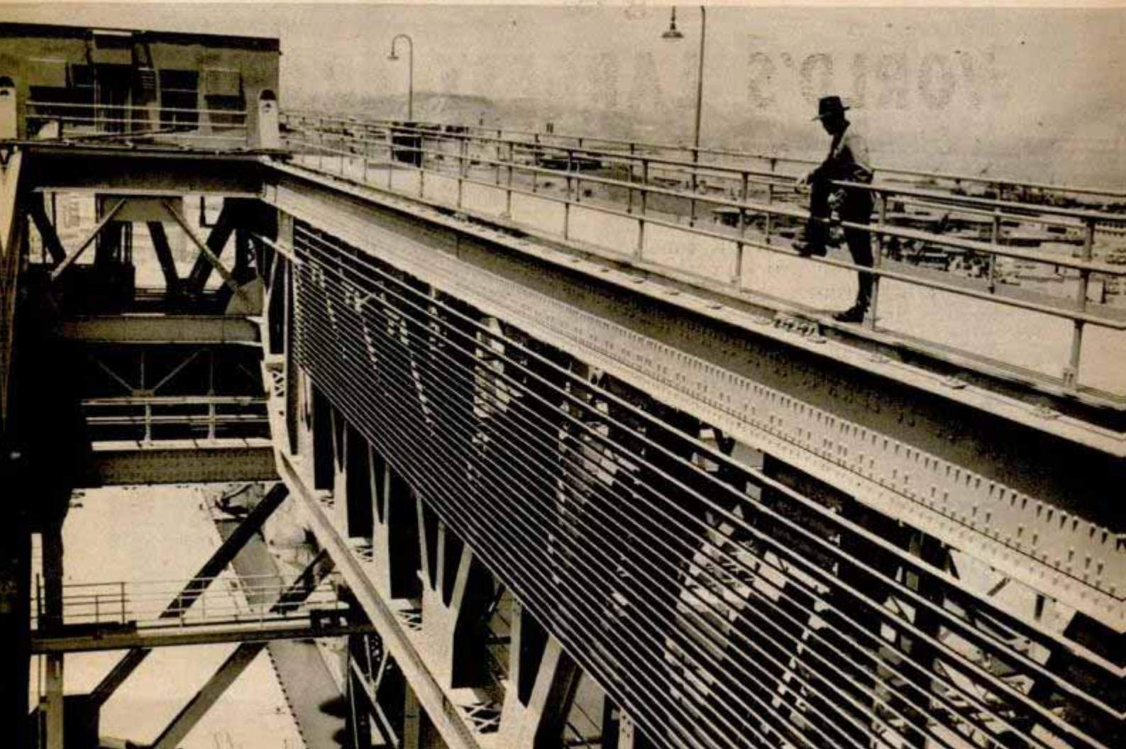
Berthed beneath the world's largest crane is the aircraft carrier Hornet, showing how the structure projects out beyond it. Tops of the trolleys that run on the crane are 207 feet above water. Below, long open slot inside the crane structure, on top of which one of the trolleys will move from side to side, dangling a main and an auxiliary hook downward. Parallel bars at the right will furnish the power
