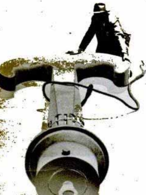
At left is the biggest hook of all, a 5-ton casting that will hang from the equalizer beam when weights near 400 tons are being handled. Right, 245-ton capacity hooks that will be suspended from each of the cranes
