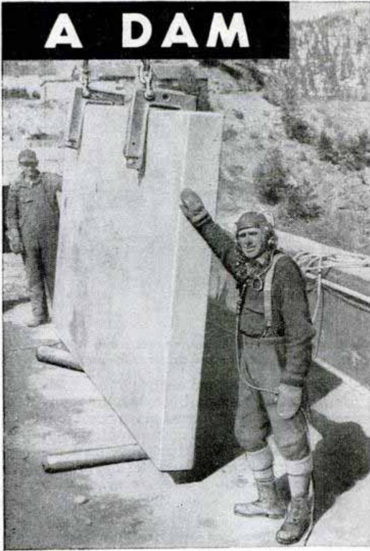
Precast concrete slab is ready to be fastened like a building block in the new face. Below, the dowels are welded together to hold the wall rigidly in place
