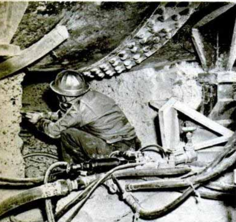
↑ Workman drills concrete before removing it in blocks ↓ Power unit weighing 450 tons is lifted from temporary installation. It was loaned to Coulee during war
