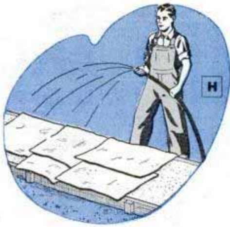
Cure concrete by covering with burlap. Keep the covering moist
