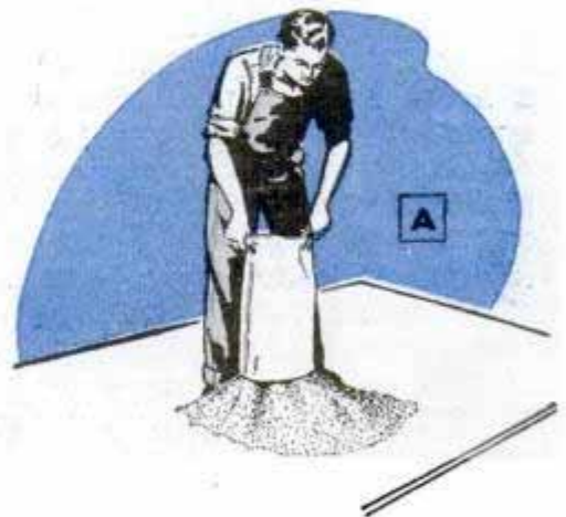
First add together measured amounts of cement, sand and gravel as at A above. Each bag of cement contains 1 cu. ft.
