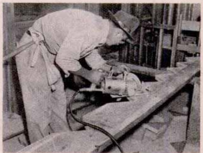
Here Jacques is cutting a stair stringer with an electric saw. A saw of this type will save much time
