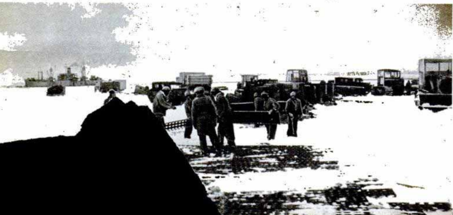
Metal airstrips devised in wartime facilitated landings and take-offs of heavy planes with wheeled gear
