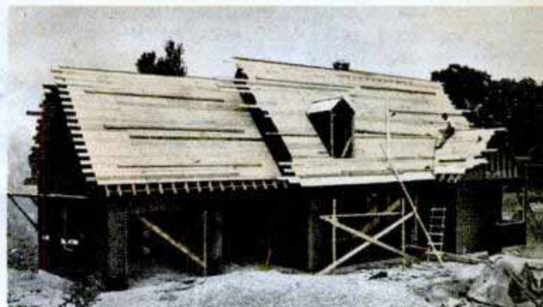
When the rafters and gable and studs are all up apply the rest of the sheathing and then put on the roof boards. Nail them close together and let the ends project. When installed, saw all of them off at one time to get a straight roof edge
