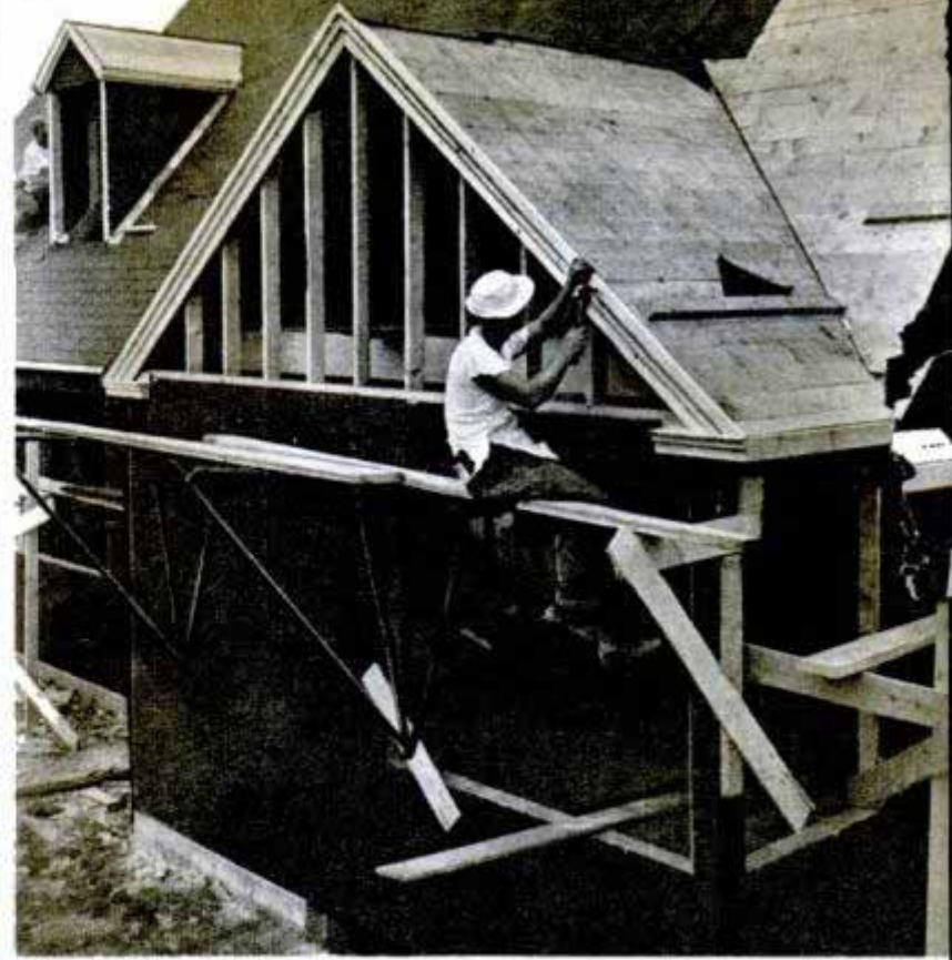
The photo above will give you some idea of how the small front gable is framed into the roof section. It is unnecessary to cut out the roof rafters for this. The other photo shows the gable end being trimmed.
