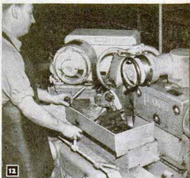
Valves from hard-driven engines are ground here
