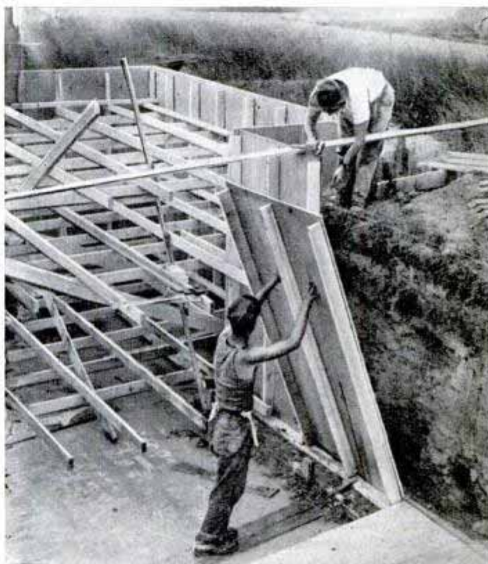
Plywood panels stiffened with 2 by 4s make good forms, and later can be used as a subfloor. The excavation walls serve as the forms on the outside. Bracing the forms as below makes it unnecessary to cut the stock and thus ruin it for use in the house
