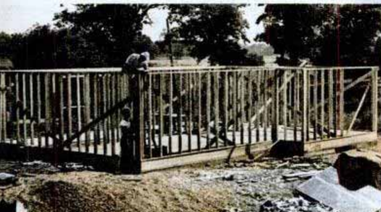
Plywood used in the concrete forms is laid on the joists for the subfloor, and then the wall studding is put up. The studs are assembled in panels on the ground and then erected. Triple studs should be used at all the corners for strength
