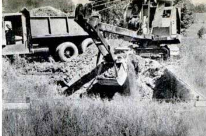
A mechanical scoop makes quick work of digging the excavation. You will have to do some shovel work, of course, to square up the sides before the forms are set
