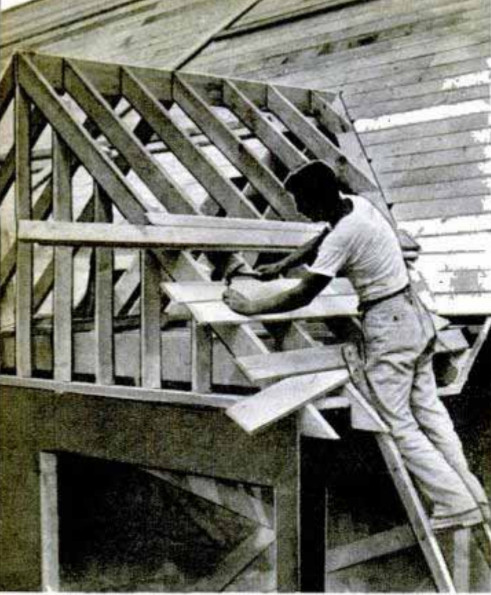
The photo above will give you some idea of how the small front gable is framed into the roof section. It is unnecessary to cut out the roof rafters for this. The other photo shows the gable end being trimmed.
