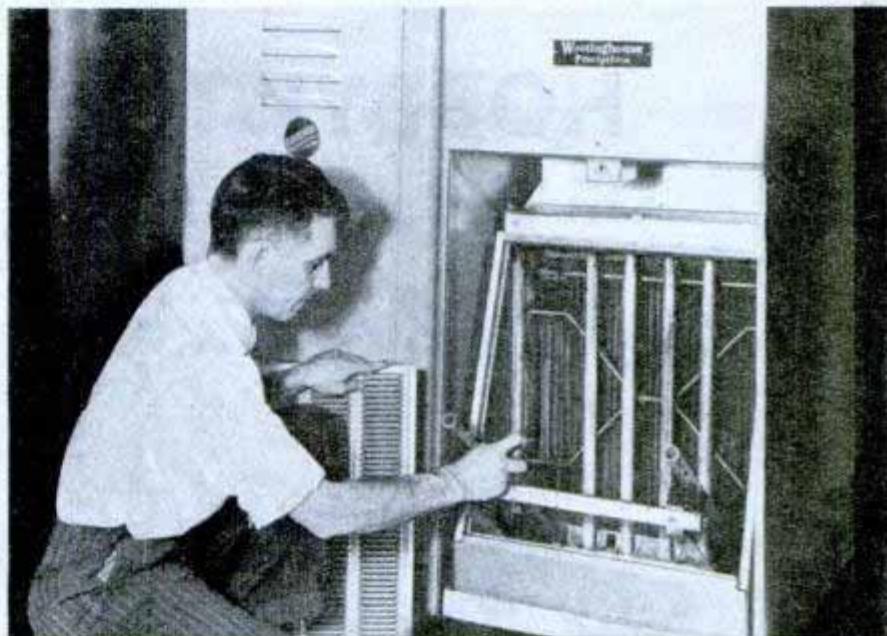
HOME AIR CLEANER picks up 85 percent of dust entering house. Dust is electrically charged, then attracted to metal plate
