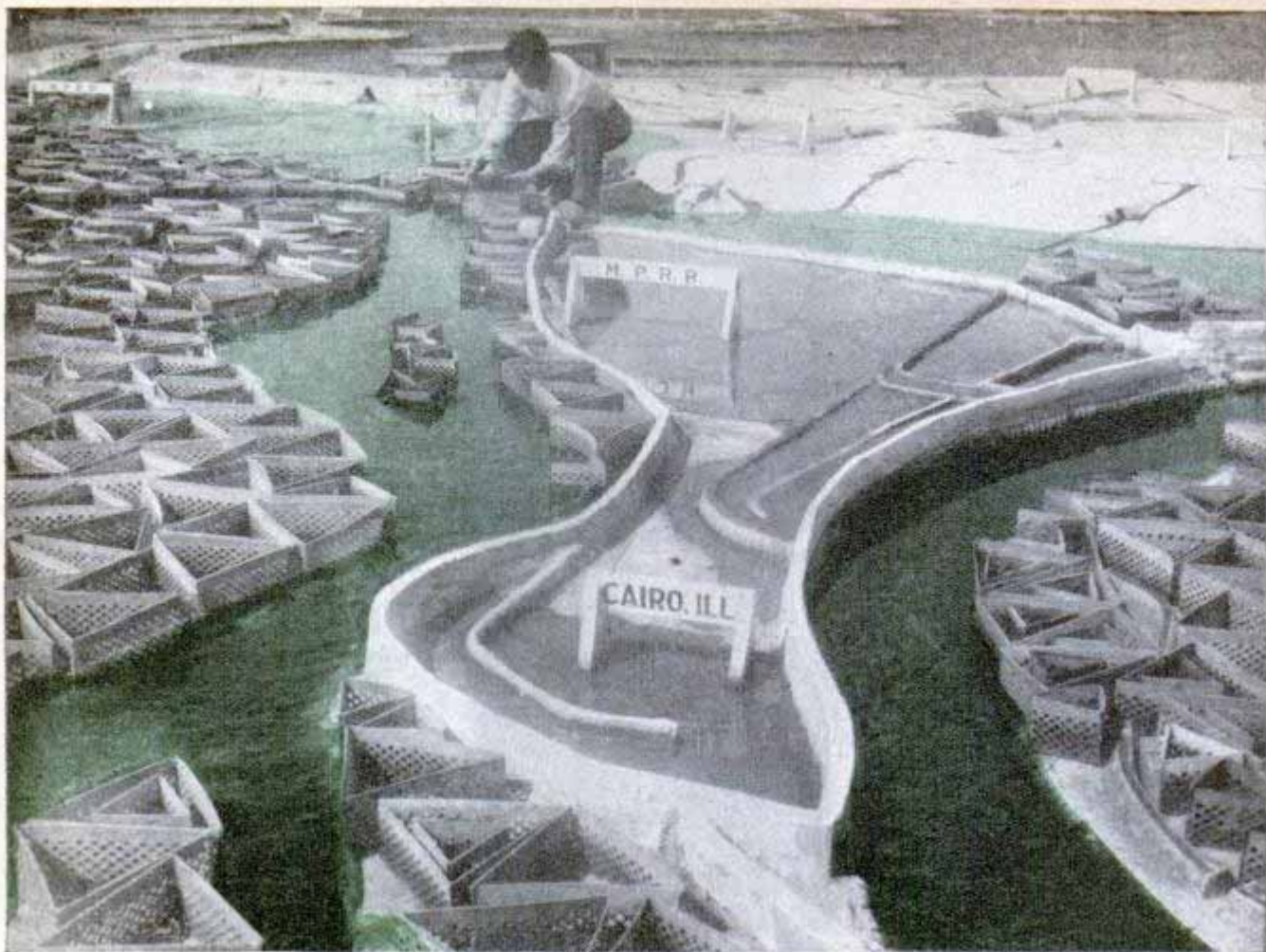
The mighty Mississippi River is reproduced in miniature in model studies of flood control for Cairo, Ill. Below, testing model of New Jersey canal and locks
