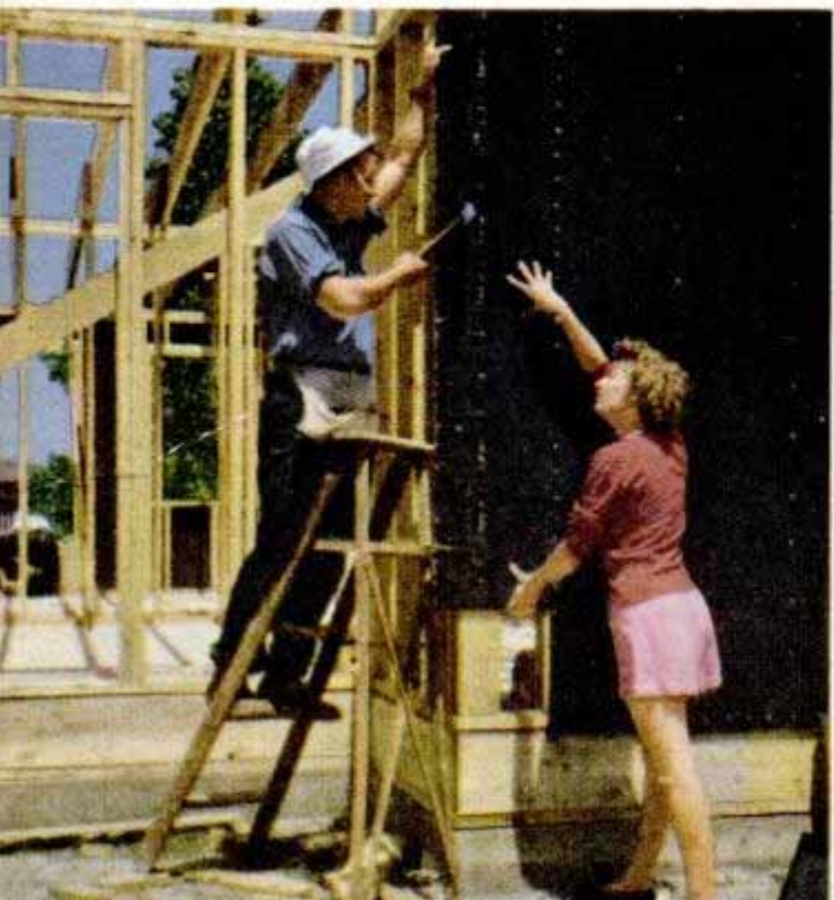
One of chest units which Jacques built for bedrooms is set into wall. Below, applying sheathing
