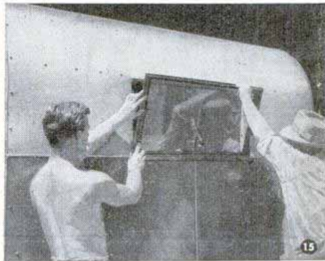
Rather than bother to make them yourself, buy the sash ready-made. These are all metal and come with the frame and sash in one unit. Fasten with screws
