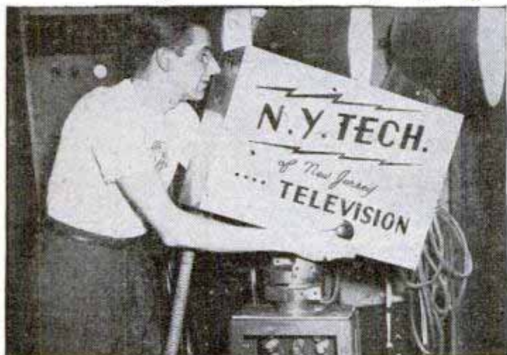
Ex-G.I. taking pictures with N.Y. Tech's Iconoscope Television Camera, which is used in the resident school's course entitled "Transmitters and Camera Technique."
