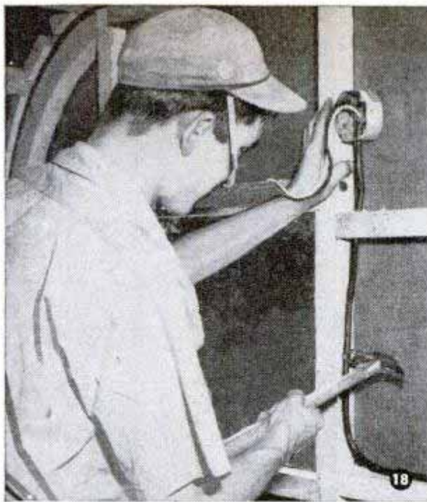
Wiring is carried through holes bored in the studs and frame members. Long runs should be stapled
