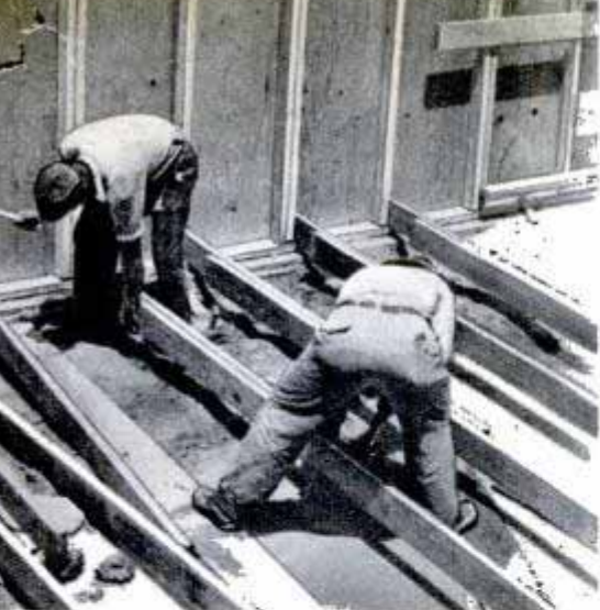
JUNE 27 —"Finished foundation forms for house and started forms for porch"
