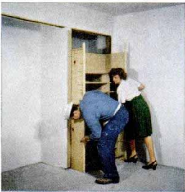
One of chest units which Jacques built for bedrooms is set into wall. Below, applying sheathing
