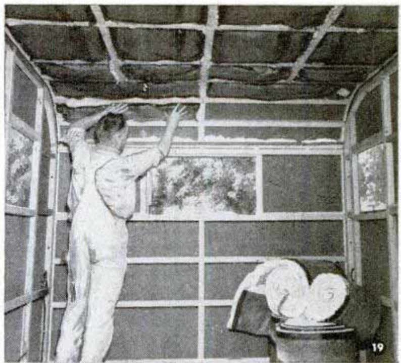
After wiring is installed, auto-body insulation in quilted form is pressed into place between the studs and roof members
