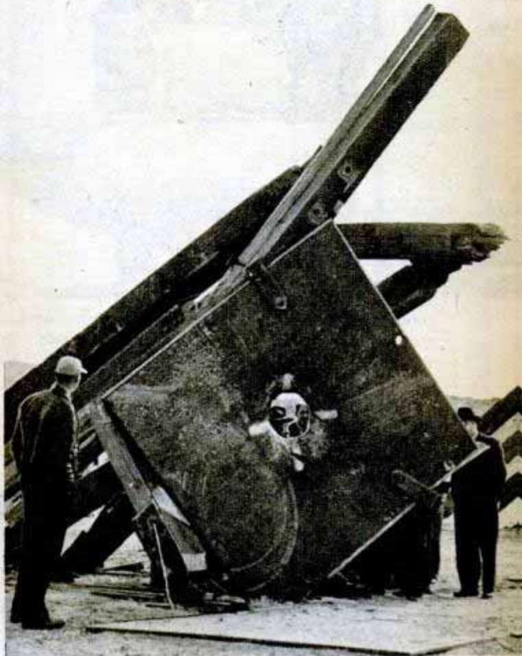
↑ Note marks left by fins when rocket penetrates target ↓ Ordnance experts examine opposite side of the armor
