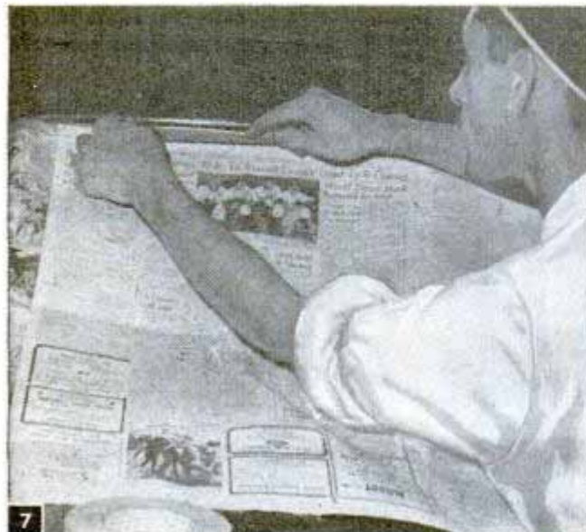
Above, mask glass and trim, using masking tape to cover small parts and to hold newspapers as below
