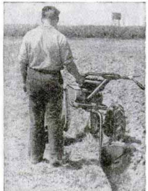
Handlebar controls on two-wheel tractor allow operator to walk to one side when plowing or cultivating
