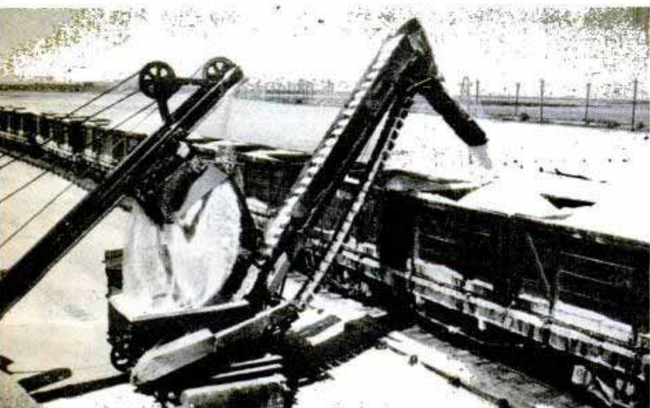
Power shovels load long strings of ore cars with salt taken from a high stock pile of crystals on the beach of Great Salt Lake
