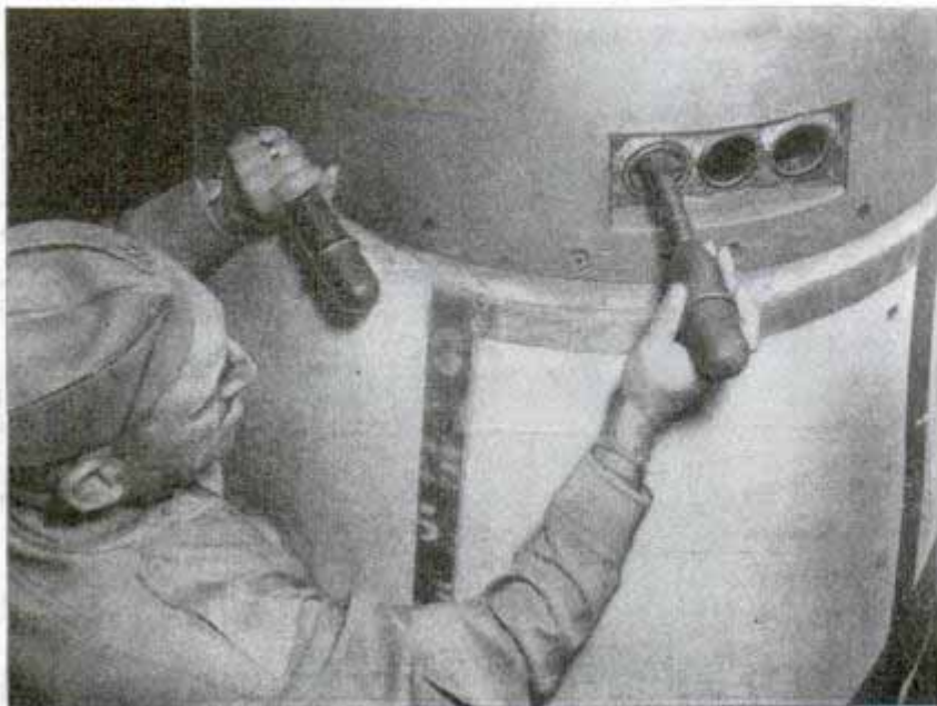
Artificial meteors in rifle grenade cases are inserted in the warhead
