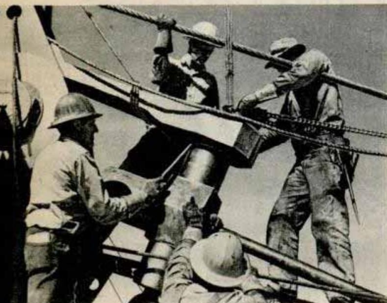
High over a raging river, riggers dismantle a construction trestle with same freedom of movement an average man has on the ground. Below, fastening cableway
