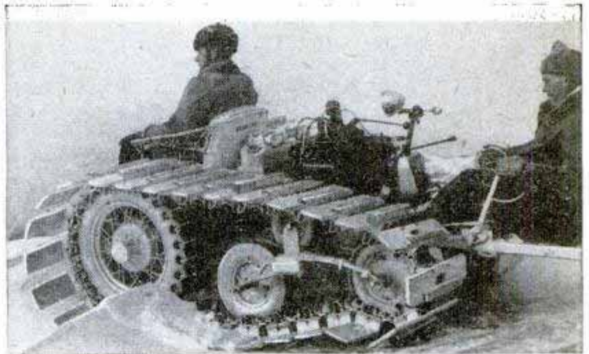
Indian princess and her companion enjoy their first ride in the Far North's snow vehicle. The cleats on the broad flat tracks give traction in softest snow
