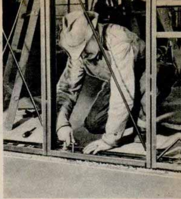
Steel wall frame is bolted to foundation
