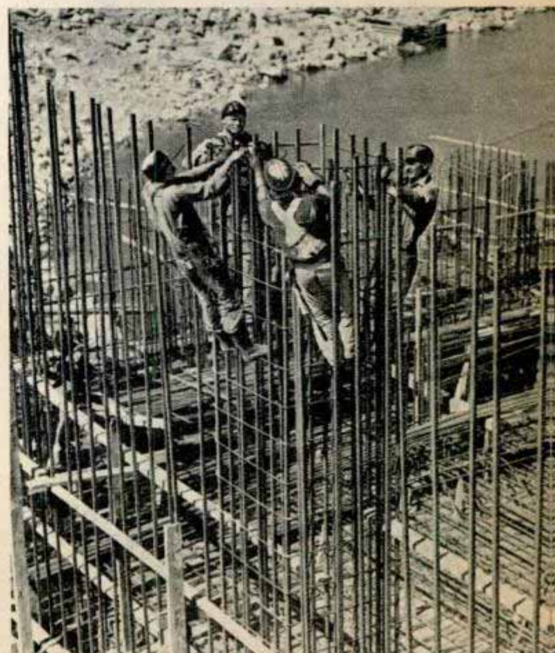
Setting reinforcing for walls and columns of a dam
