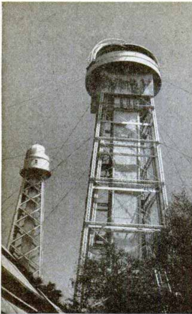
Two sun towers (150-foot unit at left and 60-foot tower at right) are used in solar studies at Mount Wilson
