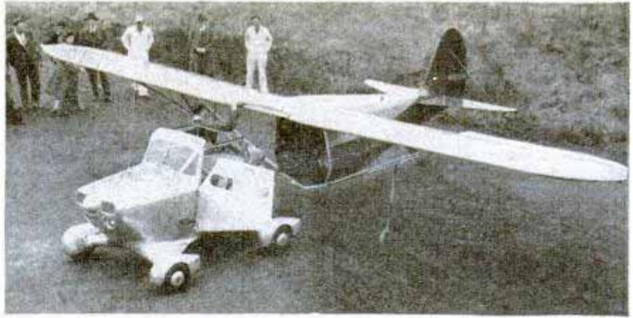
As a two-passenger automobile, left, the Airphibian can go 750 miles on a tank filled with 30 gallons of gasoline. Converting it from air to road use requires disconnecting two locks and takes five minutes. The silver colored, aluminum bodied coupe has a roll-back canvas top
