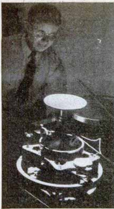
Sun's image is studied as it falls on white disk (left) at base of Mount Wilson's 150-foot tower. Right, electrically driven time clock automatically exposes frame of motion picture film in the Climax coronagraph
