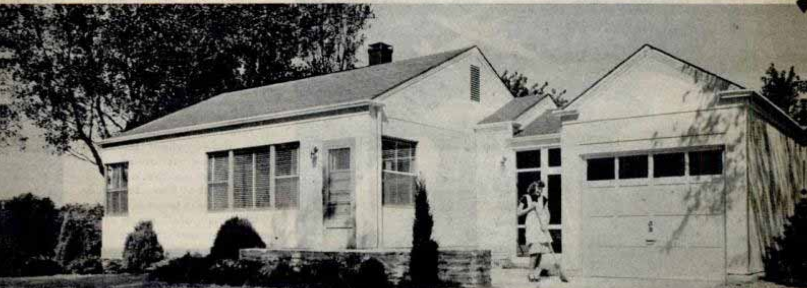
↓ Although this is the standard size for the Butler aluminum house, a complete wall panel can be removed in a few hours and extra panels added to both walls and ceiling to increase the size of a room or the entire home
