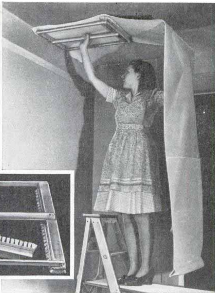
Brushes smooth paper against ceiling so that it dries without wrinkles
