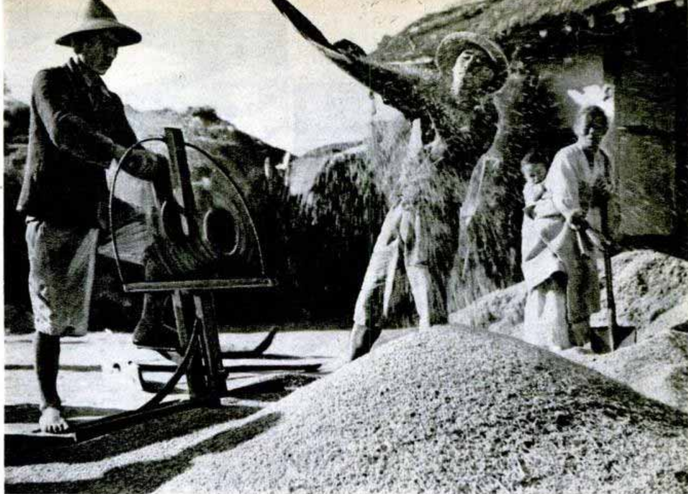
Korean farmers, top, blow small pieces of straw from threshed rice with foot-powered propeller. In modern method, vacuum tubes suck up all the unwanted chaff
