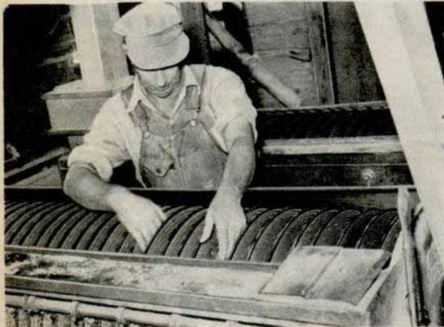
In Japanese rice mill, husked rice pours from machine into rope bag. Below, steel disks separate kernel from rough outer husk in modern machine used in rice milling operations in Louisiana Farm Security Administration photo
