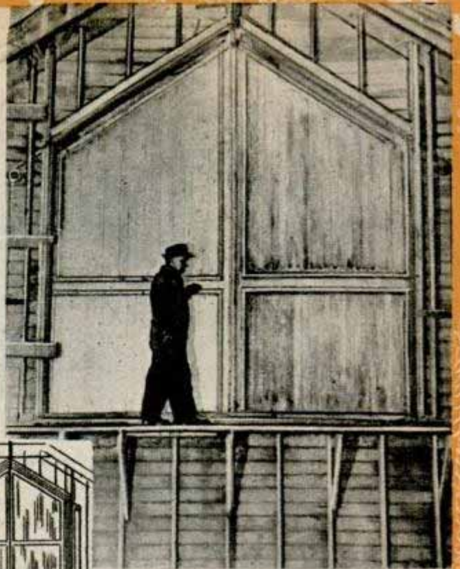
If the doors should open suddenly this farmer would disappear. The walkway should be three feet beneath door level with a handrail
