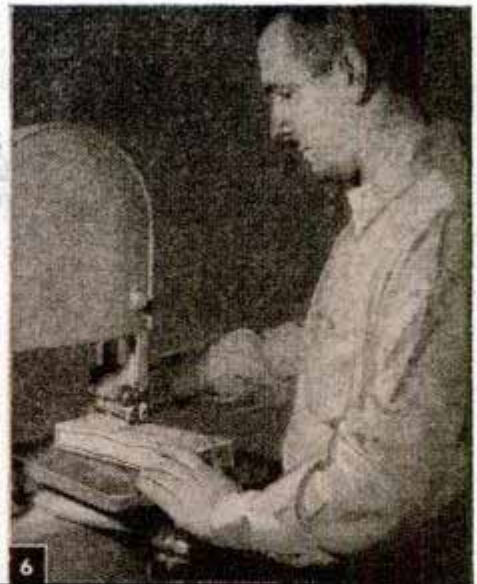
Nearly all parts of figures can be bandsawed to the rough shape
