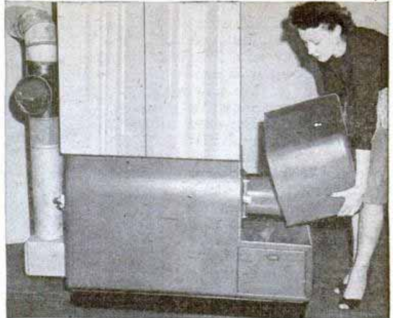
Circulating fan in oil-fired furnace changes air six times per hour. Dust and dirt are kept out by filter
