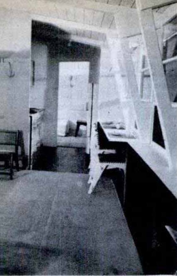
Right, with one of the end walls and part of an interior partition in place, the builder assembles the roof trusses
