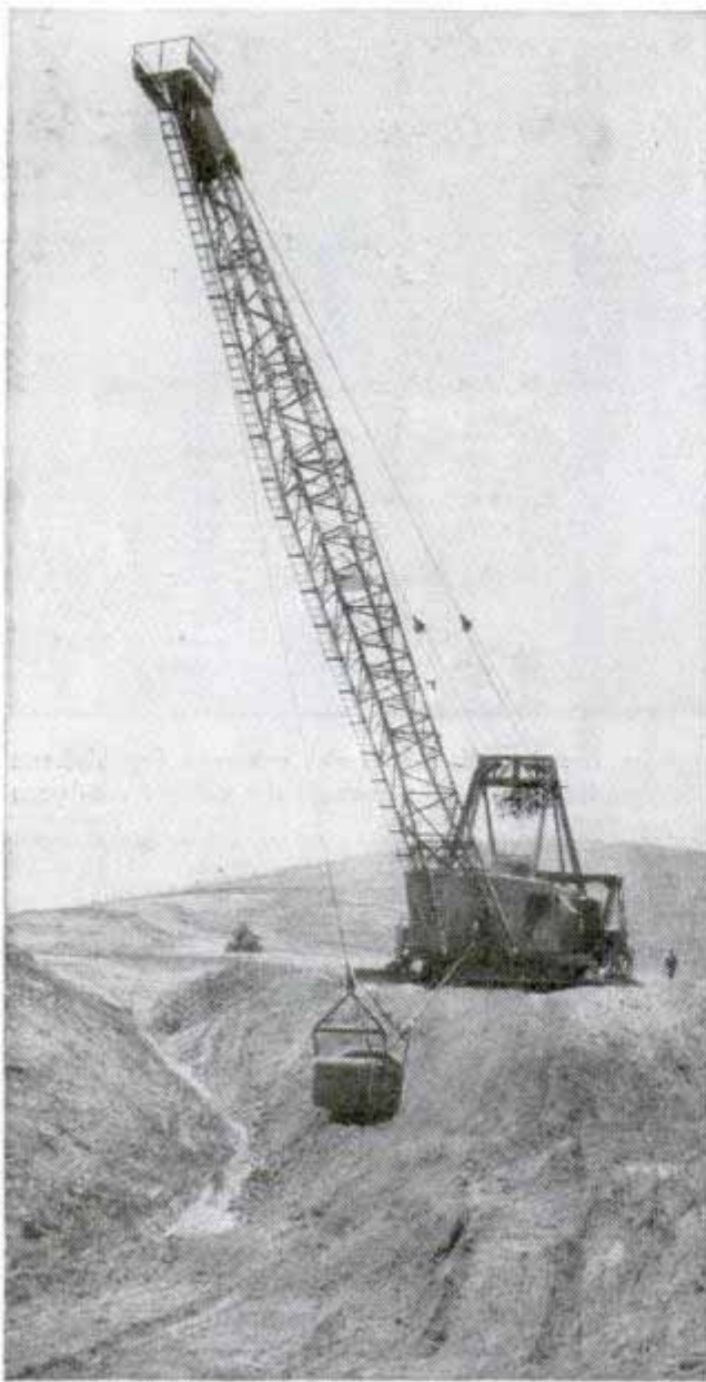
Dragline hauls five cubic yards of earth in one scoop. Below, side view of mechanical ditch digger
