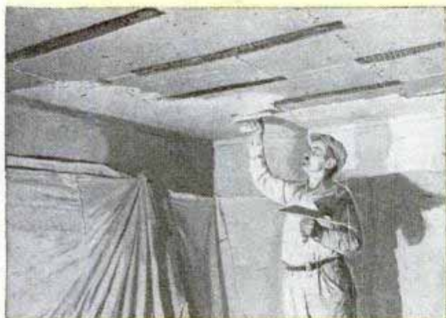
Strips of metal lath are used over joints, staggering them as shown. First coat is troweled about 1/4 in. thick and roughened with a whiskbroom while soft to provide a "key" for second coat
