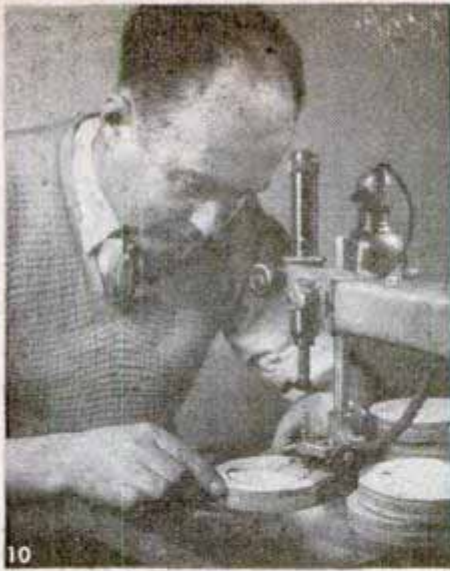
And finally, the center is sawed out of the disk leaving two separate parts, a ring and a matching inner disk
