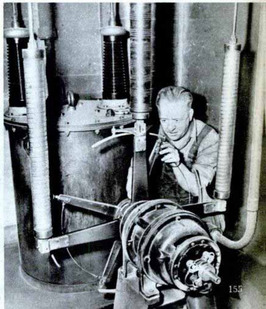
Checking the weight of a 400-ounce gold certificate bar worth $14,000. Below, cleaning the electrodes of the power unit that operates the mint's electrostatic air cleaners
