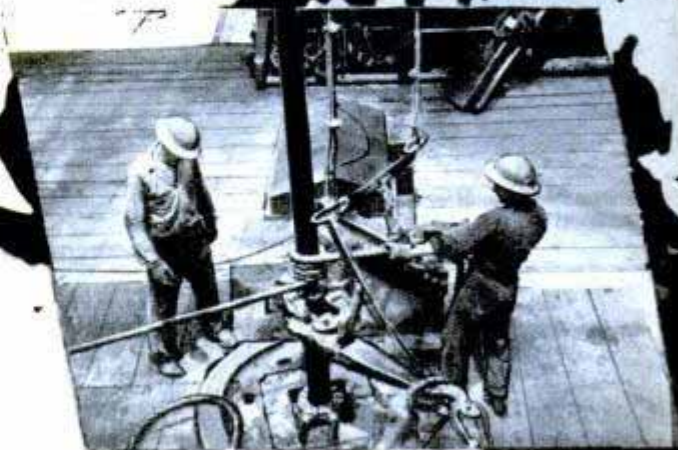
Tightening the drill pipe on a derrick boat working at Lake Salvador in Louisiana
