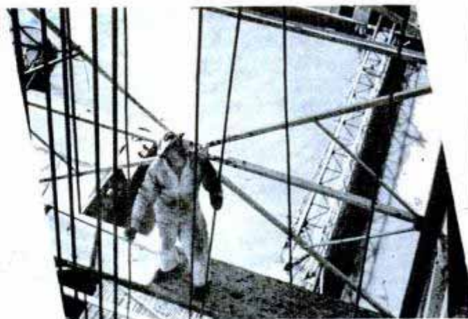
Derrickman perches on a board as he rides downward from his platform to adjust pipe
