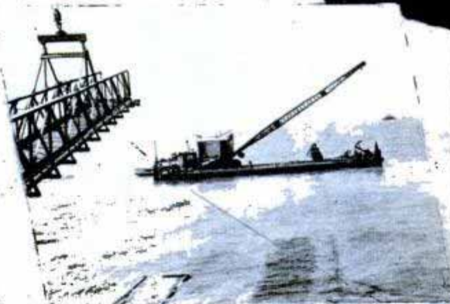
Catwalk towers above an oil well chute, ready to connect derrick and boiler barges
