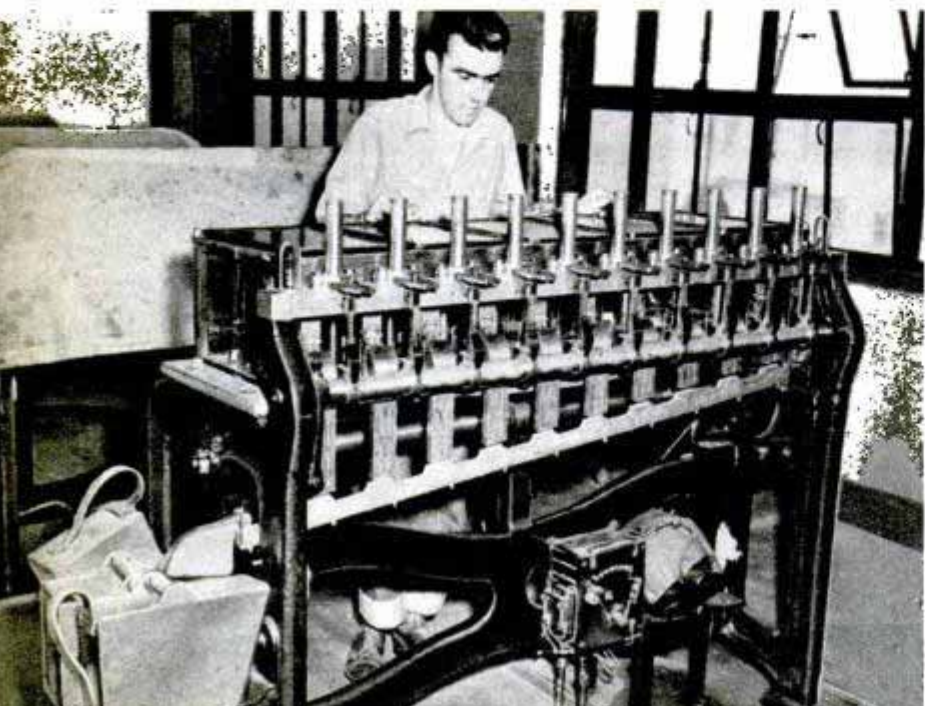
Copper blanks soon to be pennies get "squeezed" in device above to give them thick edges, vital for long wear. Weighing machine, below, checks coins to be sure they are within legal tolerance
