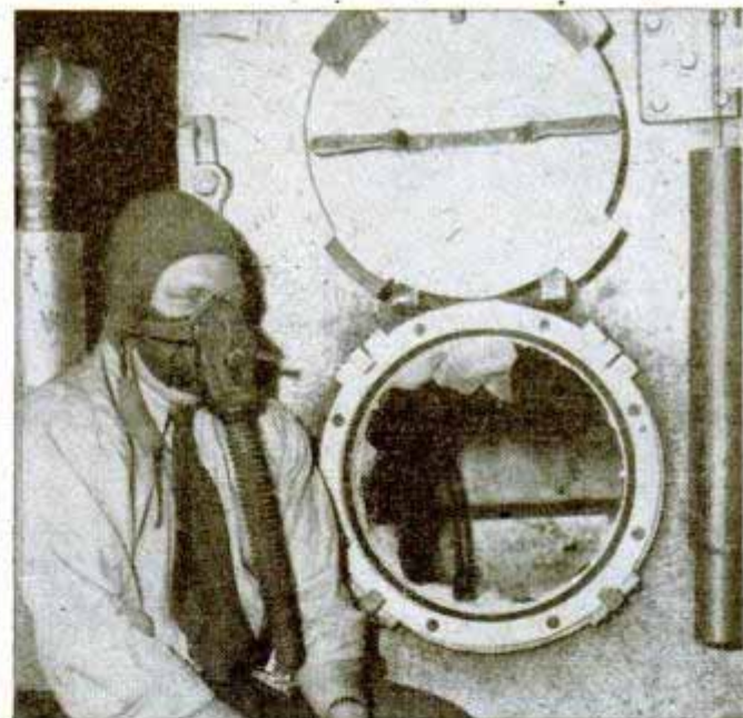
Dr. Fred Hitchcock of Ohio State University locks the heavy steel door of the decompression tank for a test. With a loud report, the panel is blown out and pressure in the two chambers rapidly becomes equalized.
