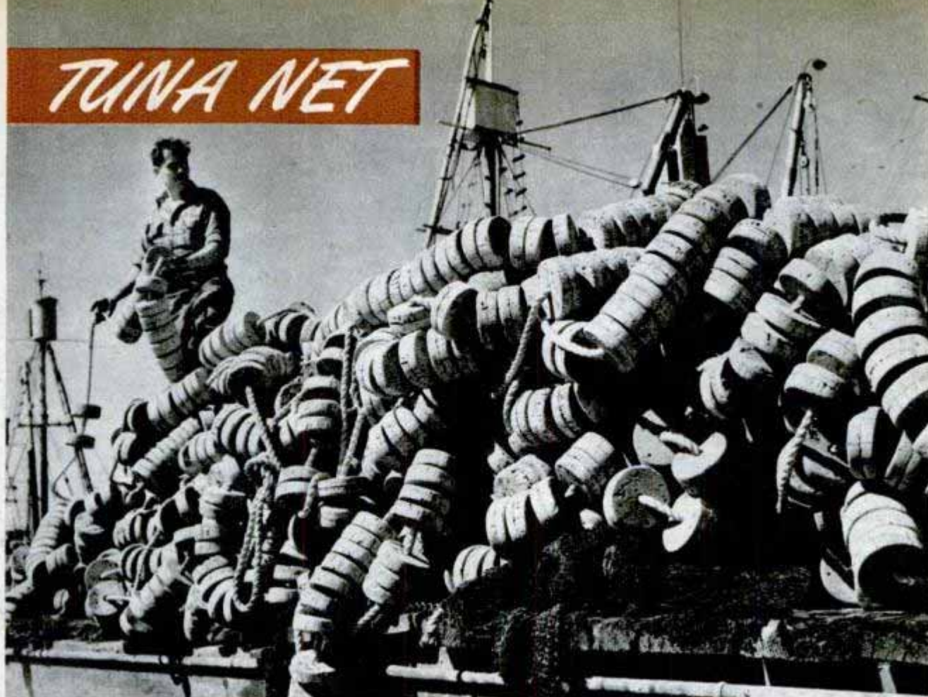
Cork beads for a tuna man. In groups of three, 10,000 of them are tied to the cork line to keep afloat the $15,000 circle of tarred net that pulls in tasty tuna for your table. A crew of 11 men handles the net
