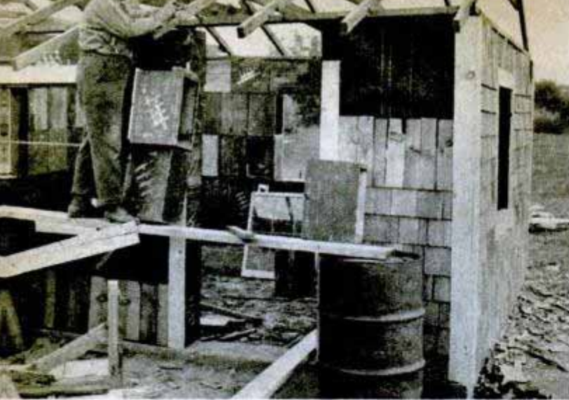
SURPLUS AMMUNITION CASES provided part of the lumber for Carl Hendrickson of St. Paul, Minn., to build a house. When this picture was made, the boxes still bore Army and Navy ammunition labels on the side
