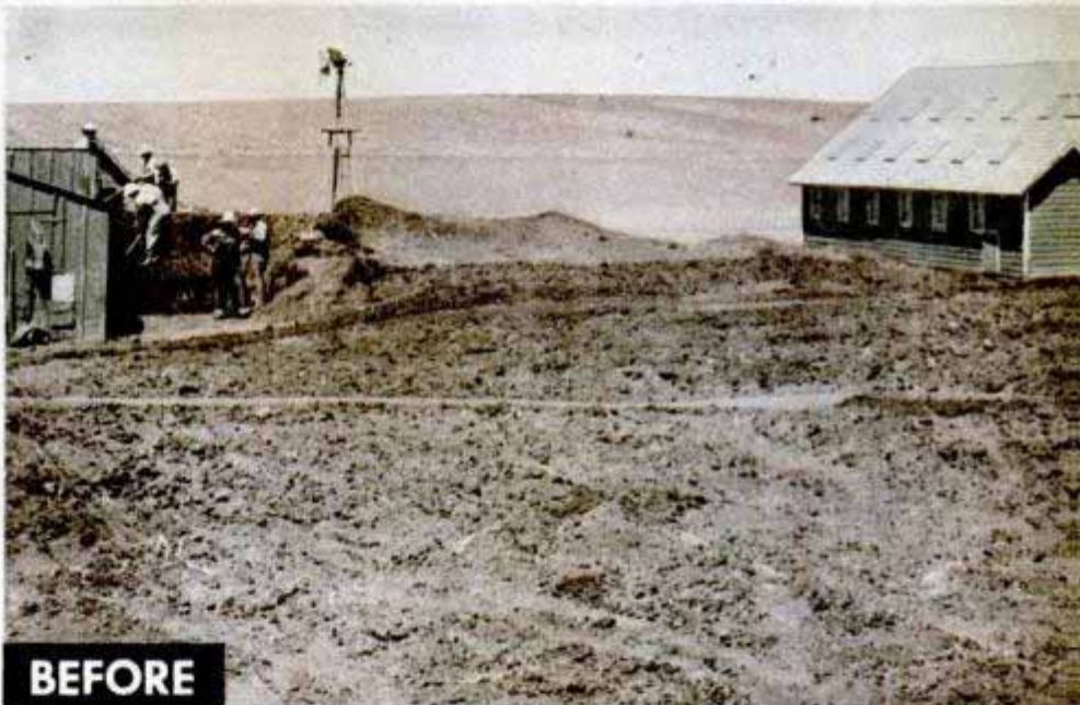
↑ Farm teamwork clears the "blow" dirt away from half-buried buildings
