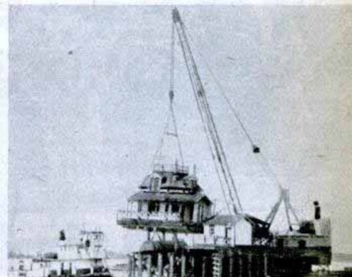
ABANDONED LIGHTHOUSE was moved from the juncture of the Columbia and Willamette Rivers to Burlington, Oregon, to solve the housing problem of an enterprising couple. A huge crane mounted on a barge lifted the lonesome 50-year-old structure from its heavy pilings and carried it to its new site on the shore
