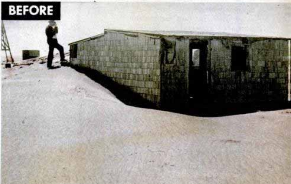
↓ Drifting sand has reached almost to the roof of this little farm home; fences have been torn down to permit the suffocating sand to blow away
