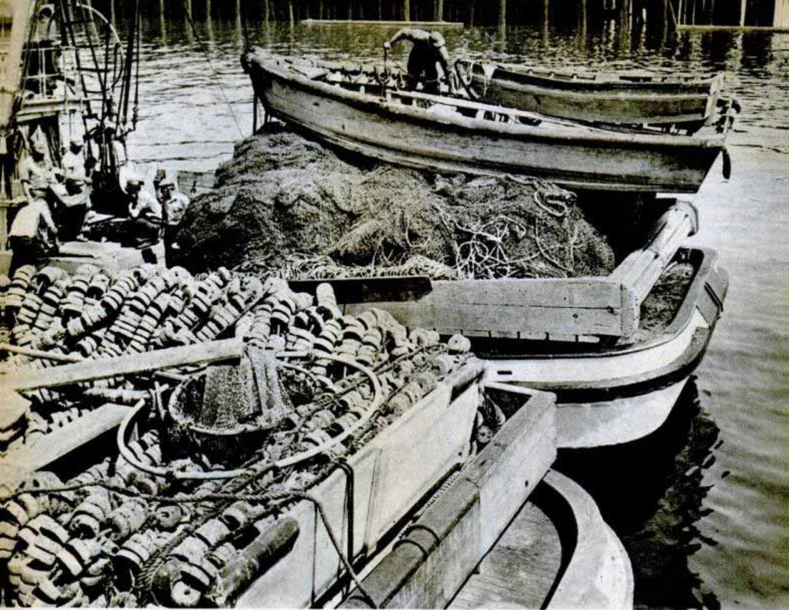
A power-driven turntable at the stern hauls in the eight-ton tuna net when everything is ready. The big skiff, which marks the free end of the seine, and the utility boat, top, are loaded aboard; then the purse seiner (below) heads for the open sea and—with luck—good fishing
