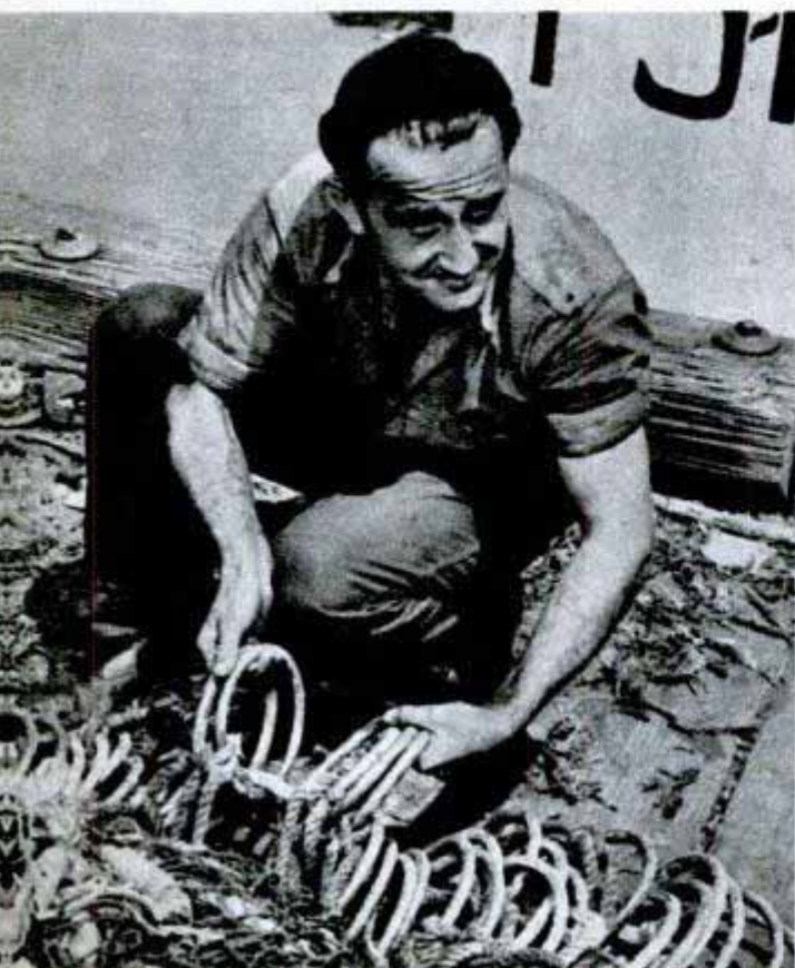
↓ Like old-fashioned moneybag, enormous purse seine has a "drawstring." It's a one-inch rope threaded through steel rings tied to bottom lead line. After several seasons of use, this one must be replaced
