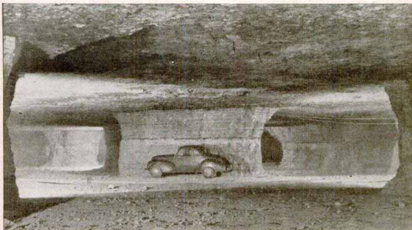
Natural limestone vault near Atchison, Kansas, covers 15,000 acres; holds about 52,000 tons of perishable foods
