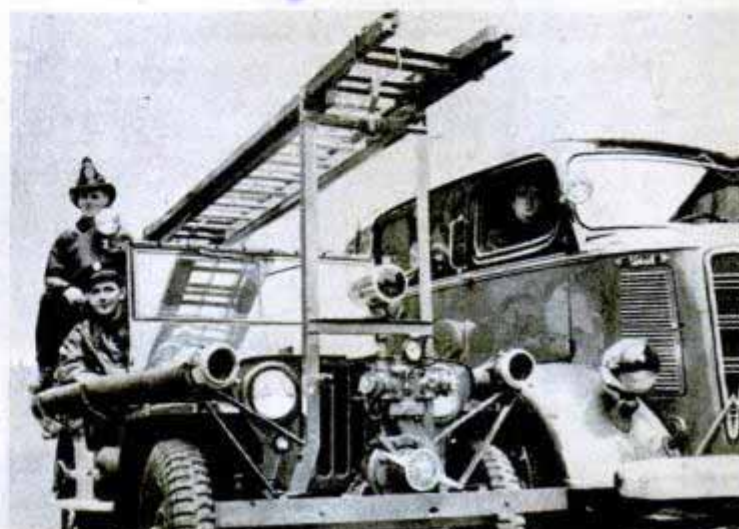
JEEP FIRE ENGINE , a dwarf compared to a regular size machine, is ideal for hurdling ditches and speeding across bumpy fields to combat fires in rural communities. Some industrial plants also use the modified war jeep to scoot through production aisles and hurriedly reach the scene of a fire or explosion. The fire jeep costs $2800
