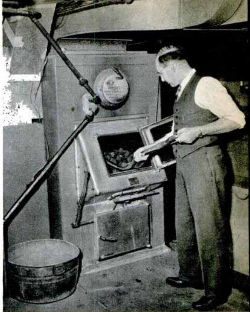
Smokeless furnace, fired by its developer, Prof. Julian R. Fellows of the University of Illinois, directs smoke and gases from new coal through coal already burning. Diagram below shows how the furnace operates
