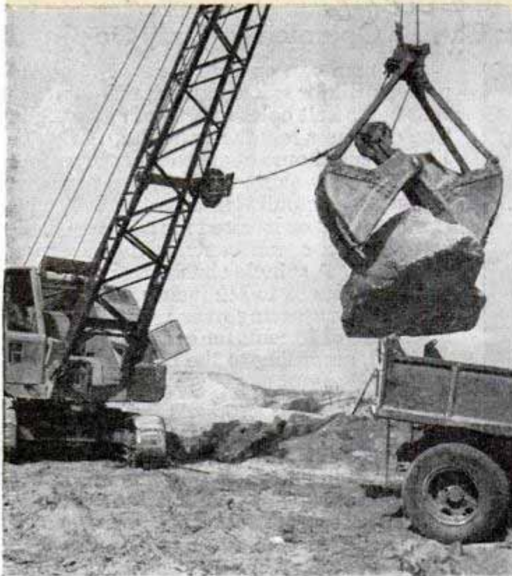
From this pipe line spews forth land-building sand scooped from the mountains of Southern California. Below, giant rock is lifted into place atop dike that is pushing land farther out into Long Beach Harbor
