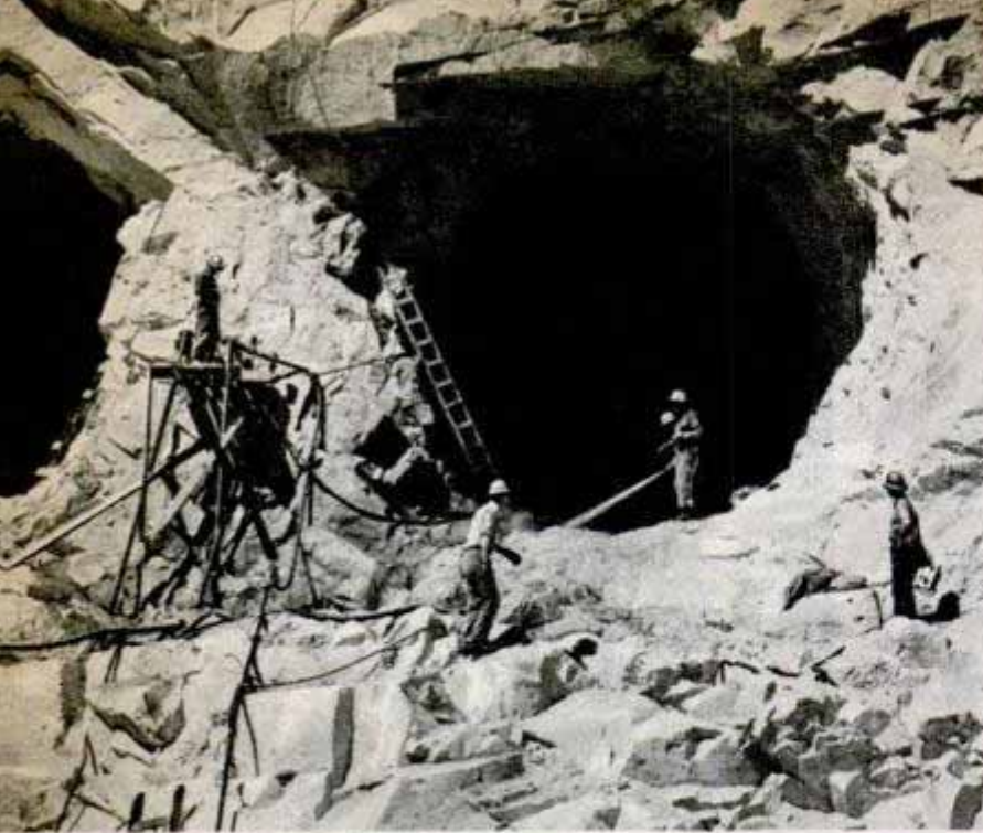
Through 12 huge tunnels, shown under construction above and below, 50 tons of water per second will be lifted 280 feet over canyon walls from the lake to fill the irrigation reservoir
