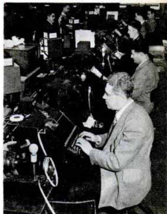
Communications flashed from the American Cable & Radio operations room (right) via transmitter (below) reach Europe in 10 minutes. Transmitting and receiving equipment handles 38 overseas circuits
