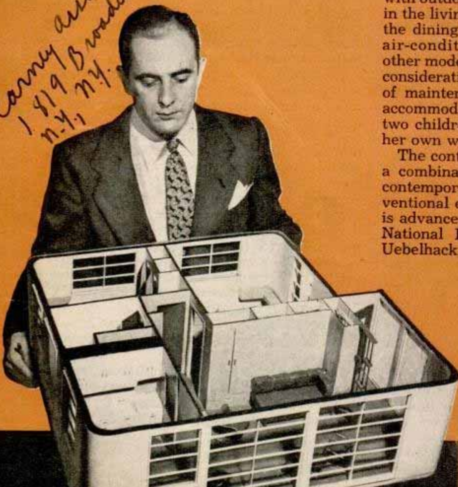
Model of "featherweight" plywood prefab made in four sections, each with built-in fixtures including beds
