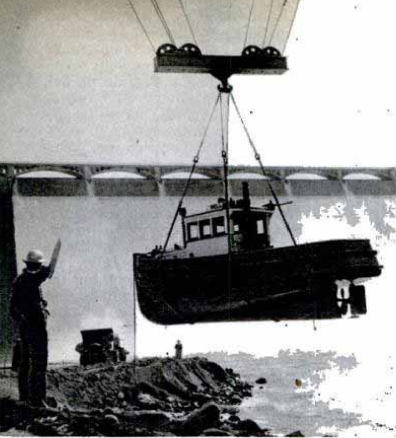
A half mile away, a cableway operator guides the controls which launch a 22-ton Bureau of Reclamation tug, left, in the waters below Grand Coulee Dam. Right, power switchboard through which power is fed to pumps
