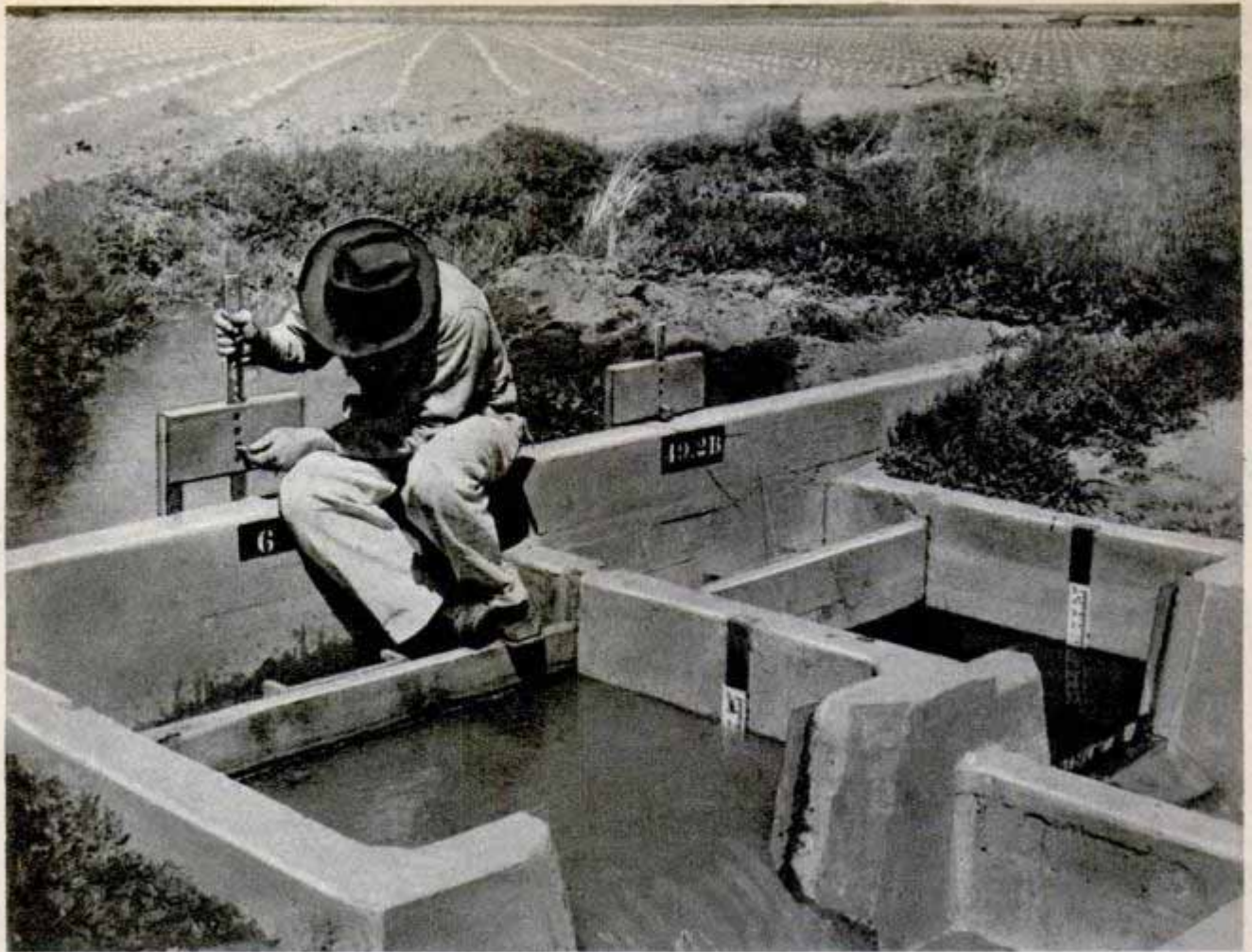
Farmer adjusts the head gate of canal sluice box to control amount of flow of life-giving water to dry fields
