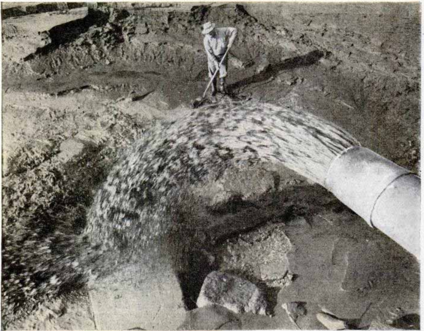
From this pipe line spews forth land-building sand scooped from the mountains of Southern California. Below, giant rock is lifted into place atop dike that is pushing land farther out into Long Beach Harbor
