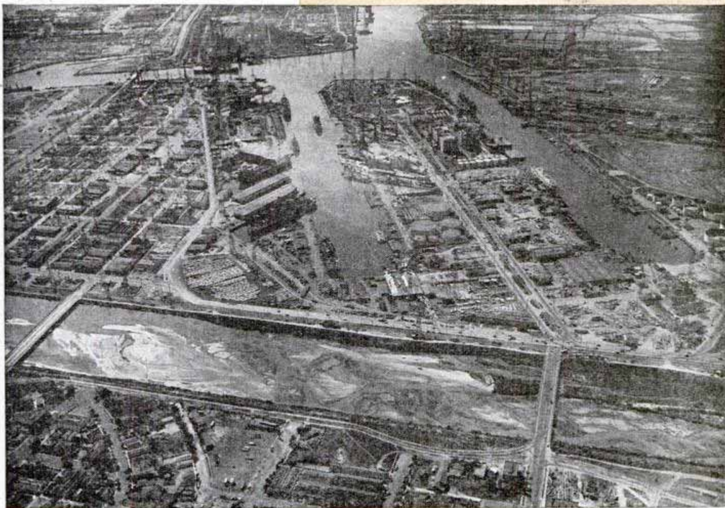
Ships unload at a completed pier in the harbor. The land was built of silt from the Los Angeles River. Below, sandy channel of the river (foreground) sweeps past the harbor
