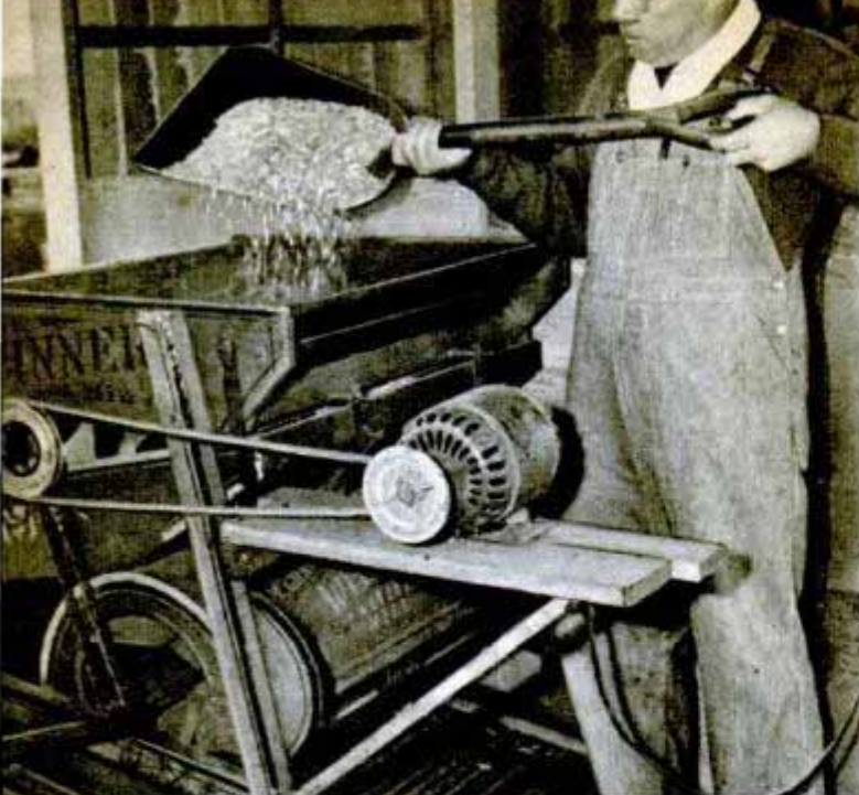
Fanning mill (at left) is driven by a small portable electric motor. Right, electric screens instantly kill flies
