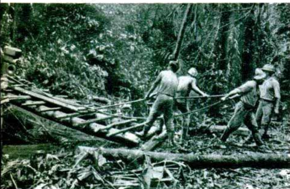
Below, building the $20,000,000 Panama fuel pipe line with a daily capacity of 265,000 barrels of fuel oil—a wartime project U. S. Navy photo
