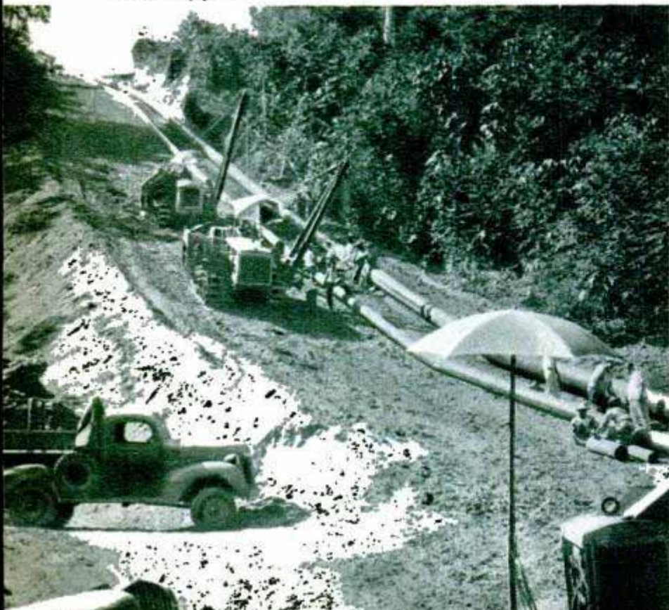
Below, building the $20,000,000 Panama fuel pipe line with a daily capacity of 265,000 barrels of fuel oil—a wartime project U. S. Navy photo
