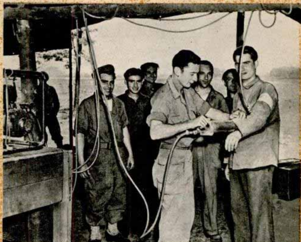
Delousing machine (left) developed by the Quartermaster Corps dusts 600 persons per hour with DDT powder. Right, an American soldier delouses former slave laborers and political prisoners freed from a German camp
