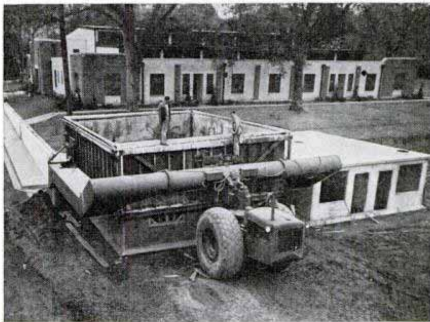
At the site (above) the home is set down and the house layer prepares to move away for more concrete to build another structure. Below, Tournalayer containing another new house is on way to site
