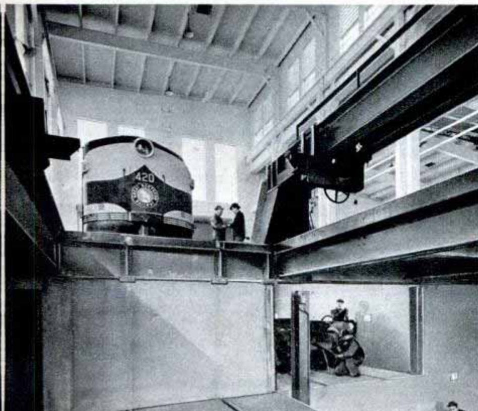
Great Northern's new Diesel service shop at Havre, Mont., has a drop table (lower left) and track pit 205 feet long (right). Design was adapted from Italian railway
