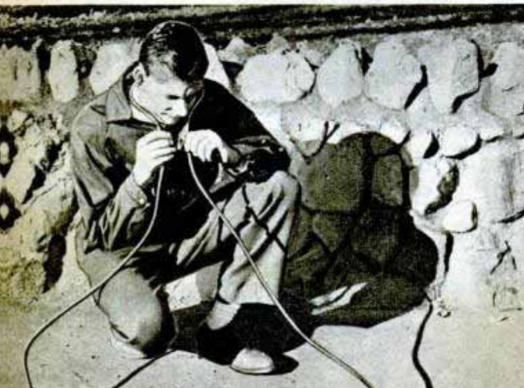
PLUMBER'S "STETHOSCOPE" locates underground leaks in water pipes and leaks in steam pipes behind walls and under floors. Air chambers amplify sound
