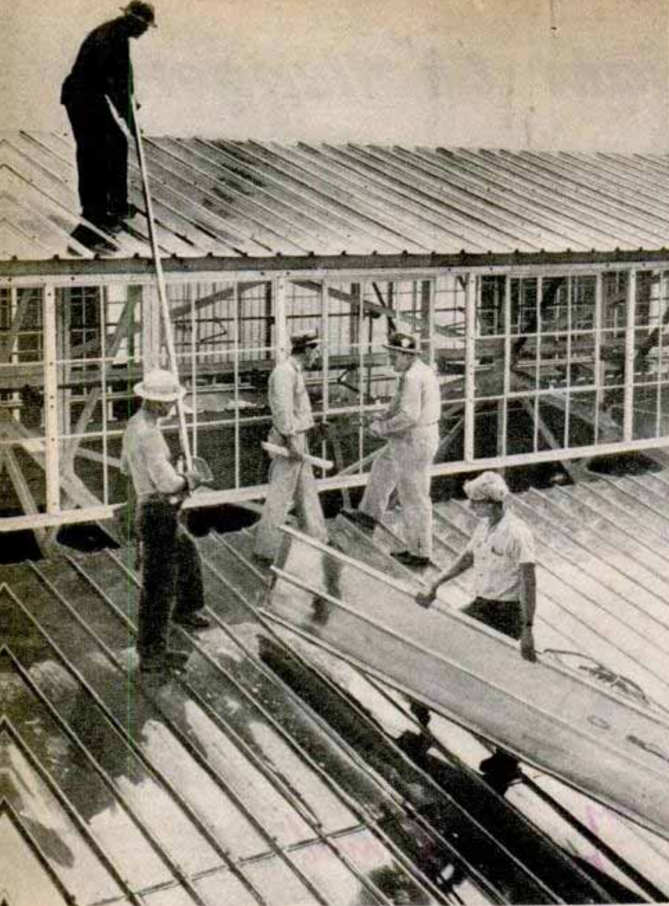
Above, aluminum roofing requires no paint, resists corrosion. Two of the workers wear aluminum helmets. Below, stacks of lightweight utensils for postwar kitchens
