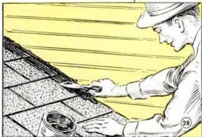
Joints between siding and roofs should be resealed with paste roofing compound before painting, or better, flashed to the siding if this was not done on the original work
