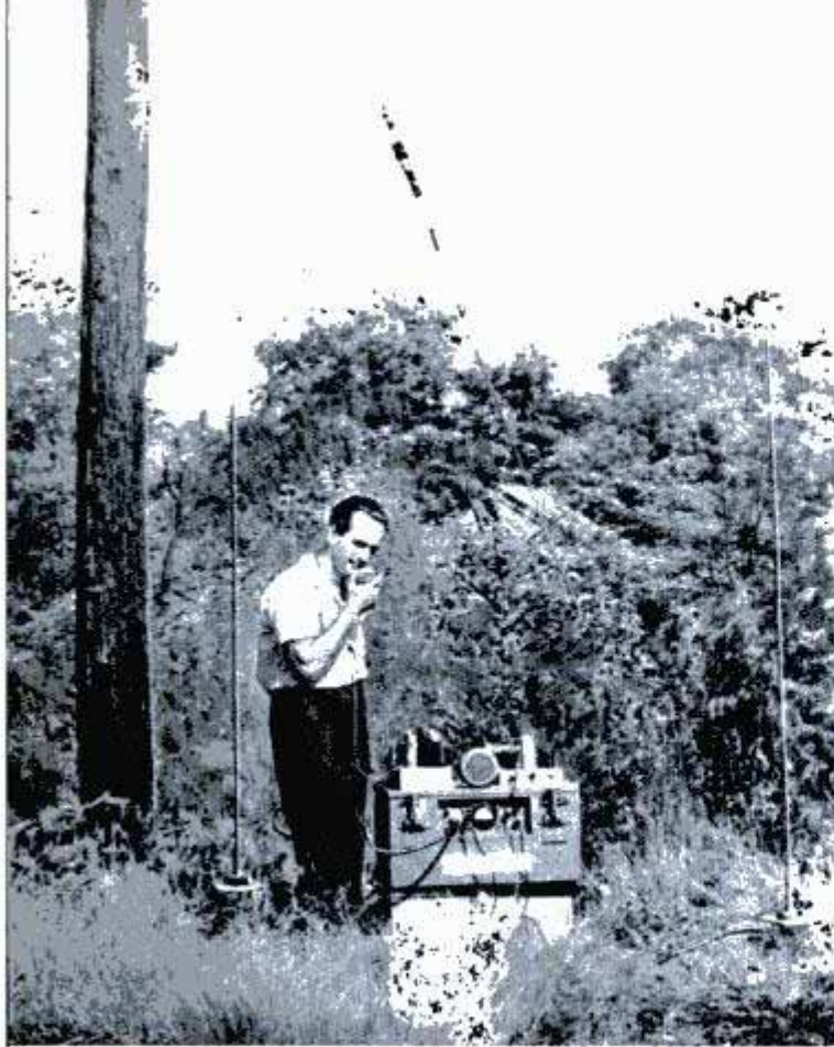
When lines are down, radio "patching" solves communication problem. Left, operator of portable transmitter-receiver spans gap in telephone line by putting signals on the air. At other end of gap similar unit receives message which is put back on wire. Right, testing walkie-talkie for use on handcar to keep repairmen informed of approaching trains. Below, cutaway drawing shows layout of Rock Island's rolling radio laboratory
