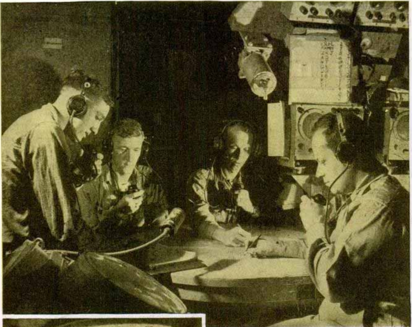
Four observers maintaining a surface plot in CIC. Left, raid plotter notes approach of a bogey, carefully recording time to the left of the track path. The small "o"s mark the course of a friendly plane
