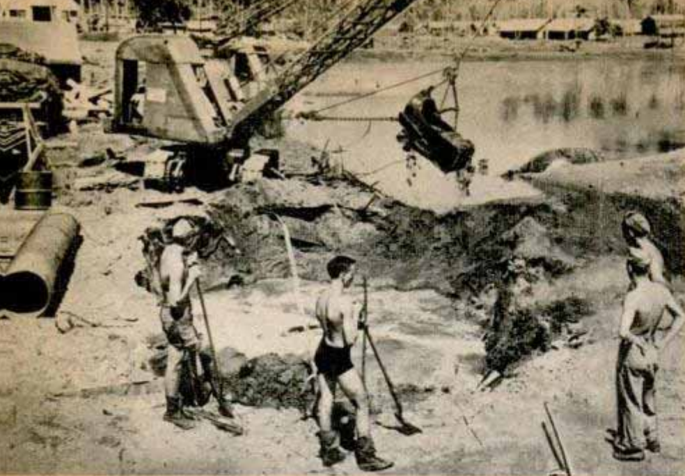
Digging flume to drain malarial lagoon into ocean. Nearby is camp
