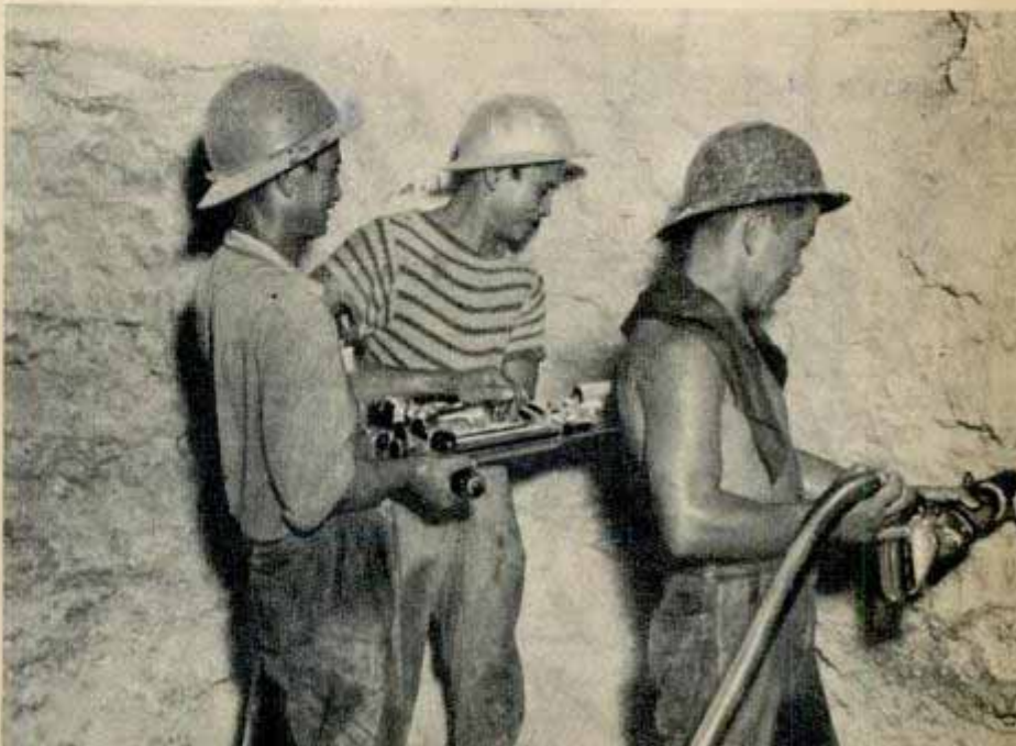
Giant rainbarrels catch water during tropic storms. Below right, tunnel workers drill holes for dynamite
