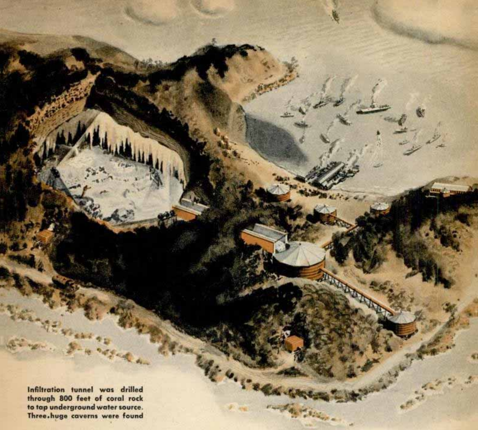
Giant rainbarrels catch water during tropic storms. Below right, tunnel workers drill holes for dynamite
