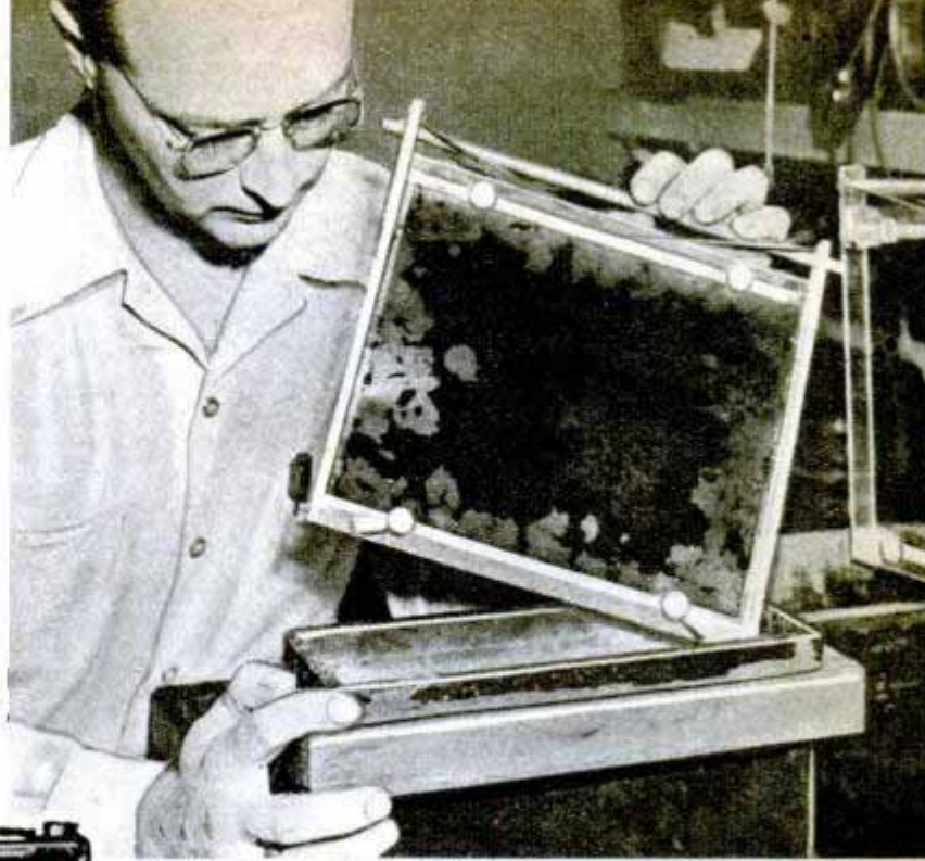
Courtesy Grover Photo Products Plastic hanger with locking grips holds film during processing. Left, X-ray base used as camera stand
