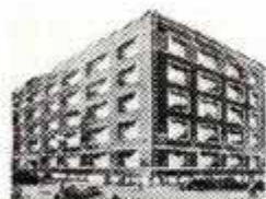
This modern fireproof building is occupied entirely by the Coyne Electrical School.
