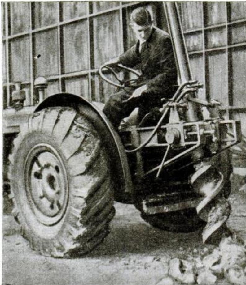
Auger attached to tractor gearbox digs postholes for Aussies
