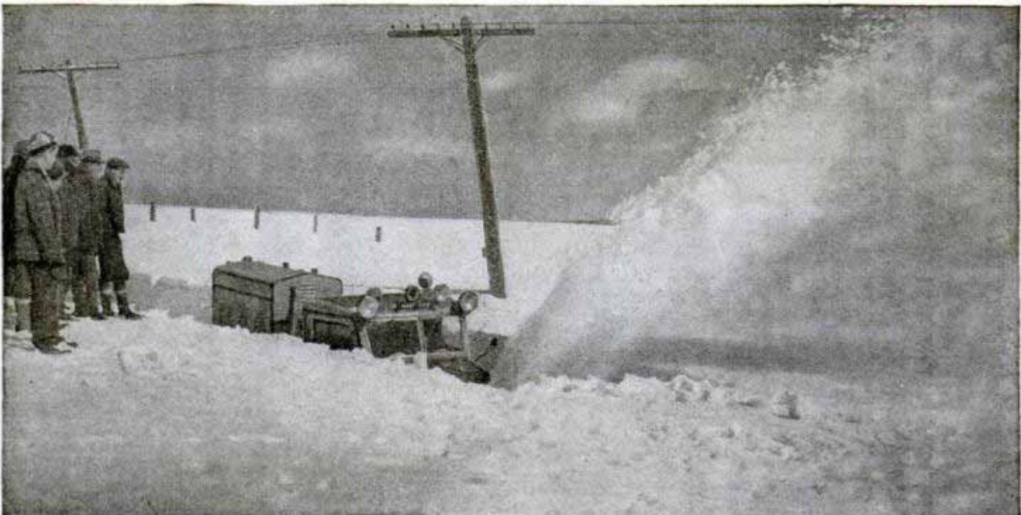
Brother of the rail plow, the highway model eating into a deep drift below can fling a plume of snow 125 feet. Many were built for the Army.
