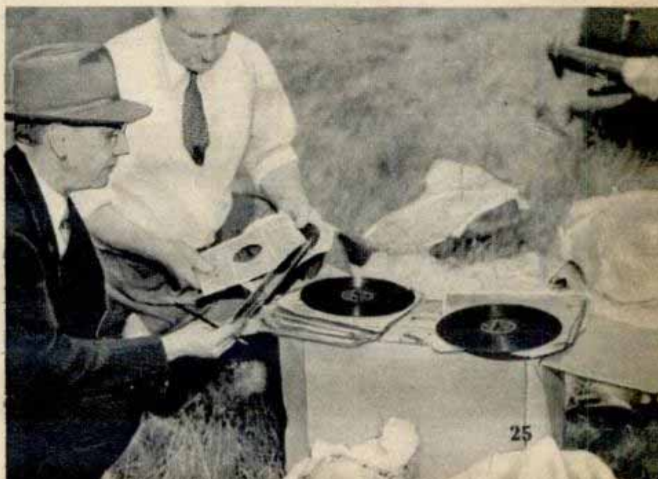
Swinging from special parachute is fiberboard carton containing phonograph records. Below, records landed without scratch
