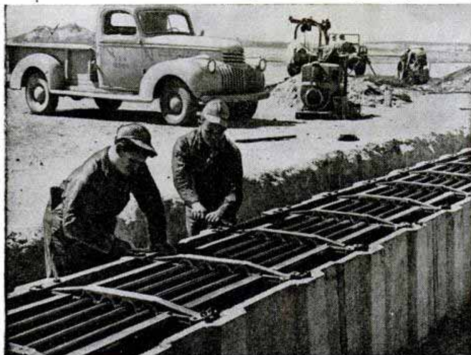
Pipe lines to carry gasoline are installed in trenches like this in FIDO installations. Below, close-up of a six-siren sonic generator which creates a noise heard many miles from Arcata, Calif., scene of the fog tests
