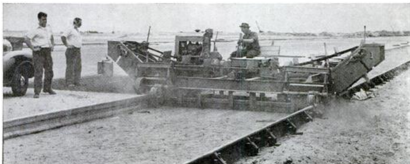
A surveyor lays out the line for 8400 feet of sewer pipe to drain low marshlands. Below, self-propelled subgrader moves ahead of concrete mixer to smooth surfaces for a long runway
