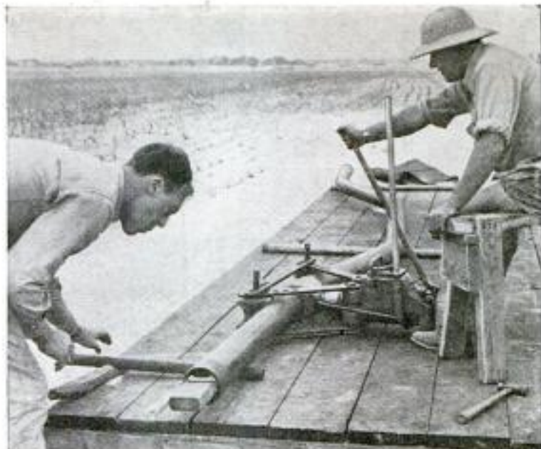
Hydraulic pipe bender that exerts 40-ton pressure twists steel pipe into desired shapes for electrical conduits at the airport
