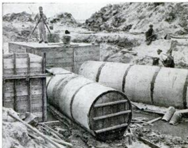
A surveyor lays out the line for 8400 feet of sewer pipe to drain low marshlands. Below, self-propelled subgrader moves ahead of concrete mixer to smooth surfaces for a long runway
