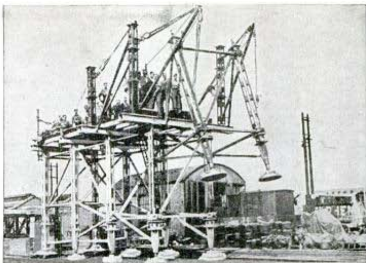
British soldiers test section of unit construction bridge which helped patch the bombed railroads in Europe as Allied troops advanced
