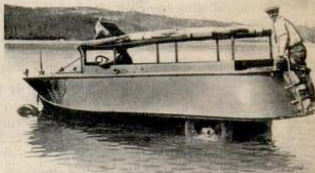
National Geographic photo Sea Turtle takes to the sea during Aleutian expedition. This 21-foot steel craft was the second amphibious car designed by Dr. Jaggard. It was powered by a Ford Mod- el T engine and had twin screw propellers. First used to study volcanic formations, Sea Turtle fathered wartime DUKW shown below grinding ashore with full load U. S. Marine Corps photo
