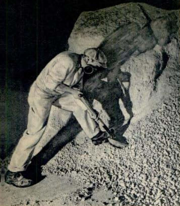
Clay is mixed with feldspar and flint, water is added. Electro-magnetic slip trough takes iron bits from mix
