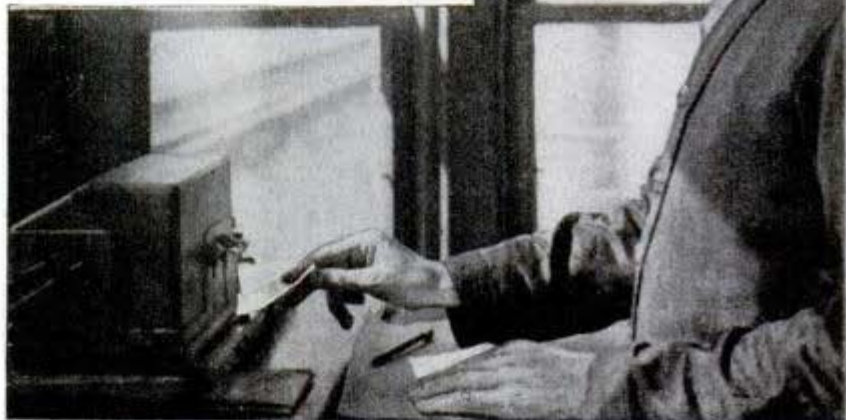
Way bills are inserted in machine which automatically records weight of cars in scale house near big classification yard
