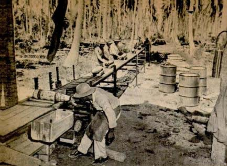
Chain belt carries rusted 155-mm. shells which are being repaired
