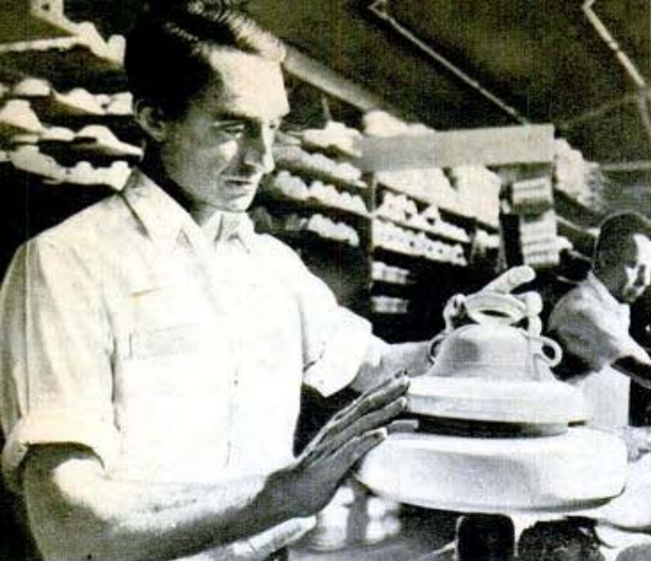
Modern potter's wheel, jiggering machine makes simple shapes. Green ware is fired in bisque kiln, above right
