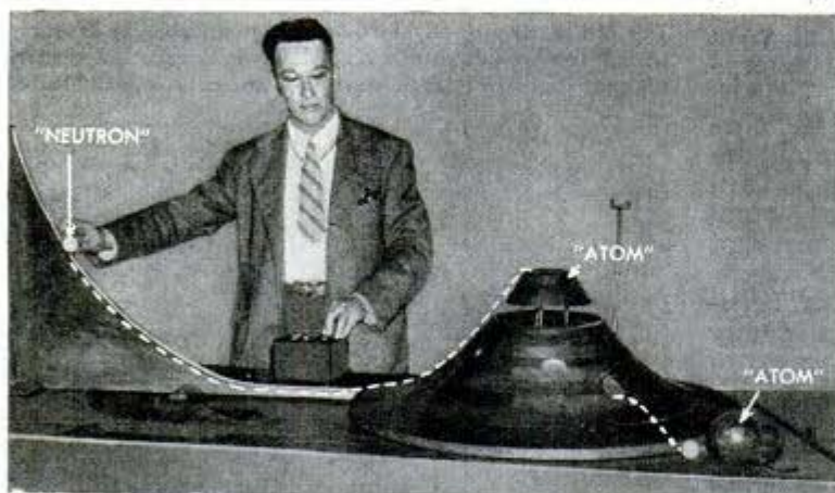
Pittsburgh Press photo Demonstrator at atomic power show in Pittsburgh Buhl Planetarium shows how slow-moving neutron enters nucleus of U-235 atom, splitting it to release second neutron which strikes another atom. Below, radium neutrons hit U-235 embedded in paraffin and screen records splitting atom
