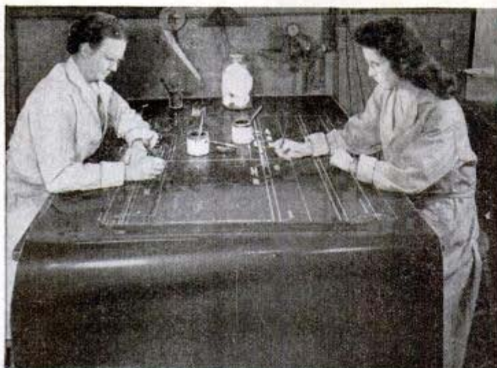
Retouchers at work on big negative from giant camera used in making blueprints. Negatives can be as large as 4 by 8 feet
