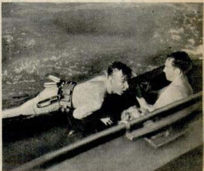
His explosives planted under water, a diver comes up
