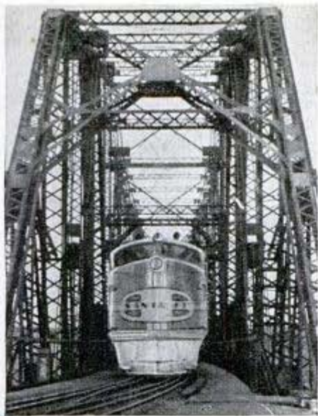
Diesel locomotive slows pace across old cantilever bridge which was a bottleneck until replaced with modern span. Below, new double-track bridge at Needles, Calif. Santa Fe photo
