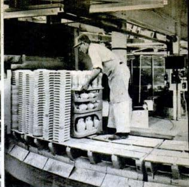
Modern potter's wheel, jiggering machine makes simple shapes. Green ware is fired in bisque kiln, above right
