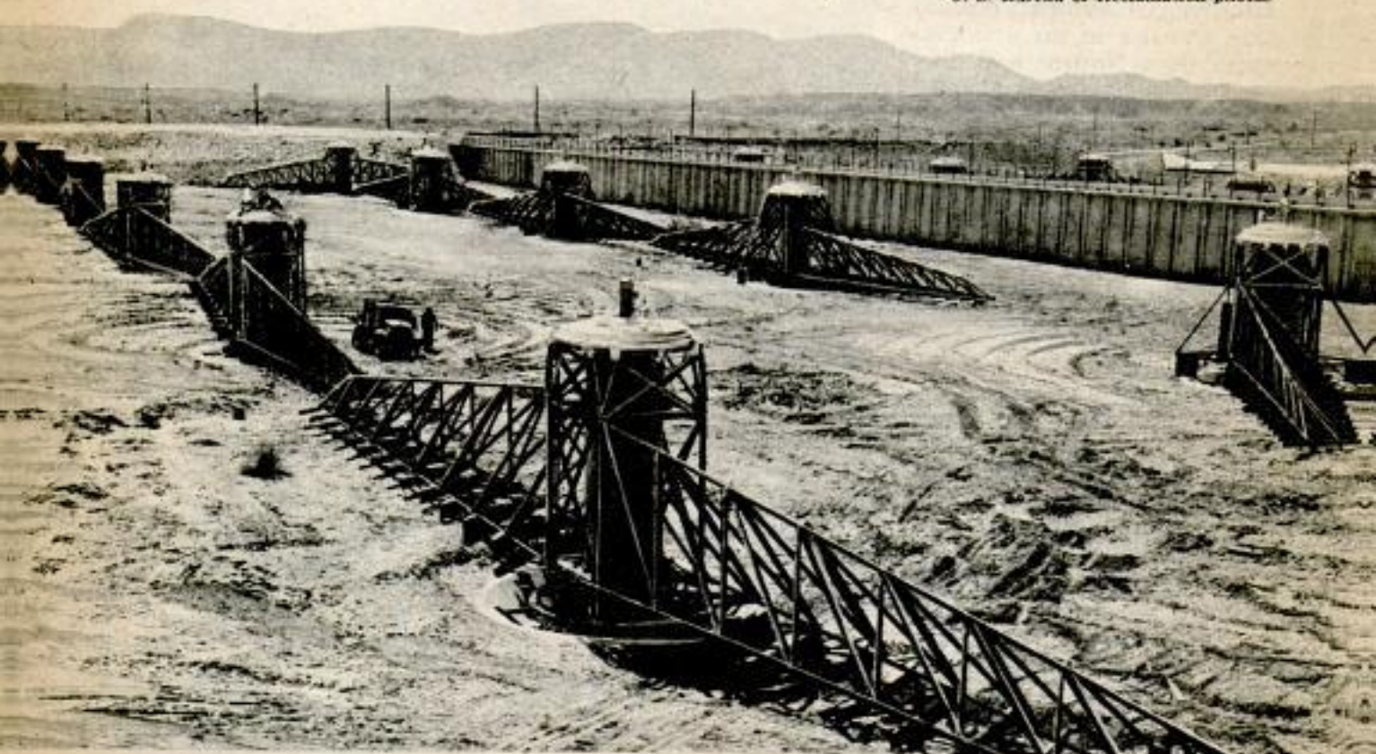
Dorr clarifier units act as huge brooms in desilting basin, keep silt from flowing into All-American Canal
