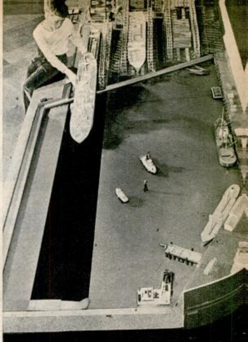
MINIATURE SHIPYARD an exhibit at the Los Angeles County Museum contains models showing various stages in the complex construction of cargo ships, from the laying of the keel to launching. Here is a replica of section of Consolidated Steel Corporation Yards with model of 10,000-ton C-1 cargo and passenger vessel about to leave ways to enter basin
