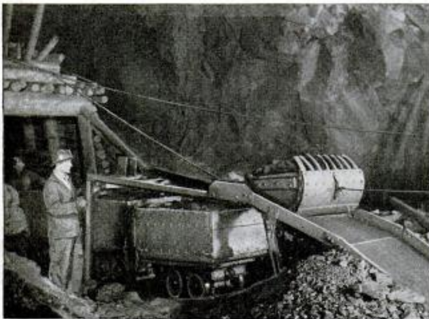
Map shows location of famed Mesabi and other ranges which provide U. S. industry with fabulous amounts of iron ore. Below, underground mine in which ore is being loaded by electric scraper hoist. Note timbered entry
