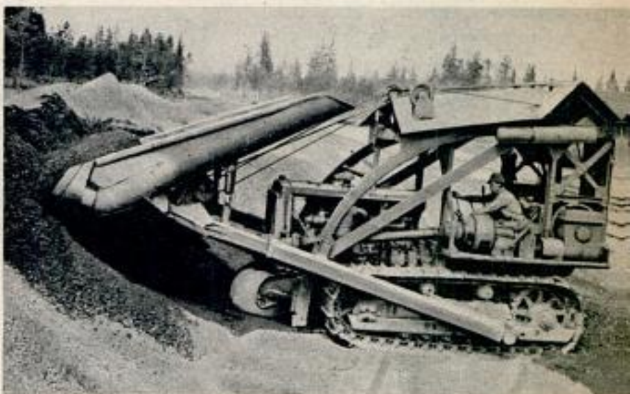
"Cat" with special loader above is used for loading ballast into cars. Portable phone below warns workers trains are due
