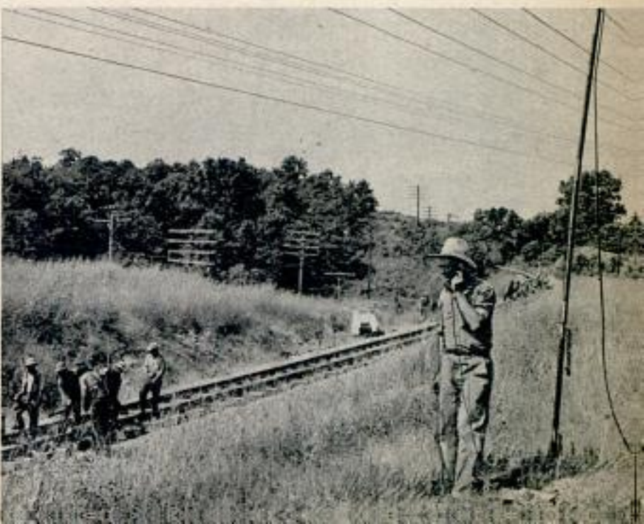
"Cat" with special loader above is used for loading ballast into cars. Portable phone below warns workers trains are due
