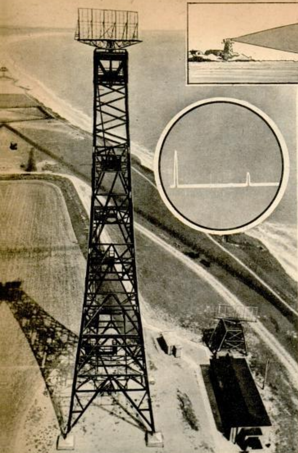
Radar station on British coast has 185-foot tower. Circle inset shows how "pips" appear on range scope. Below, scanning screen for airport and indicator to warn pilot of other craft Civil Aeronautics Administration diagrams
