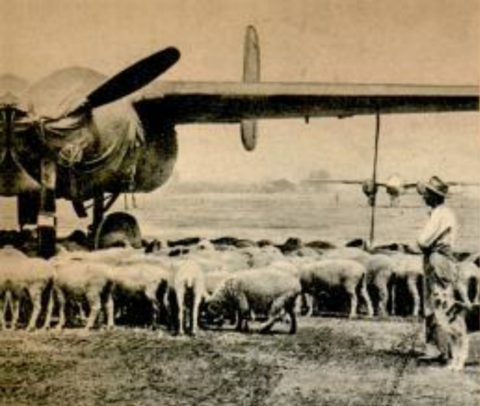
SHEEP CUT GRASS between the steel mat runways at San Bernardino, Calif., field of the Air Technical Service Command. Mowers couldn't be used over mats and grass was fire hazard until 400 sheep arrived
