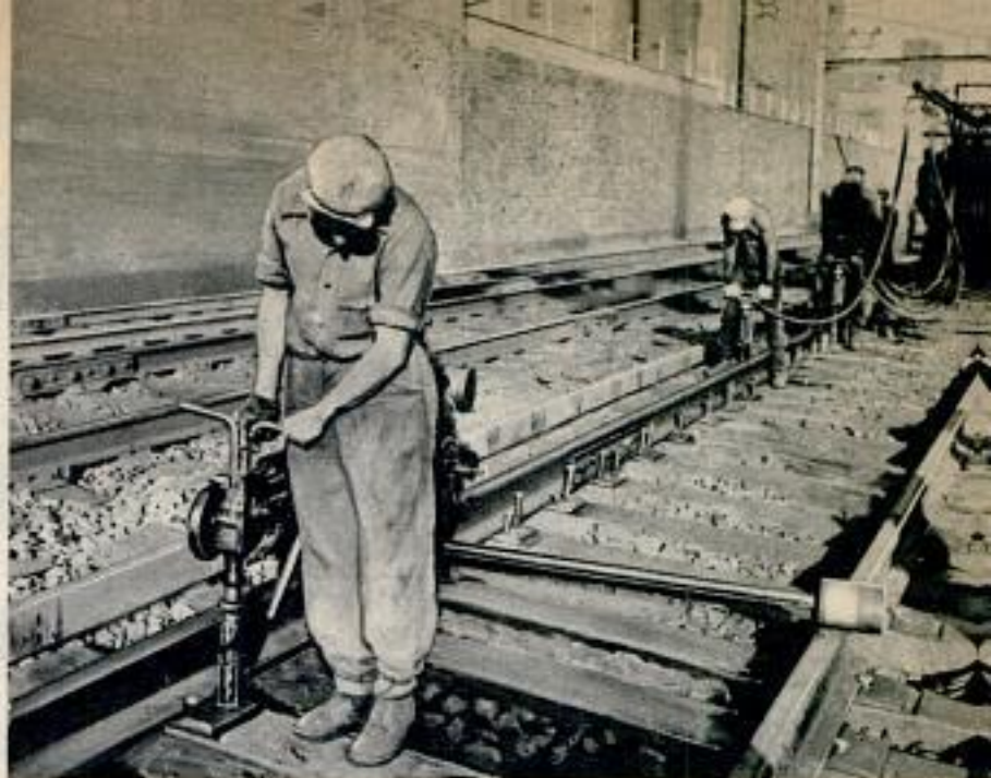
Tie borer in foreground works in team with spike drivers, rear
