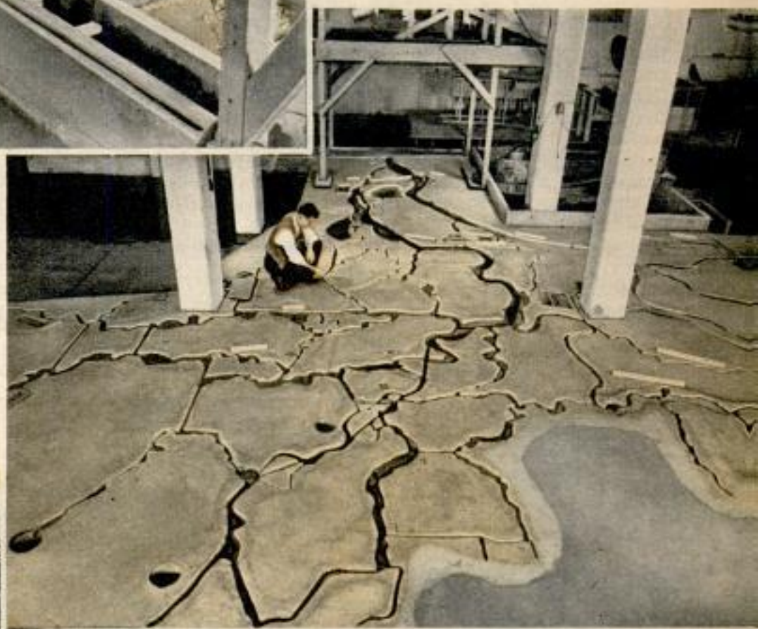
Saw-toothed wheel above in tide machine forms profile of tides in San Joaquin Delta and enabled engineers to learn if fresh water could be transferred across delta model at right. Wheel controls lifting and lowering of sandfilled box in trough of water, simulating tides. Below, 8000-ft. belt conveyor for earth-fill dam
