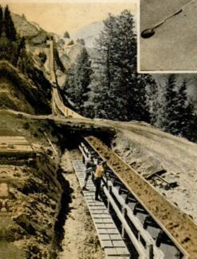
Saw-toothed wheel above in tide machine forms profile of tides in San Joaquin Delta and enabled engineers to learn if fresh water could be transferred across delta model at right. Wheel controls lifting and lowering of sandfilled box in trough of water, simulating tides. Below, 8000-ft. belt conveyor for earth-fill dam
