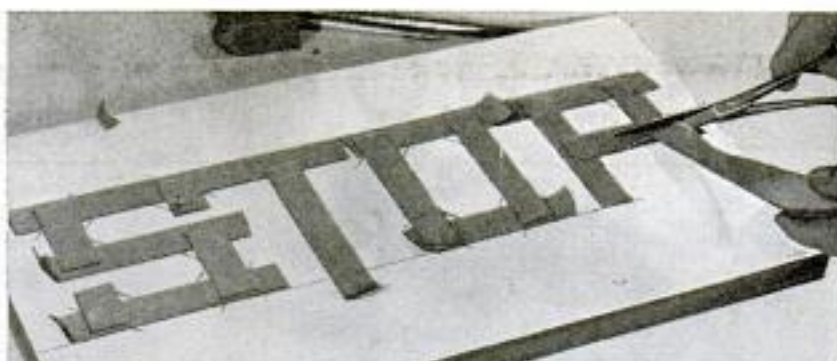
⑧ APPLY TAPE OVER SKETCH, OVERLAPPING ALL CORNERS
