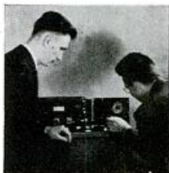
The RCA Radio Altimeter assures that the last mountains have been passed before letting down to the airport in the valley below.
