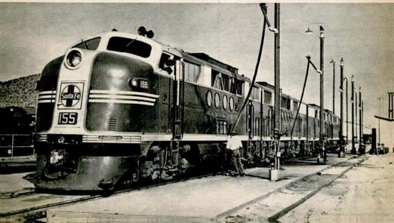
A four-unit freighter spends eight minutes at the fuel racks filling its 5000-gallon tanks with Diesel oil
