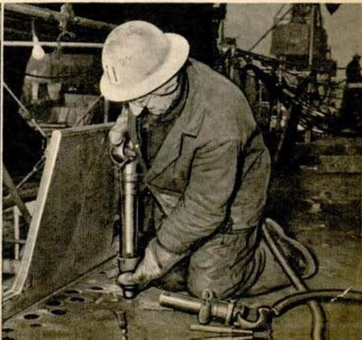
Below at left, workmen building wood pattern for steel gear which will be made for fighting ship. Right, rivet is driven home in deck; it is one of hundreds of thousands of many sizes used in ship building
