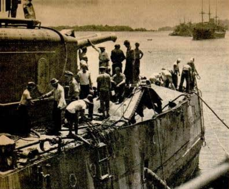
Repair job for navy yard—stern of cruiser Marblehead caught direct bomb hit in Battle of Java Sea. Note bulging afterdeck
