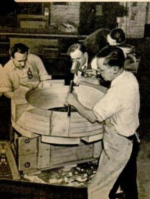
Below at left, workmen building wood pattern for steel gear which will be made for fighting ship. Right, rivet is driven home in deck; it is one of hundreds of thousands of many sizes used in ship building
