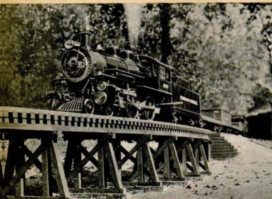
Smoke pours from stack and steam pops safety valves as live steam model pounds over wooden trestle of miniature railroad system. Below, left to right, English type engine, scale model caboose and an American live steamer. Track gauge of the system is 4\frac{3}{4} inches
