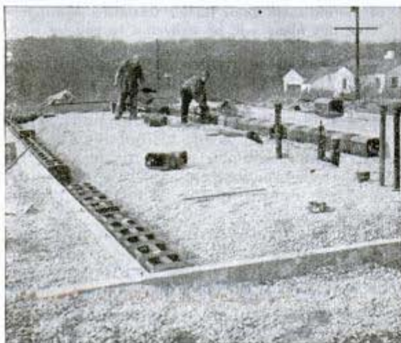
First construction stages, below. Warm air from heat lines, left, is forced through tile floor ducts, right
