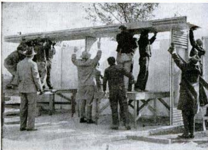
Raising a roof panel of prefabricated model home
