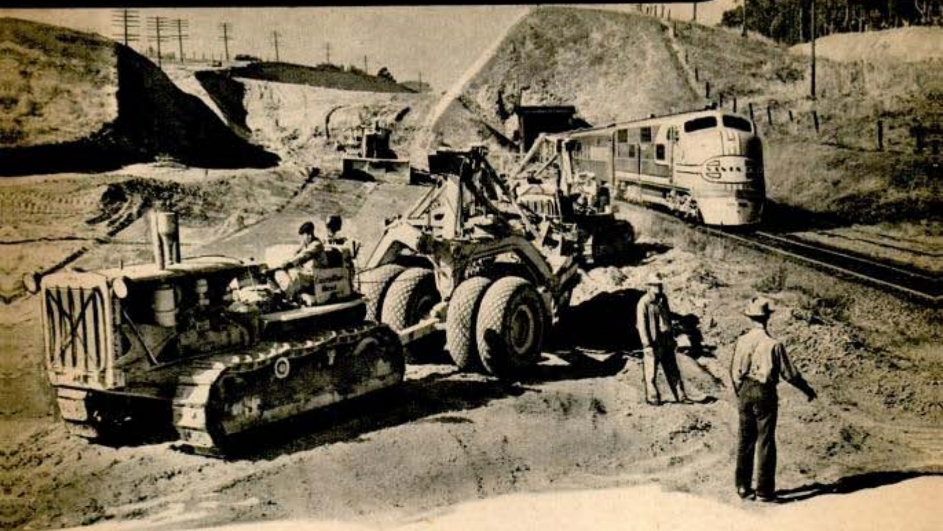
Caterpillar Tractor Co. photo Diesel power moves an 80-foot "mountain" to eliminate railroad tunnel. Below, lowering 6-cylinder Diesel to salvage boat Cooper-Bessemer Corp. photo
