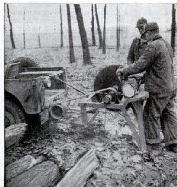
Postwar jeep pulls trailer loads up to 5500 pounds. Below, power takeoff delivers 30 h.p. to buzz saw
