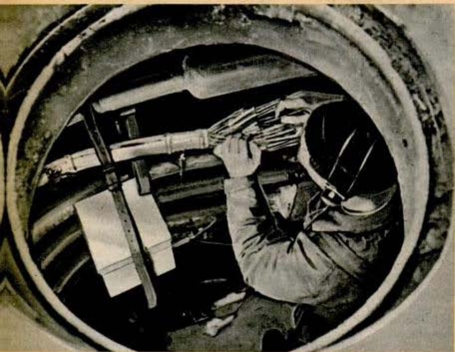
Working in manhole, splicer uses exploring amplifier to locate particular pair of wires by tone testing. Below, service group switchboard for 9th Air Force shows one small part of vast network of military communications 9th Air Force photo
