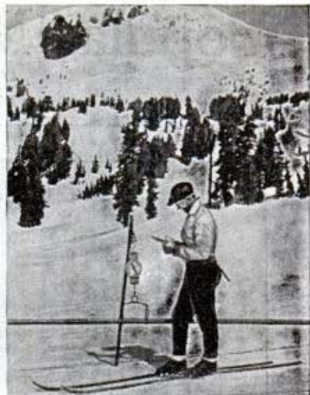
Rangers plan to use four-part Army snow tractor that disassembles for air transport. Right, snow sampling tube to measure water content is suspended from scales. Below, clearing a lane to fight a forest fire.
