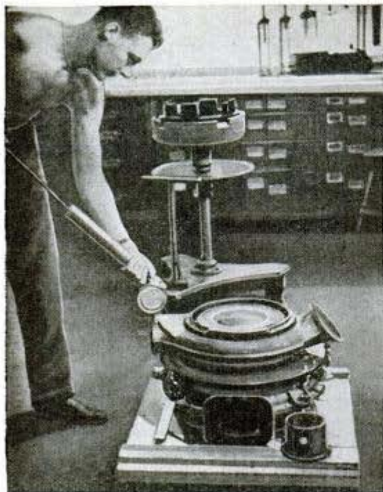
Insect gun acts as oil spray for turbosupercharger
