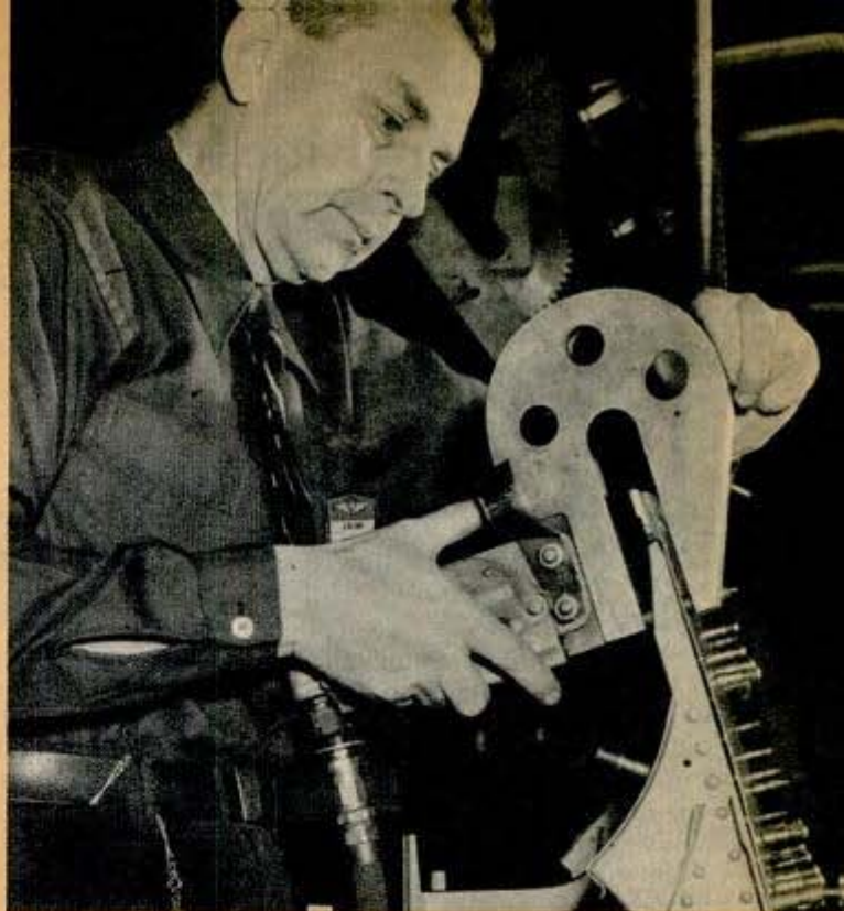
Douglas Aircraft Co. photo Aircraft worker devised squeeze yoke he uses with pneumatic gun for riveting end of wing. It eliminates need for bucking. Below, Navy officer turns coconut sculptor
