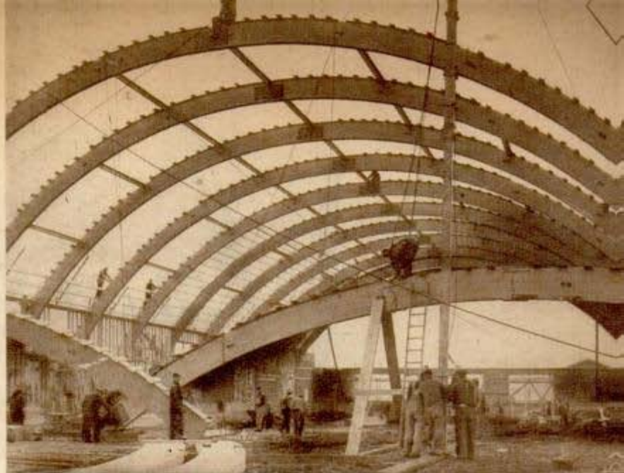
After arch is built up of plank laminates, clamps are used for shaping. Below, glue wheel takes guesswork out of applying correct amount to wood
