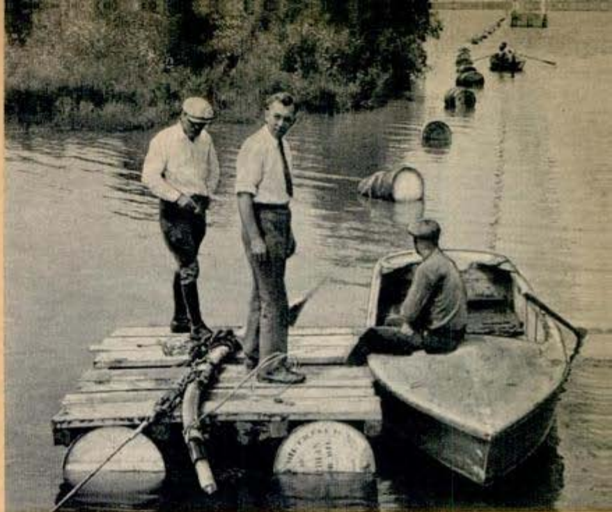
Pontoon method is used to lay submarine telephone cable across river, above. Coaxial cable amplifier, left, can handle frequency band up to 3,000,000 cycles wide
