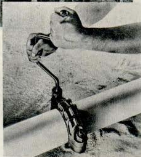
Above, "switch yard" for pipe line from India was installed by U. S. Army Engineers. Right, bolts on the completed joint are tightened after rubber gasket ring has been slipped over end of pipe. Below, GI takes "pulse" of line at pressure gauge
