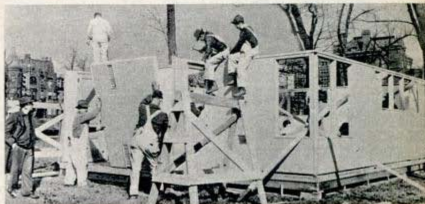
House nears completion (above) as panels for pantry and broom closet are raised into position. Below, completed four-room house designed as temporary home for British families has five cheery front windows
