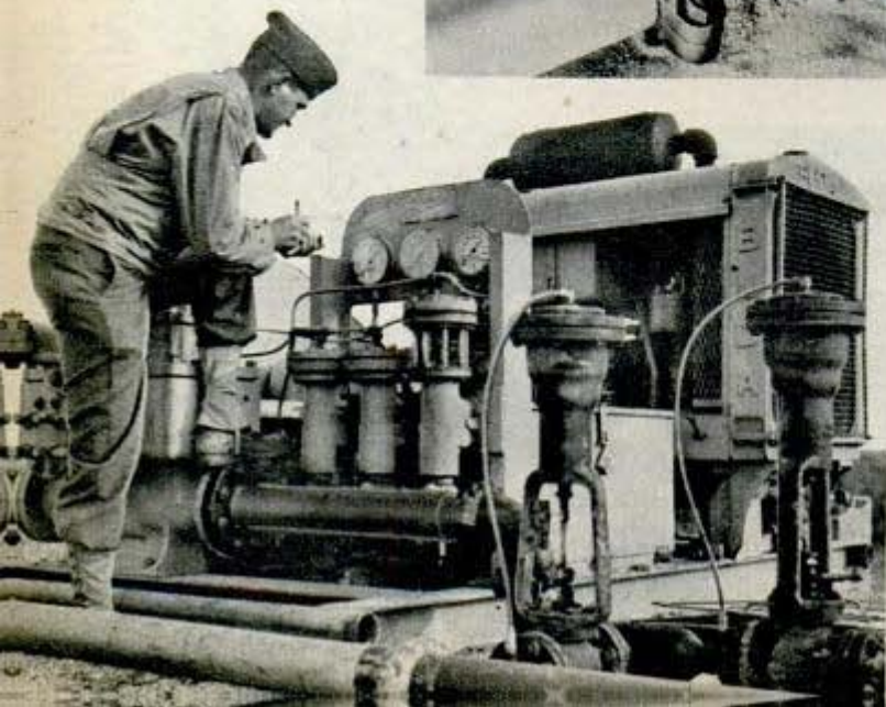
Above, "switch yard" for pipe line from India was installed by U. S. Army Engineers. Right, bolts on the completed joint are tightened after rubber gasket ring has been slipped over end of pipe. Below, GI takes "pulse" of line at pressure gauge
