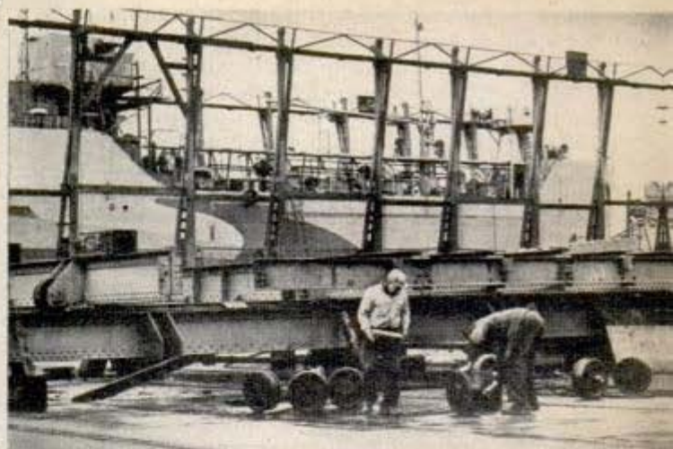
Cradles (above) rest on the shore while iron wheels are removed and greased. Below, two of the cradles, one carrying a ship, are ready to slide down the rails into water
