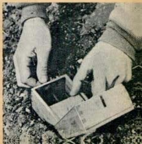
Contact with strings fastened to two fuses sets off mine below, left. Trip igniter in bottom of mine, center, explodes booby trap under it. Below, right, deft hands of an engineer make wooden box mine harmless
