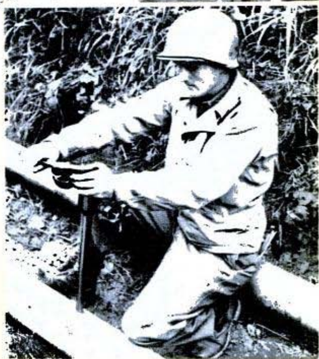
Tanker discharges cargo at overseas port. Right, sample is taken from pipe to test quality of oil
