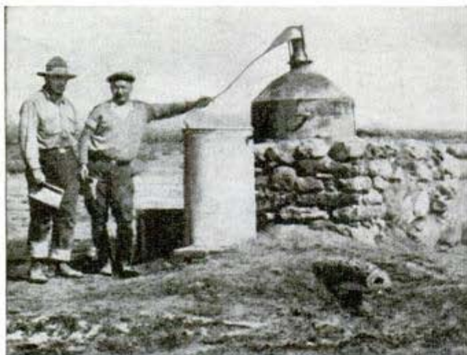
Crude still on beach produces drinking water from the sea
