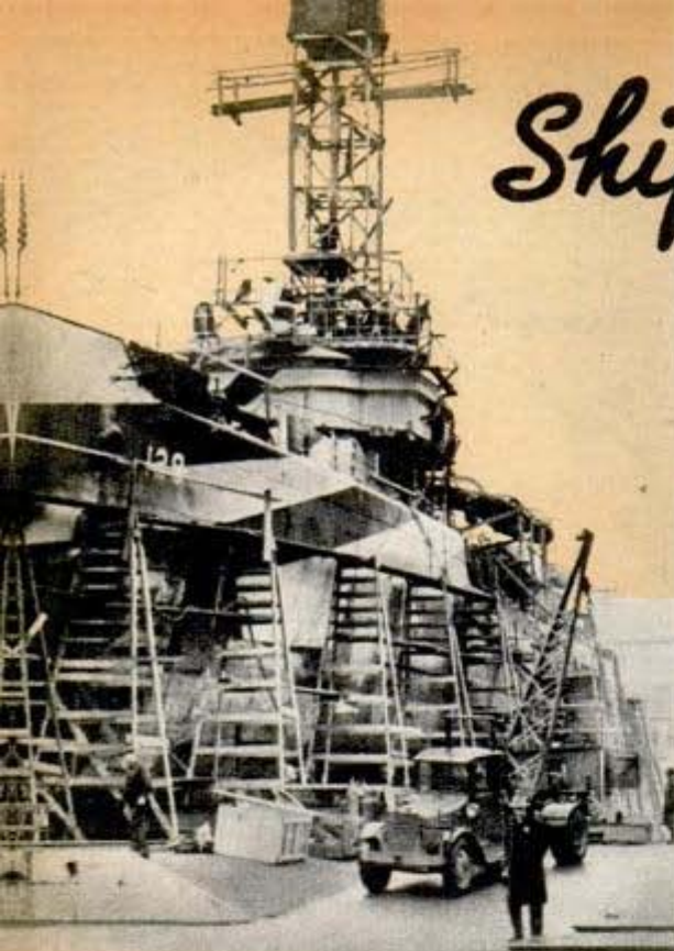
Cradles (above) rest on the shore while iron wheels are removed and greased. Below, two of the cradles, one carrying a ship, are ready to slide down the rails into water
