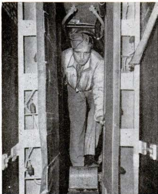
Temporary fuel tanks fill B-24 bomb bay on long ferry flights
