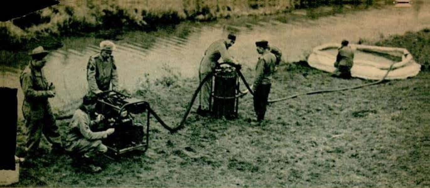
This portable apparatus can produce 15 gallons of pure drinking water per minute from a jungle stream
