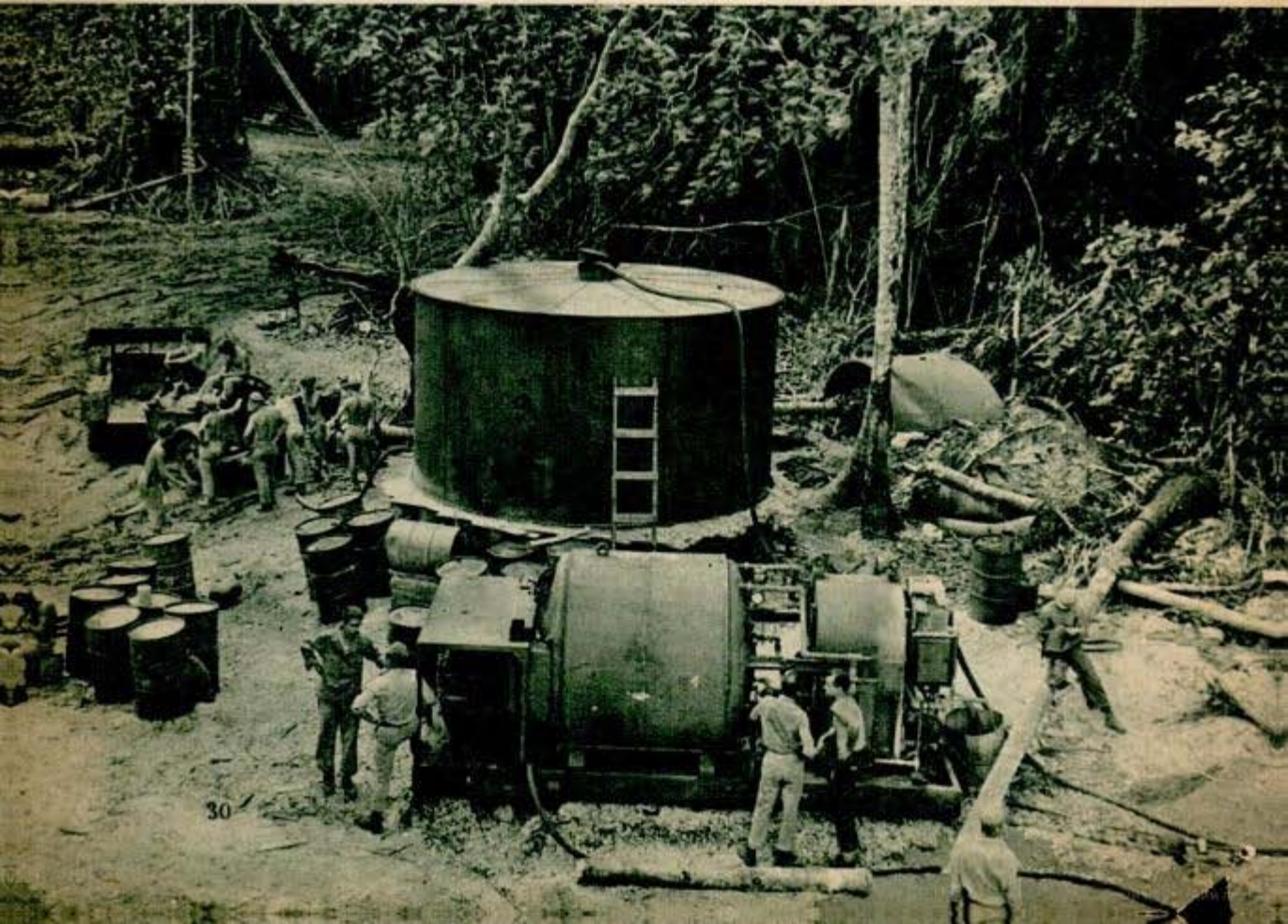
Tank of water purification unit on island in the Pacific can supply 10,000 soldiers with one gallon apiece
