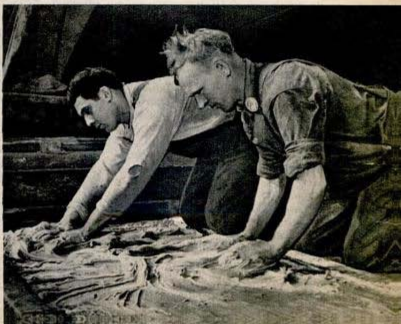
Flagman signals that tide has reached peak and big ship can start first trip. Below, workmen spreading launching grease over special liquid wax on ways; it takes 5,000 pounds for job
