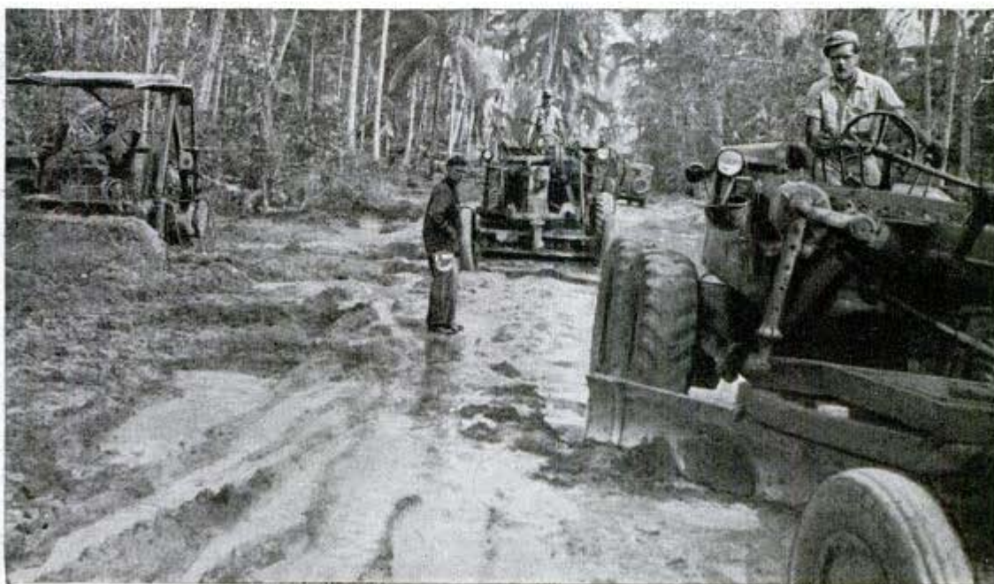
Courtesy R. G. Le Tourneau, Inc. Scraper and "tiltscraper" built for air shipment will do work of 50 men. Below, Yanks build road through jungles of Leyte
