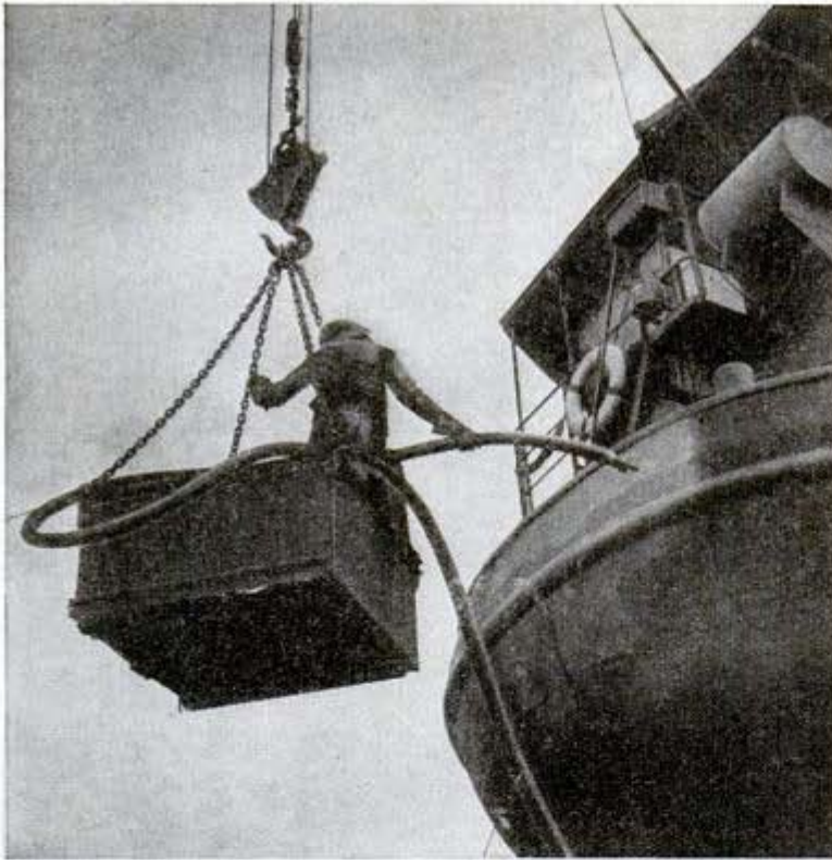
Camouflage paint is sprayed on tanker at storage depot for lake wells
