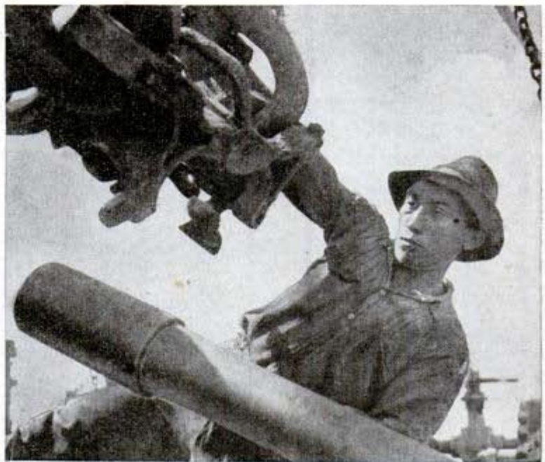
Pulling out drill pipe during operations on Lake Maracaibo
