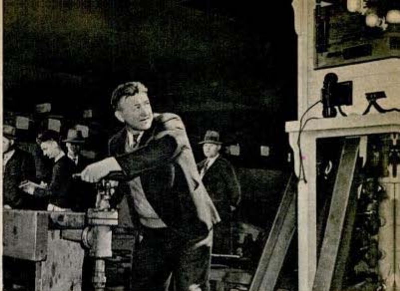
Waiting for the signal to start final act of launching. When light flashes, throttle is opened and several million pounds of ship start down the ways in the cradle built around the craft
