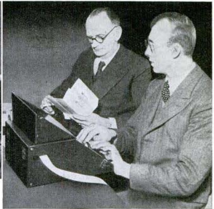
Above, a blind man taking dictation notes on a machine (below) which punches Braille characters onto tape
