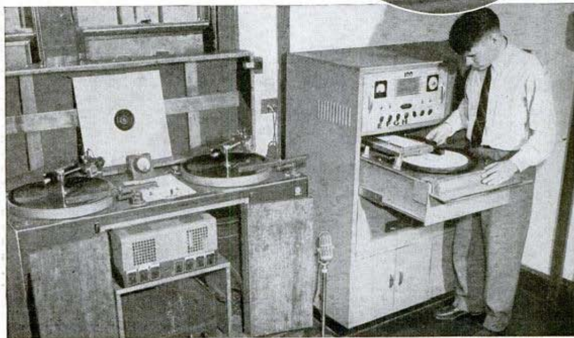
Above, data on card guide monitor as he tunes set to hear a scheduled broadcast from Berlin. Right, stepping on switch enables monitors to make instant checks of frequencies and keep dial settings accurate. Below, a supervisor records program on Memovox machine. Lone disk runs two hours. Other console holds a high-fidelity unit
