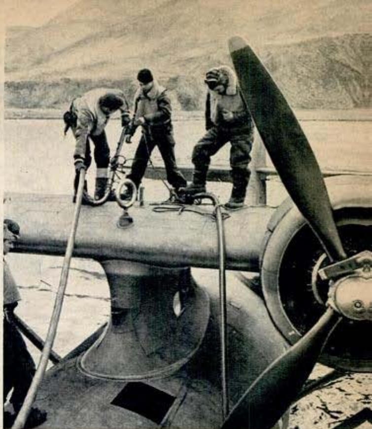
Above, refueling from a seaplane tender is a ticklish job even in calm weather. Below, forced down somewhere in the Pacific, a seaplane is hoisted aboard an assault transport after being towed alongside by a small boat
