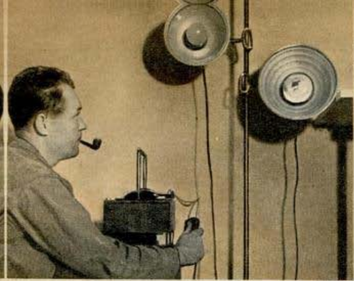
For indoor lighting amateur uses a specially wound transformer to double output of photo-floods. Right, scrim softens light for close-ups
