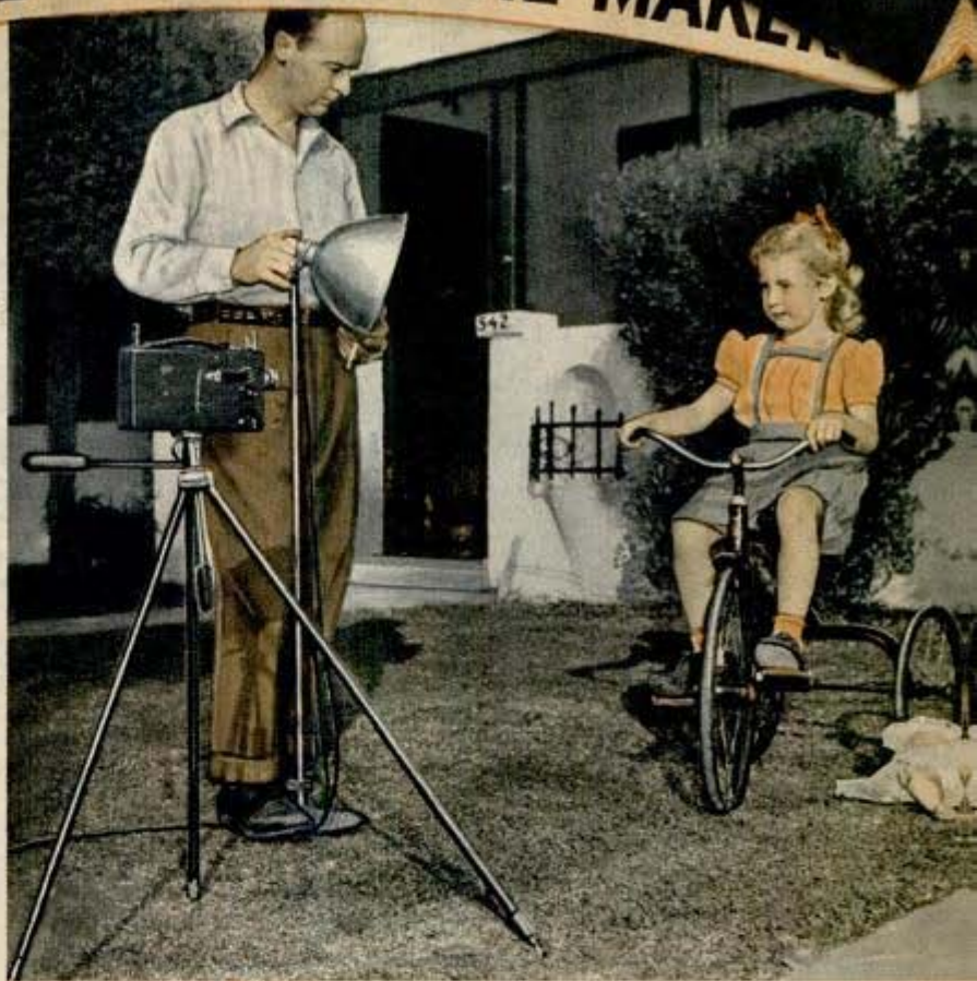
Photoflood lamp is positioned for an outdoor motion picture to lighten the shadows caused by bright sunlight. Below, parts of a movie projector are rigged up for printing extra copies of home movies
