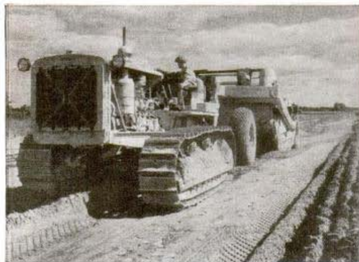
AAP photo Above, loading a tractor aboard a glider for Air Commando Force operations in Burma. Below, "Cat" with scraper widens banks for rebalasting along Duluth branch line of Great Northern Railroad
