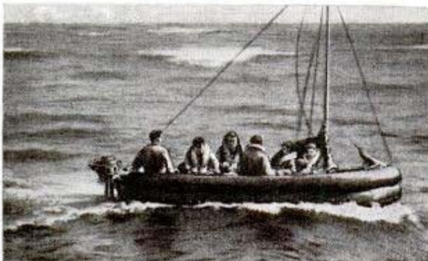
3 As boat package is opened, inflation automatically begins, while survivors cling to lines. Any of the packages will support an injured or exhausted man, who can be quickly drawn to raft.
