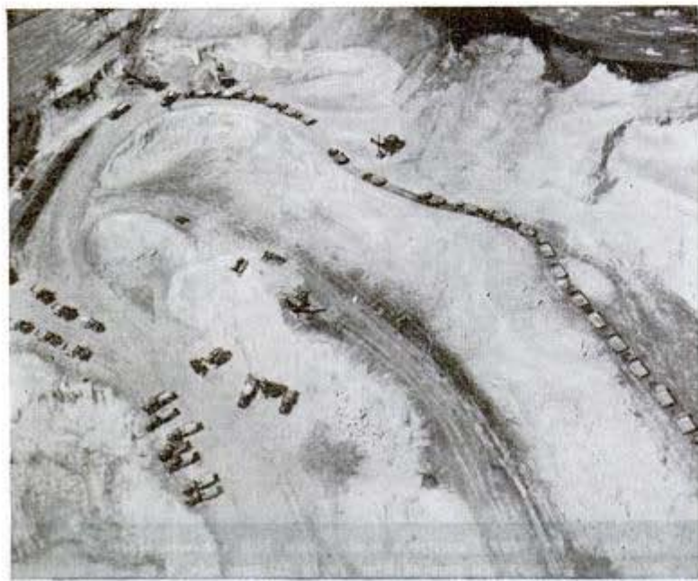
Trucks are lined up to move a mountain of crushed white coral to surface runway on Saipan
