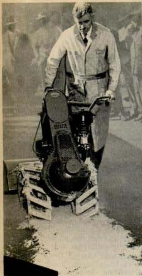
Left, Rototiller making soil "cement." Above, it churns earth into even seed bed
