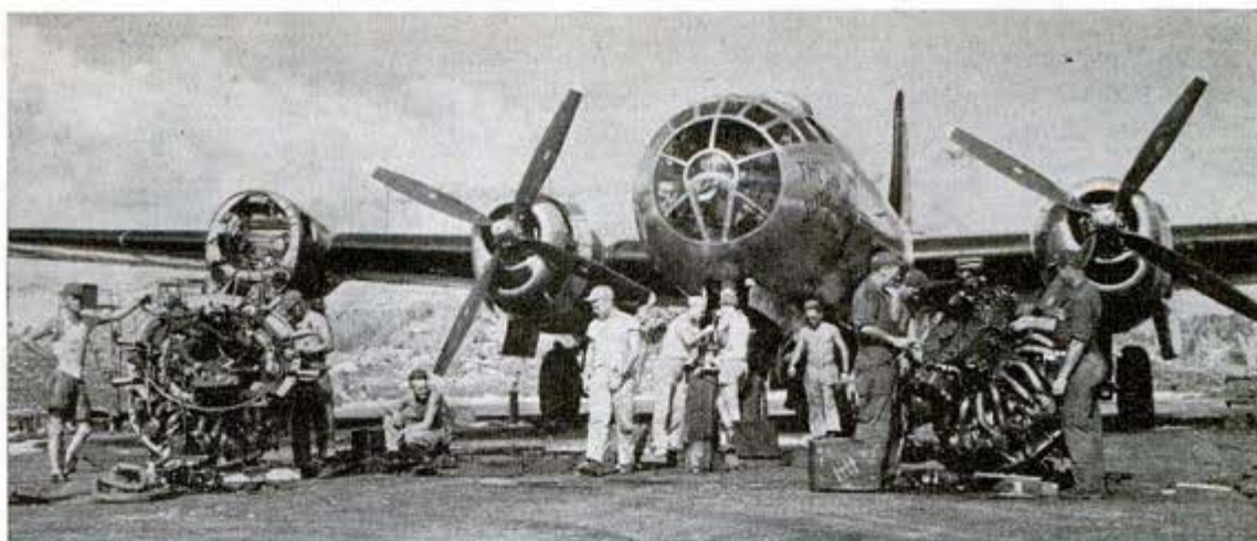
Superfortress gets its first engine change at 20th Air Force headquarters on Saipan Island
