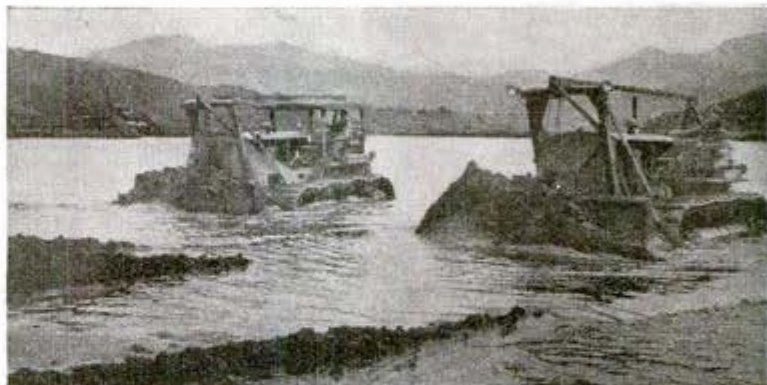
Yoke of giant earthmover, above, frames land levelers busy in Iceland. Below, bulldozers scrape Alaskan inlet to obtain sand fill for runway
