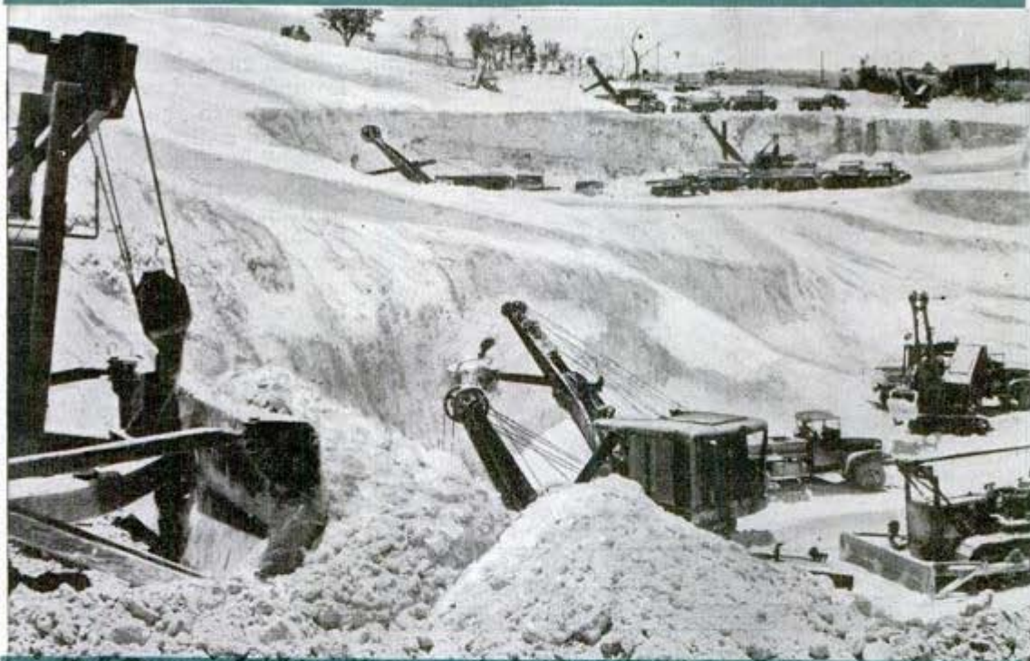
Cutting up a coral mountain on Saipan, engineers get prized construction material for B-29 bases. Above, bulldozer pushes coral to waiting trucks. Below, Superfort soars from smooth coral runway AAP photos
