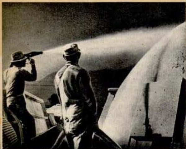
Left, concrete is sprayed on a balloon, which was inflated with an air pressure of 1\frac{1}{2} ounces per square inch. The new engineering building at Loyola University in Los Angeles is shown from the inside (above) and outside (below) Photos by Maynard L. Parker
