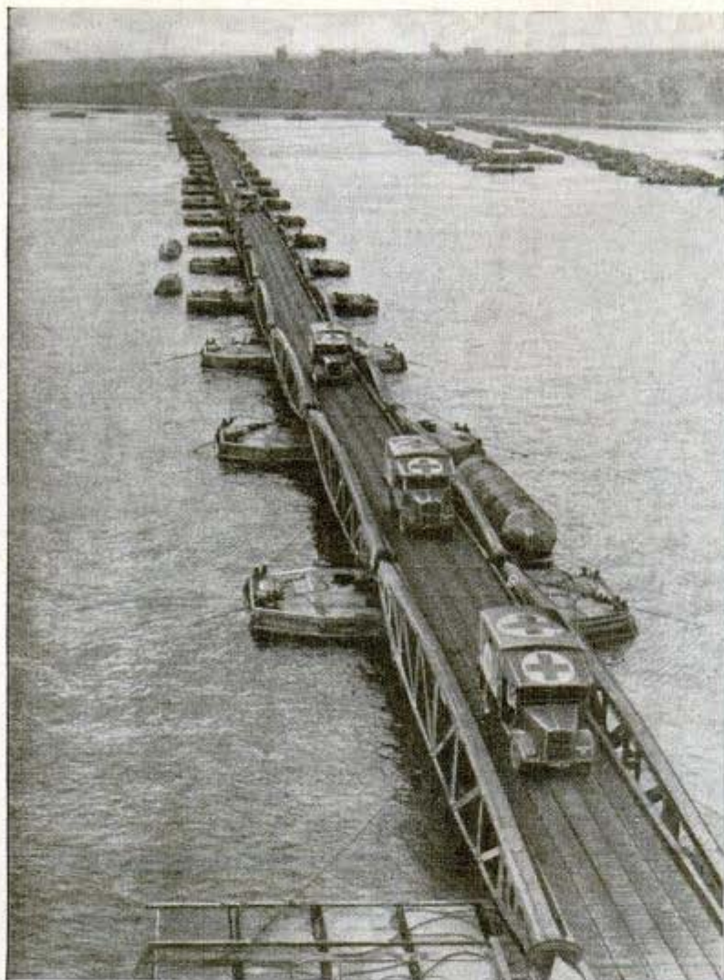
Above, a British prefabricated pier at Normandy made up of small bridges resting on floats. Below, a wilderness bridge on the Alcan highway
