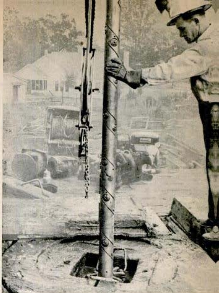
Above, preparing to run casing gun perforator into hole. Left, reading magnetometer which reveals mass of rock under ground that may form oil basin; gravity meters are used for the same purpose. Midway on derrick below, operator can be seen steadying pipe as rotary helpers on the floor below "stab" the pipe
