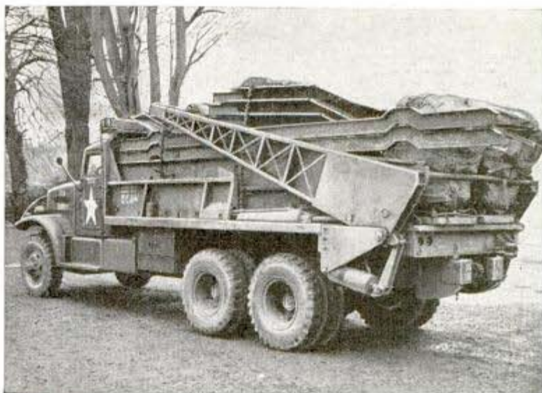
Above, overall view of a loaded bridge truck equipped with hydraulic crane. Among assorted construction equipment are two complete trestles
