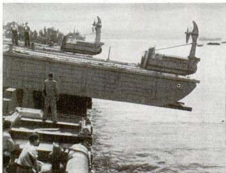
Landing boat's crew jumps on board (above) as craft is lowered to the ship's rail. Below, a row of pontoon barges equipped with self-propulsion units is launched by Seabees from the deck of an LST
