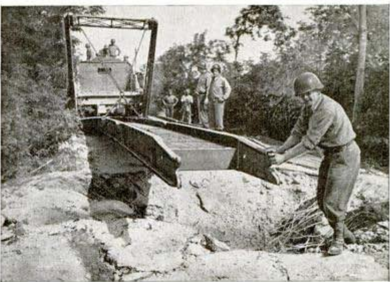
Above, hydraulic truck crane lays final treadway section on ponton bridge over the Seine River. Below, bridging gap left by a blown-out span
