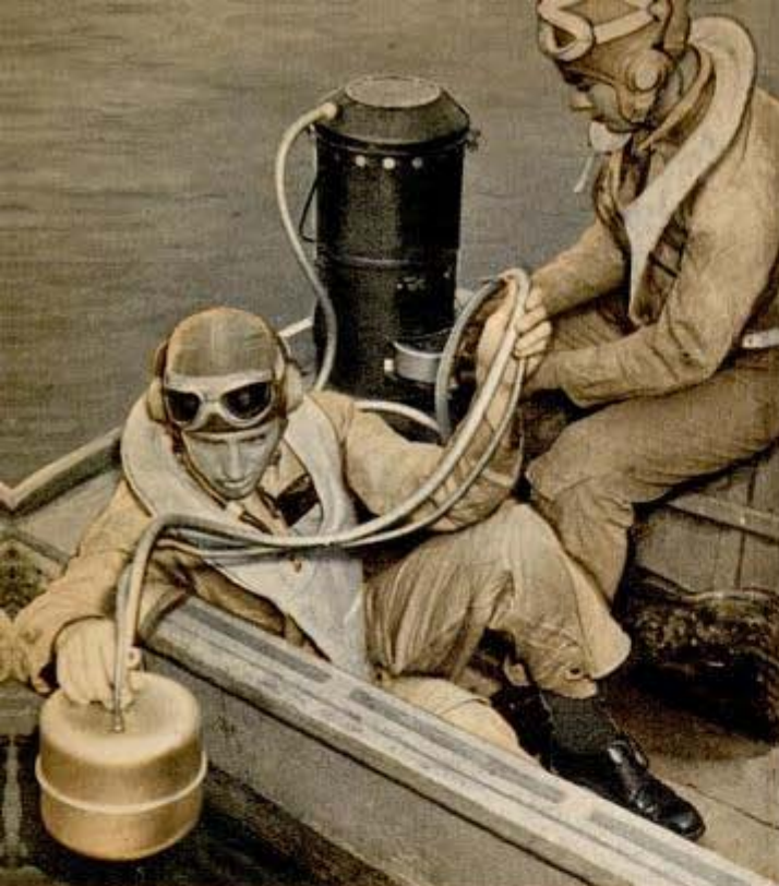
Above, larger rafts carry apparatus which distills several quarts of fresh water an hour. Right, lookout in car of blimp scans the surface of the ocean
