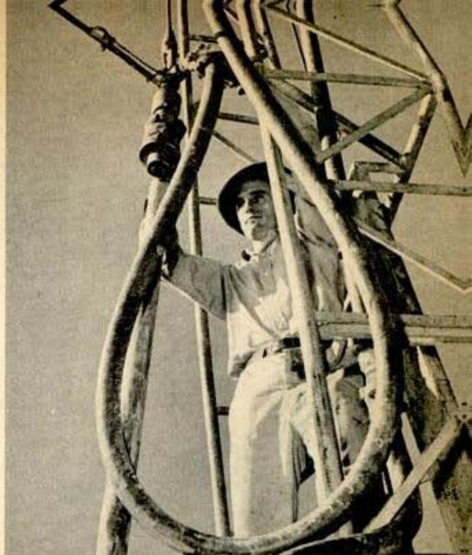
Mast-derrick of rotary drill is mounted on a truck and is used for drilling the seismograph shot holes. At bottom of page, gravity meter is rock "detective"
