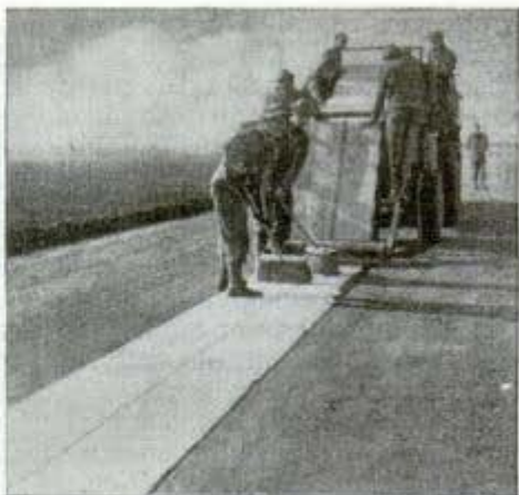
Above, laying cloth-paper runway on a new landing strip. Below, threading "stamp licker" with new roll of P.H.S.
