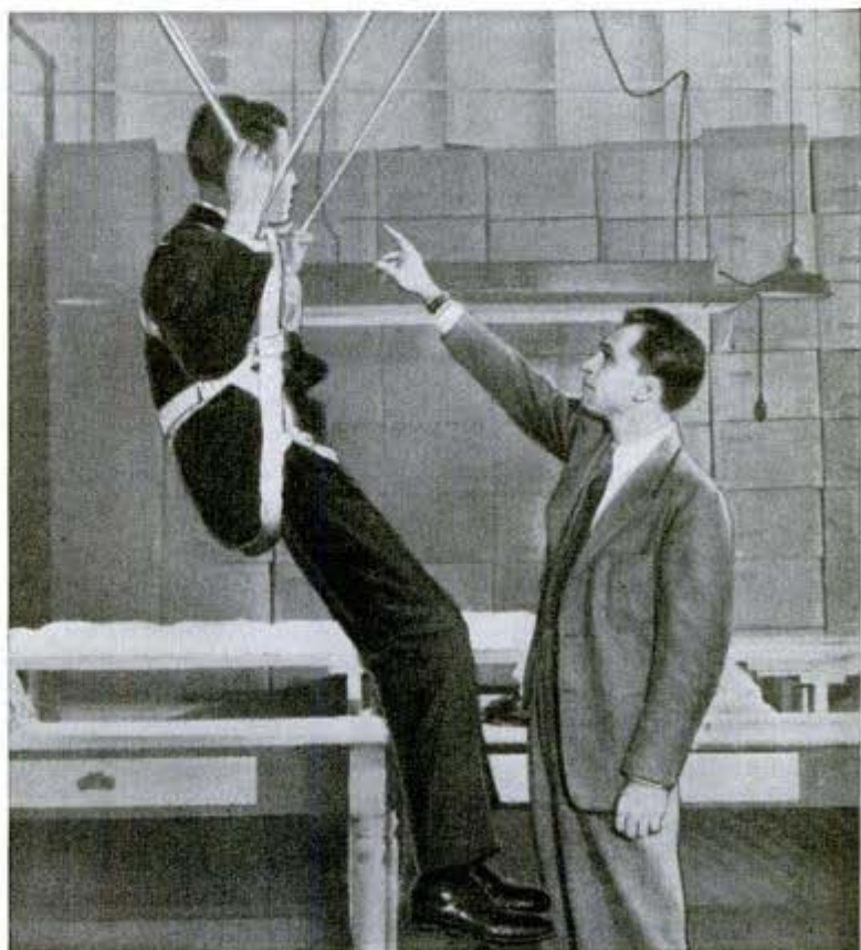
Above, nylon threads are woven into parachute shroud lines. Below, suspension rig determines how harness innovations fit under body weight
