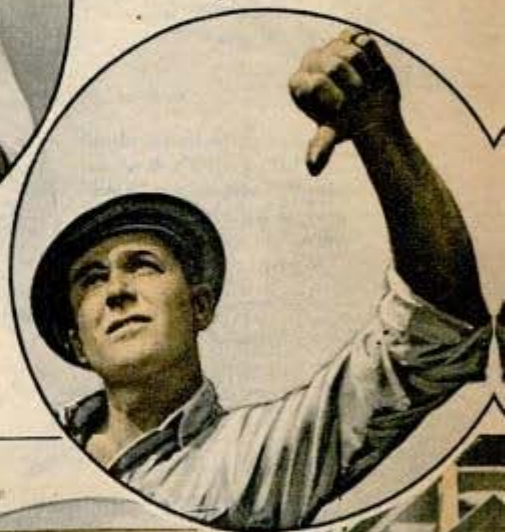
Below, by thumbs down, signal crane operator is told to lower boom
