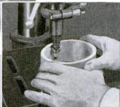
CUT SLOTS IN BOX BODY TO TAKE PINS IN LID
