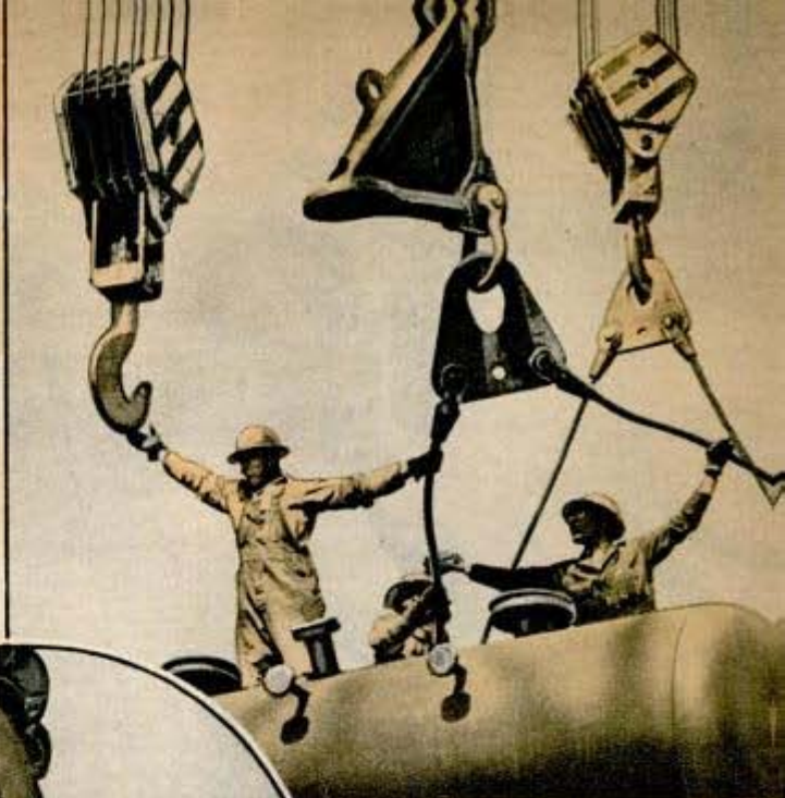
Below, by thumbs down, signal crane operator is told to lower boom
