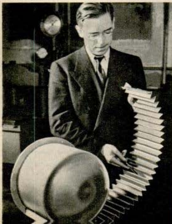
Above, bow and side view of SS Chattanooga, cruise liner which will have Plexiglas pilot house and cargo doors like a landing ship. Below, instead of welding, metal is bonded to metal by resin cement U. S. Stoneware Co.
