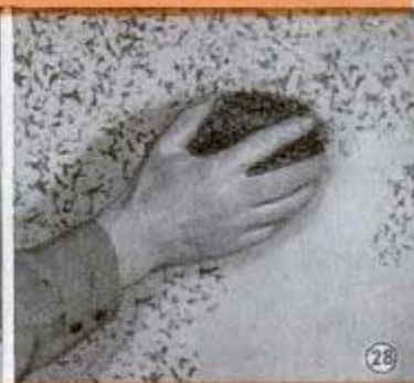
SPONGE MOTTLE —Trim sponge so that it has a flat side. Dip in water to soften, then wring dry. Press onto the color slab, Fig. 27, then transfer the paint to the wall. Two color mottles are very effective
