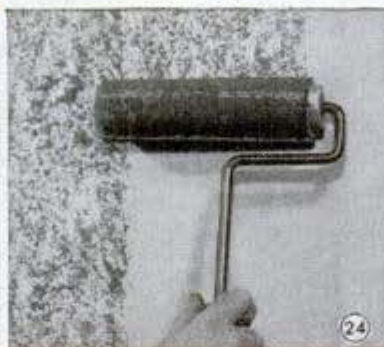
ROLLER MOTTLE —Pick up color on roller, Fig. 23, then apply roller to wall, being careful not to overlap. Two times over makes a heavier mottle, as shown in Fig. 25. Use a stippling roller, not a roller coater
