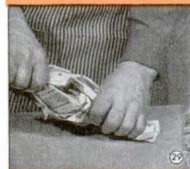
NEWS ROLL —Use a pigmented ground coat for this, not water paint. When dry, apply color coat of water paint. Crumple a sheet of newspaper, Fig. 29, and roll this over the fresh paint, Fig. 30. Change the paper as often as may be necessary. Fig. 31 shows a heavier pattern obtained by double rolling
