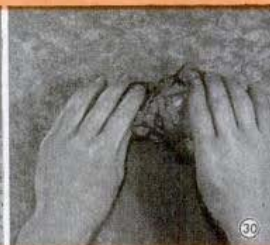
NEWS ROLL —Use a pigmented ground coat for this, not water paint. When dry, apply color coat of water paint. Crumple a sheet of newspaper, Fig. 29, and roll this over the fresh paint, Fig. 30. Change the paper as often as may be necessary. Fig. 31 shows a heavier pattern obtained by double rolling
