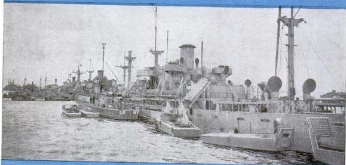
Above, one sector of breakwater created by line of sunken ships near "U. S. Mulberry" harbor off the Normandy coast. Below, panoramic view of Omaha beach before the Mulberry was set up. Barrage balloons hover over mighty assemblage of shipping as Allies pour an unending flow of supplies ashore
