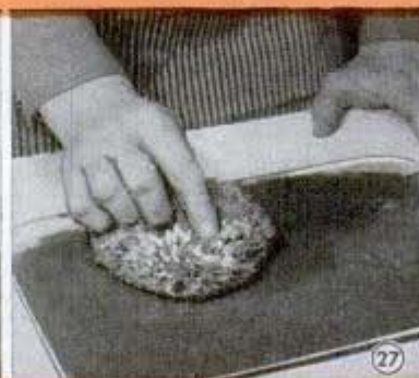
SPONGE MOTTLE —Trim sponge so that it has a flat side. Dip in water to soften, then wring dry. Press onto the color slab, Fig. 27, then transfer the paint to the wall. Two color mottles are very effective
