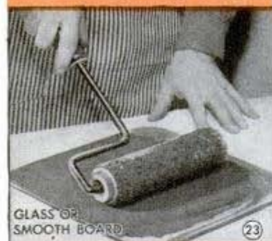
ROLLER MOTTLE —Pick up color on roller, Fig. 23, then apply roller to wall, being careful not to overlap. Two times over makes a heavier mottle, as shown in Fig. 25. Use a stippling roller, not a roller coater
