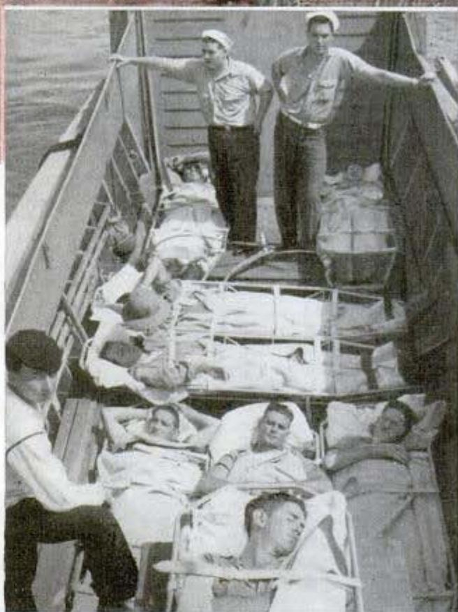
of webbing-strap. Six to eight litters can be carried. The same type of support can be installed in C-47 cargo aircraft, giving a capacity of 24 patients. Larger ships can carry up to 60. Many different types of planes, even gliders, help carry wounded.
