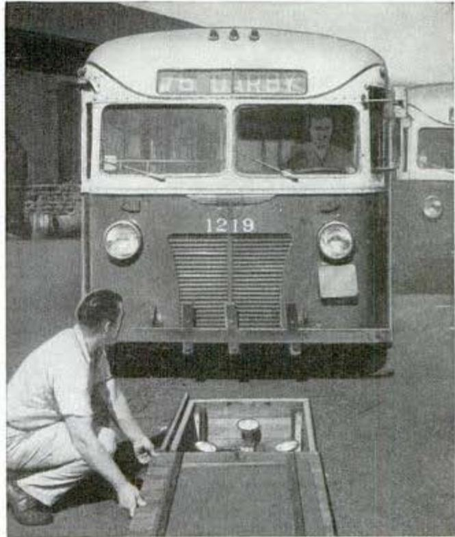
Philadelphia buses left standing in the yard are kept warm for easy starts in cold weather by parking them over infrared heating pits. Each pit, measuring 27 by 42 by 16 inches, contains three 250-watt drying lamps which direct heat on the engine when a bus is parked over a pit. Unable to build more garages because of wartime restrictions, the bus company rigged up the pit system at a cost of \$3,000 to save the 5,000 gallons of gasoline it would take to idle the engines all winter.
