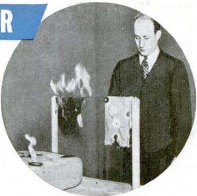
Demonstration shows that fabric treated with ammonium sulfamate ~~chars~~, whereas an untreated cloth blazes up
