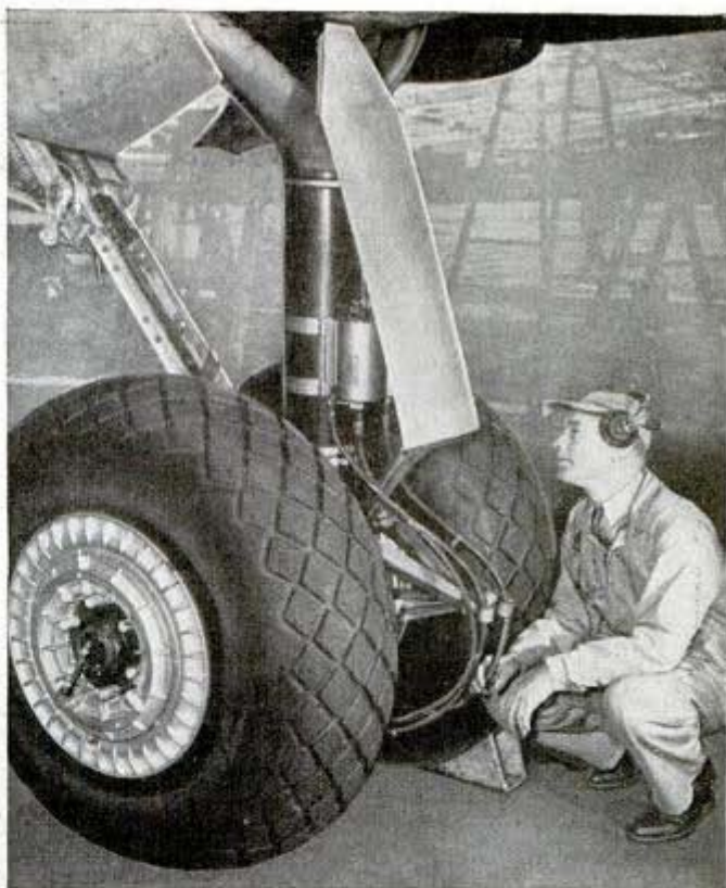
Above, looking for flaws in hydraulic brakeline installations. Left, the slenderness of an A-20 cockpit as seen from above
