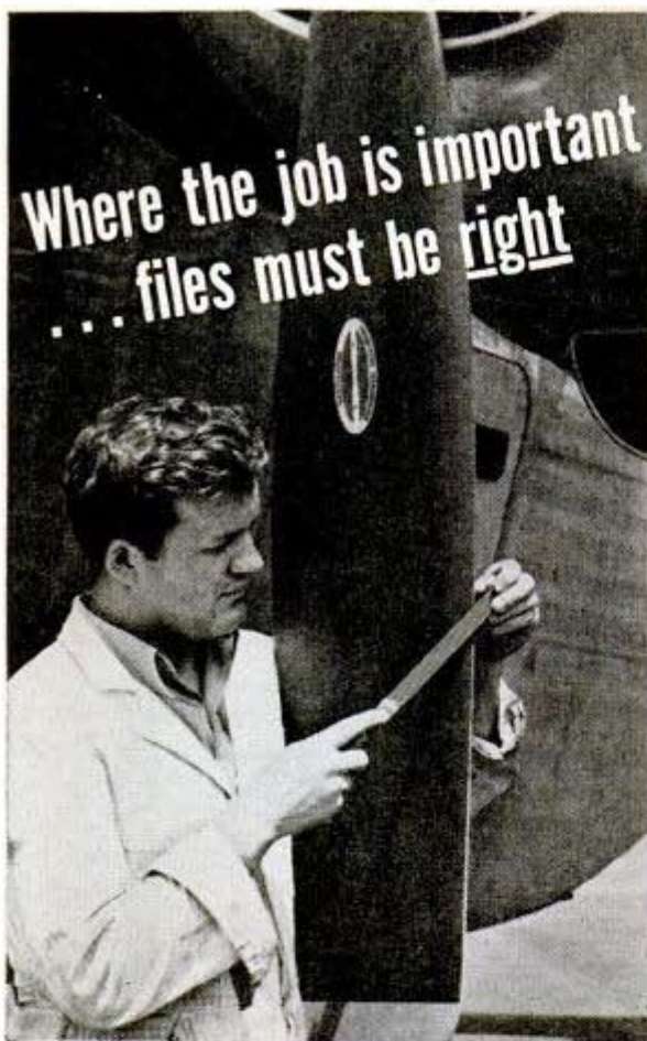
Filing nicks out of propeller blade of Budd-built RB-1 transport plane.
