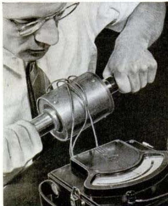
Torquemeter registers slightest twist of the shaft
