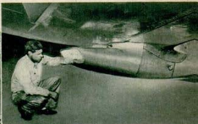
Inspecting non-drag air intake scoop. It leads cold air to radiator and expels it without the loss of speed
