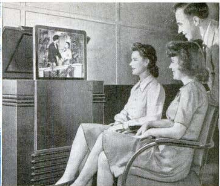
Home television screen on RCA experimental set retracts into the cabinet. Image is reflected to the 13½ by 18-inch screen
