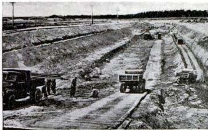
Above, a huge basin is excavated where the bottoms of concrete ships will be laid. There are three such basins in McCloskey & Co.'s shipyards at Tampa, Fla. Length of the ships is 366 feet
