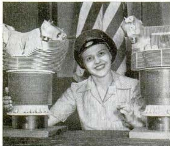
Worker compares the new fins (right) to the old type
