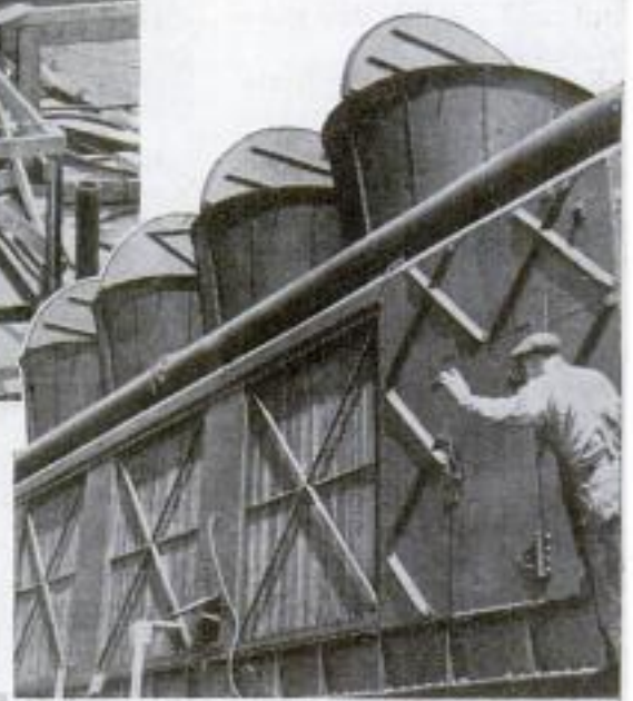
Above, final assembly work on the boiler car of one of the 5,000 kilowatt trains. Each train, consisting of eight cars, is ready to follow on heels of an advancing army, stop at the coal stockpile of a wrecked power station and feed current to factories and homes. All the trains can operate in temperatures from 40 degrees below zero to 95 above. After the war they will be available for disaster emergencies
