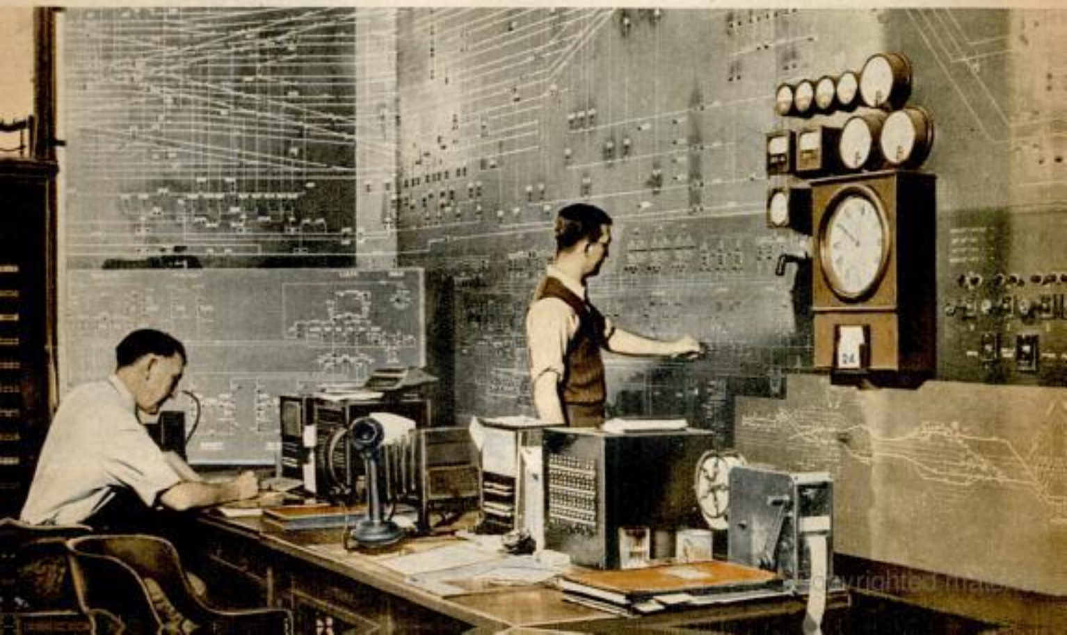
One of 88 Pennsylvania passenger trains a day between the two cities leaves the Broad Street Station in Philadelphia for New York. Below, the power director in New York City routes 11,000-volt current to wires
