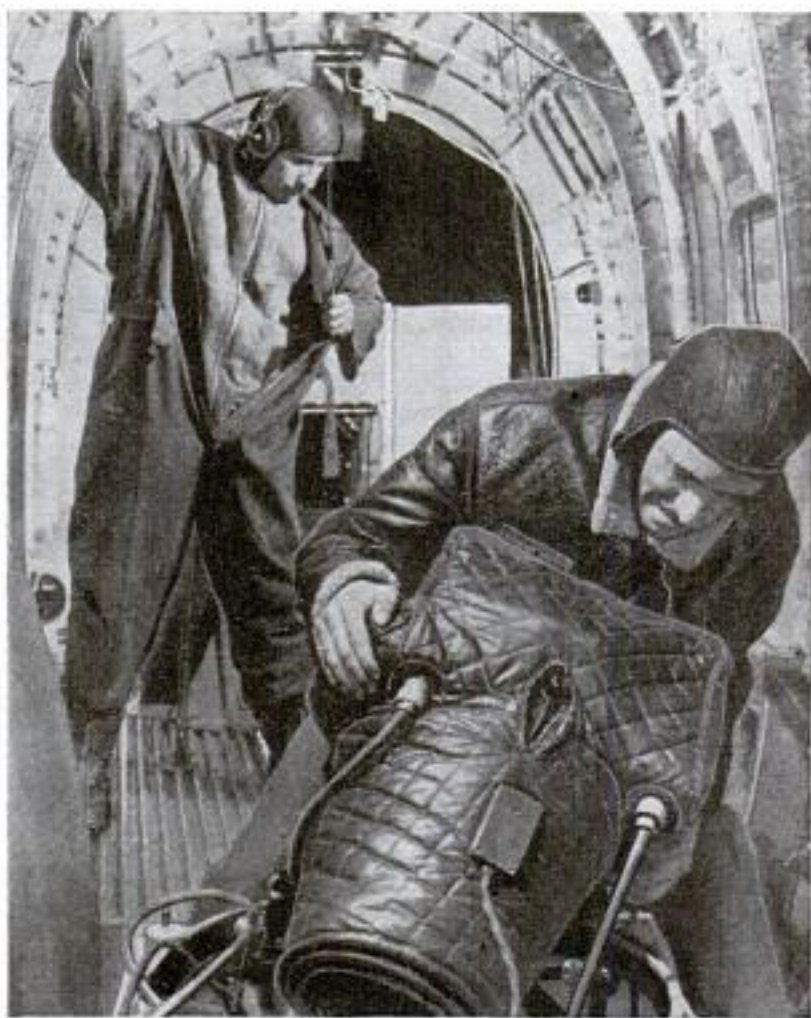
Camemen rig up an electrically heated camera for high altitude AAF Materiel Command photo
