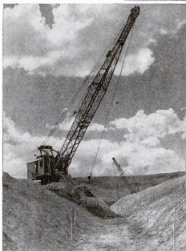
Concrete canal is fed from reservoir of Friant dam in background. Left, digging part of 37-mile canal
