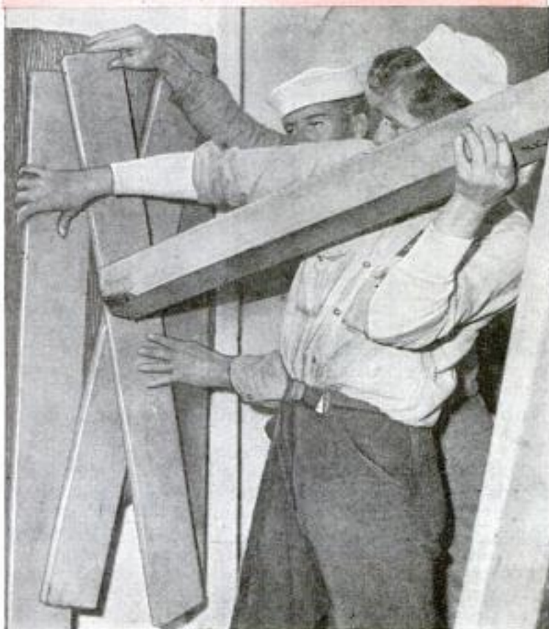
Seamen at a Navy damage-control school wear self-contained oxygen breathing apparatus while rehearsing their work. Below, recruits learn to close small holes in a ship's hull by means of a mattress, held in place with wooden planks and shoring
