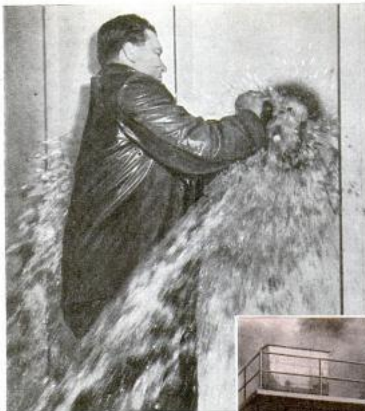
Top, Navy school teaches technique of plugging a small hole in ship's side
