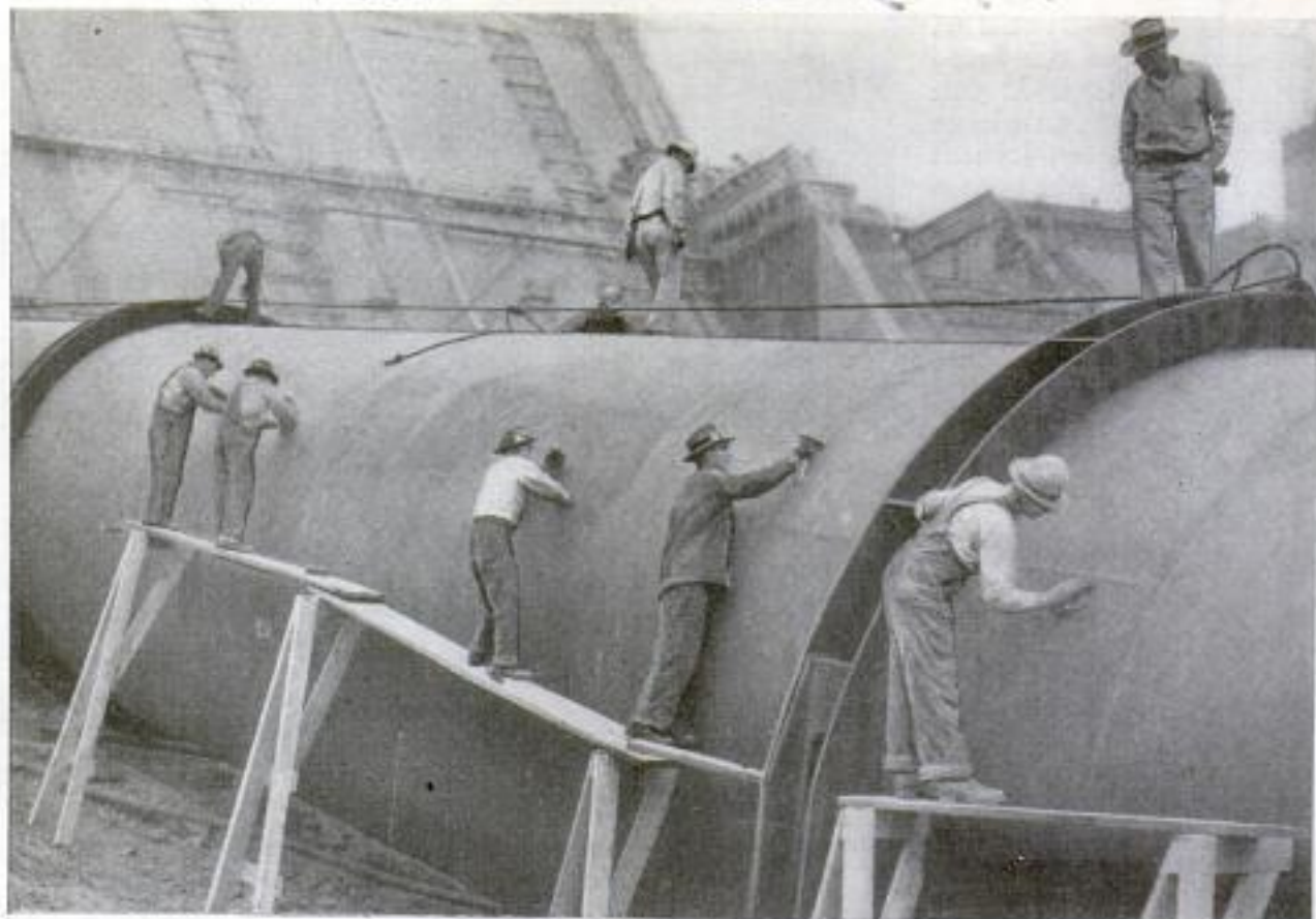
Huge penstock on Shasta dam is prepared for painting. At left, sheep on Grand Coulee
