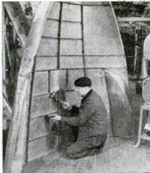
Above, part of the forward deck section of the craft, which is fireproof, worm-proof, leakproof and resists corrosion
