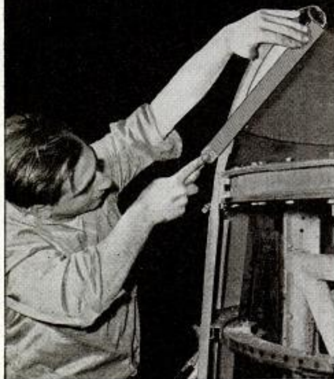
Photo courtesy Republic Aviation Corp.— Special-file operation on edge of casing.
