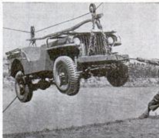
The "Little Burma Road," a trucker's nightmare 11½ miles long, is a rugged testing ground for jeep combat drivers at Camp Walters, Tex. To get cars over bridgeless streams, they must be hauled over on a suspension line (above) or wrapped in big tarpaulins and floated over (upper left)
