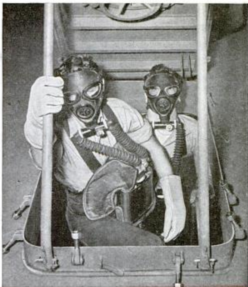
Seamen at a Navy damage-control school wear self-contained oxygen breathing apparatus while rehearsing their work. Below, recruits learn to close small holes in a ship's hull by means of a mattress, held in place with wooden planks and shoring
