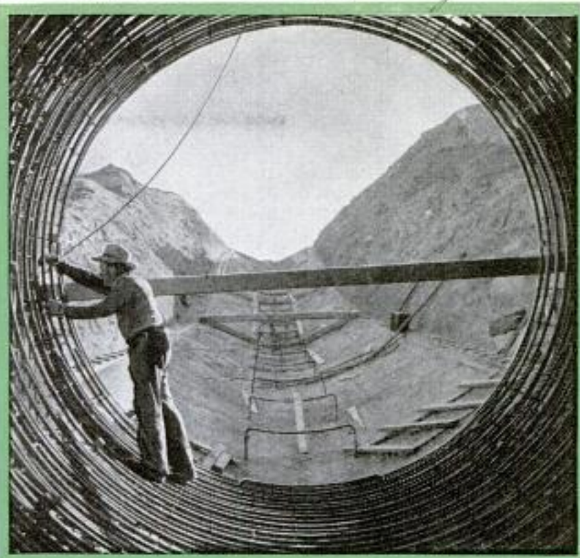
Concrete tube with steel ribs will carry waters to reclaim arid tract in San Joaquin Valley, part of a project to create 2,000,000-acre garden spot. Below, Boulder dam holds record for million-kilowatt capacity
