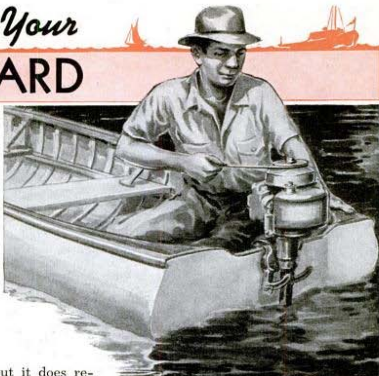
① REMOVING NUT THAT TIGHTENS FLYWHEEL
