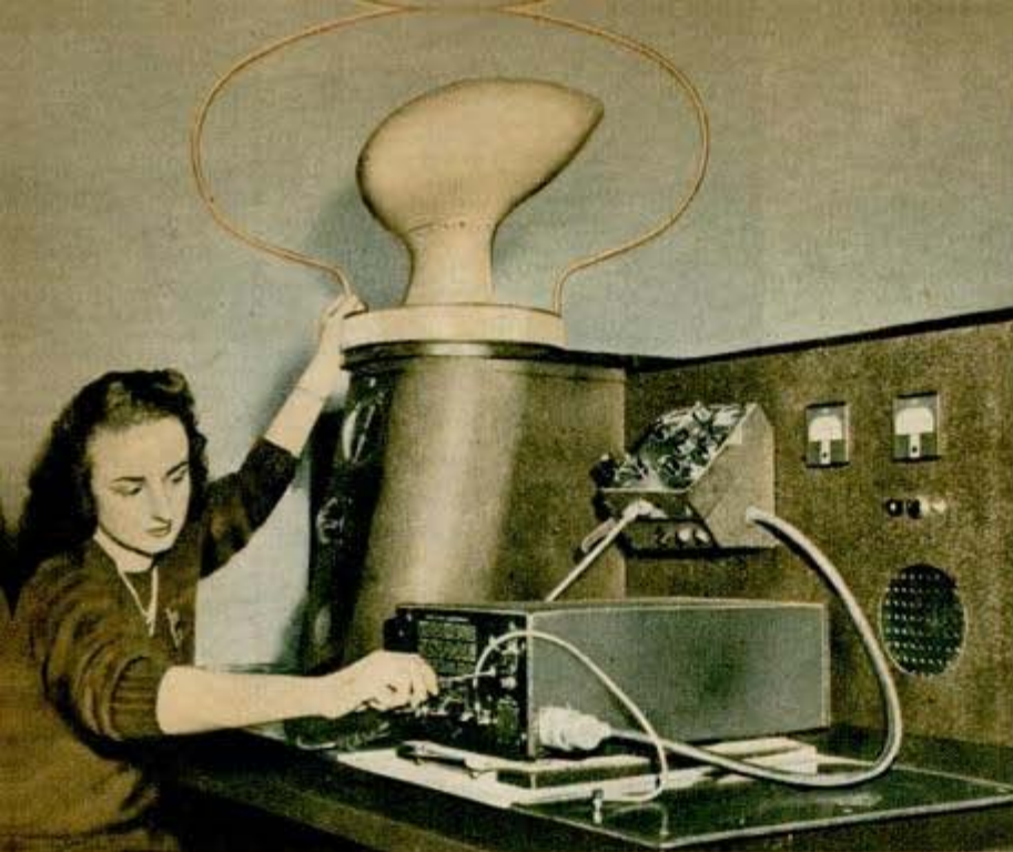
Testing an airplane radio with the help of dummy antennas in the radio laboratory, above. Two smaller altitude chambers at the Douglas factory are engaged in research, testing and improving the myriad materials and parts that make up modern aircraft. In one area, engineers are rolling a nose wheel down an incline, causing it to hit the ground with an impact similar to that of a hard landing. Electric strain gauges and a motion picture camera record the
