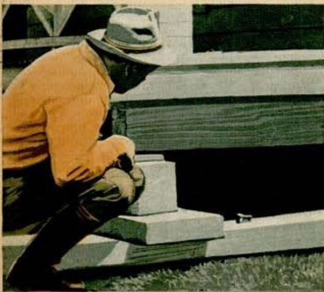
Houses on spongy peat soil are jacked up to keep floors level. Below, triple wheels on truck prevent sinking; all vehicles are specially equipped
