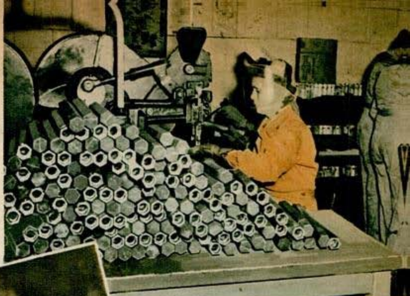
Machine operator (above) corking the vents in magnesium incendiary bombs
