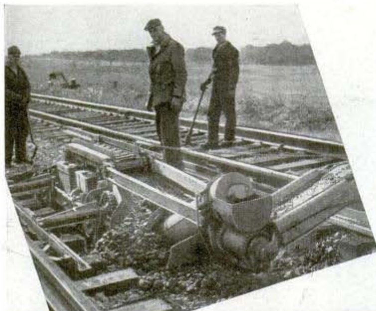
Left, cleaning ballast on Bessemer & Lake Erie R.R.; 5,000-horsepower electric giant below hauls New Haven freight at passenger-train speed
