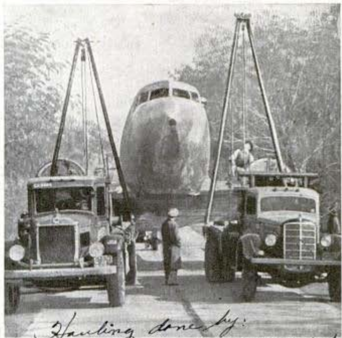
Rigging lifted fuselage at narrow bridges; below, 115-foot oil tower
