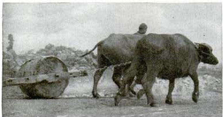
Water buffaloes help surface parking area near airstrip by pulling crude roller. Below, Chinese mechanics rebuilding C-46 at open air "factory"
