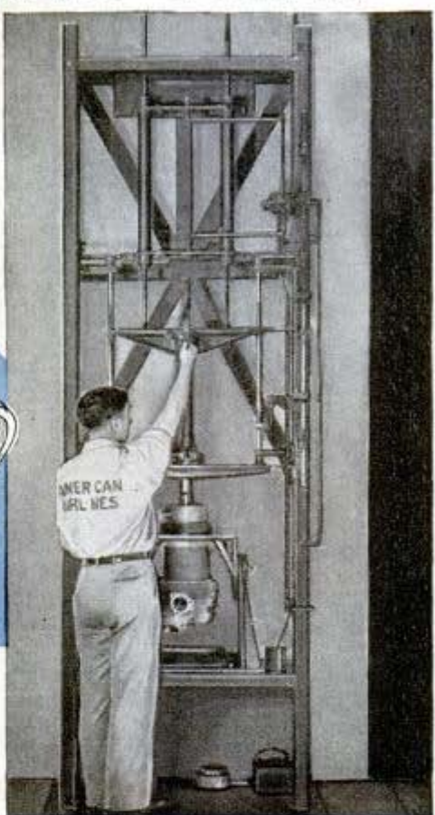
Courtesy Curtiss-Wright Corp. The "G. I. Joe's" of industry are showing ingenuity in discovering ways to increase the flow of war goods. Here are some innovations by workers: above, plastic bell cap center punch which locates the exact center of hole. Right, a polisher for interior of cylinders
