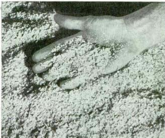
Above, milling "Norepol," rubber substitute from soy beans, corn and other vegetables at Peoria laboratory of Department of Agriculture. Below, soybean flakes for plastics
