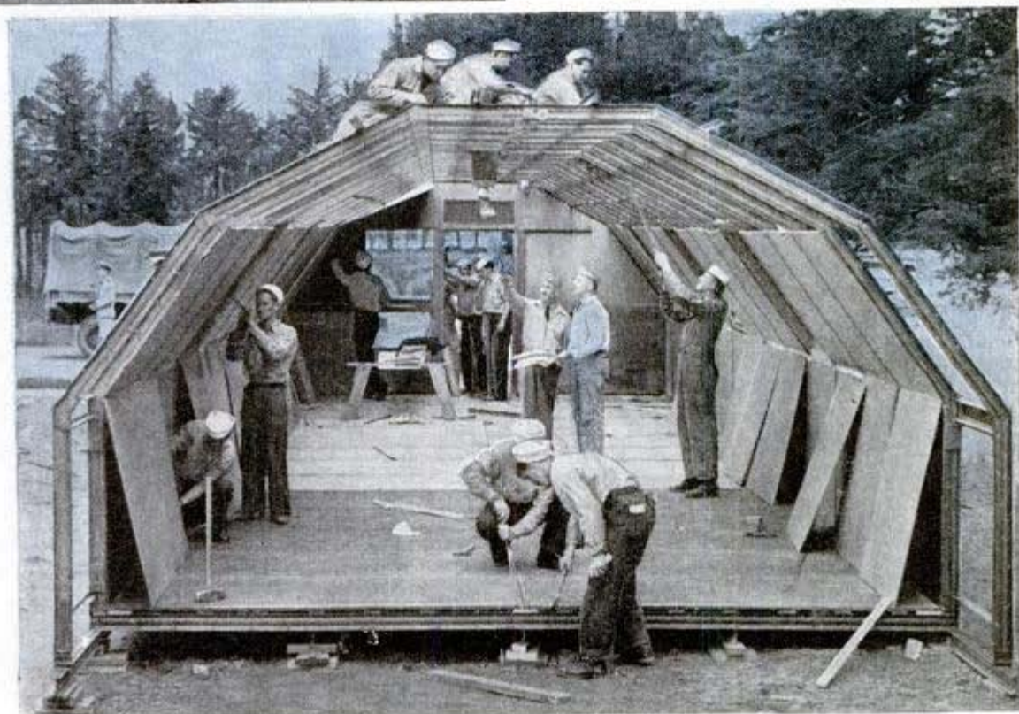
A Navy variation of the Nissen hut goes up in fast time. These huts are used from tropics to the Arctic
