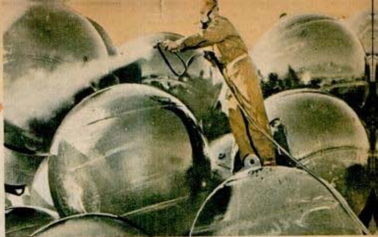
Spraying spheroid floats with anti-fouling paint to keep barnacles off. Floats get careful periodical inspections
