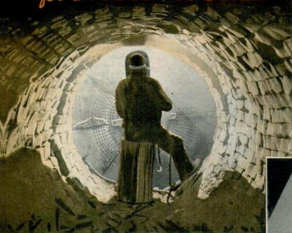
Masked workman is repairing tube mill at a cement plant
