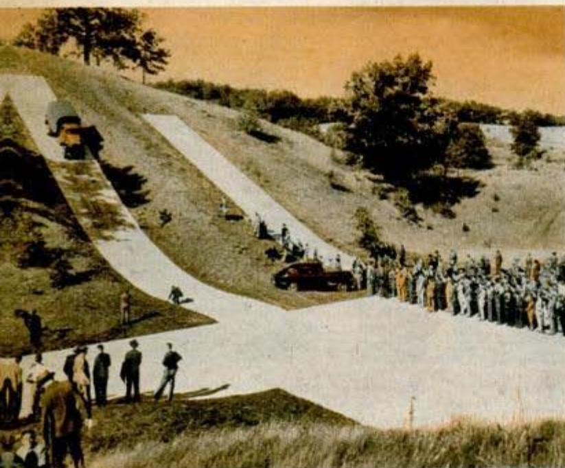
Concrete test tracks are used to check Army trucks at General Motors proving ground. Below, unique building in Los Angeles was built by pouring concrete over canvas bag filled with air
