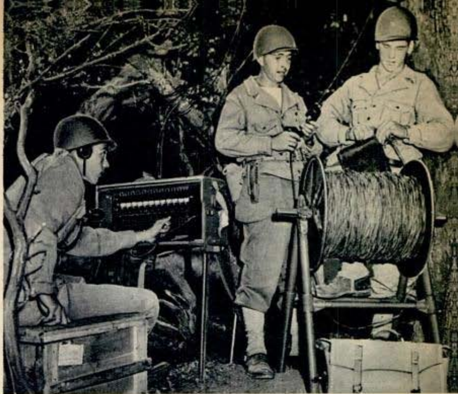
Hidden under trees, this switchboard is nerve center of artillery unit
