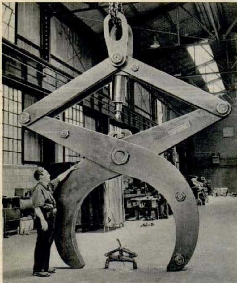
The tong is so massive it can easily pick up ingots weighing 80 tons
