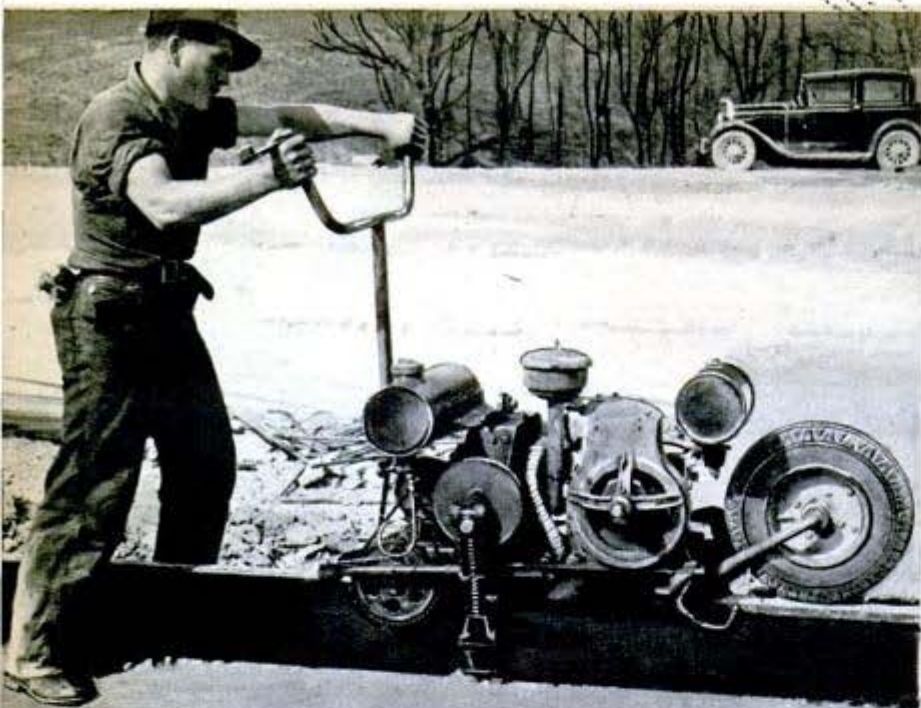
Gas-driven machine oils inside of cement form, tamps dirt on sides
