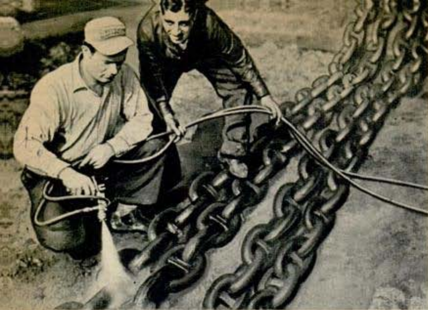
Spraying paint on anchor chain of a U. S. Maritime Commission ship
