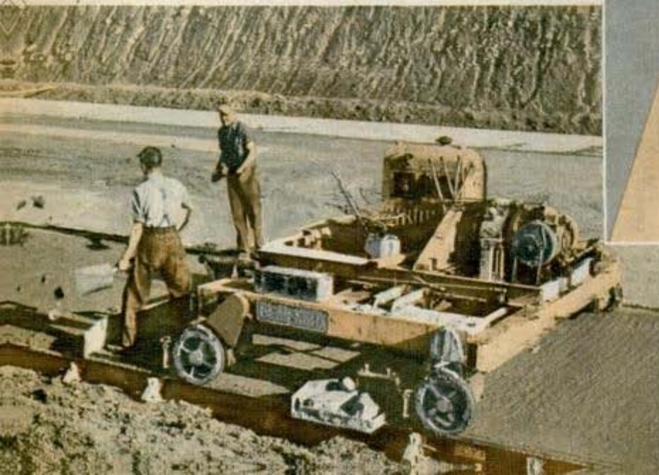
Concrete smokestack (above) is symbolic of the important part cement plays in vital war industries in the United States. Left, finishing machine moving over a strip of pavement
