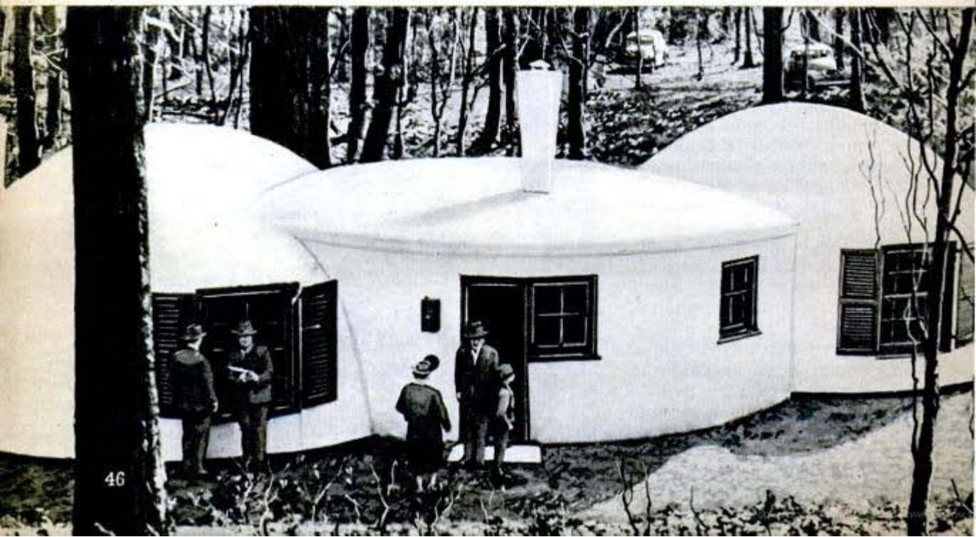
This barrel-type concrete house was "poured" in three units; interior finish is plaster on metal lath
