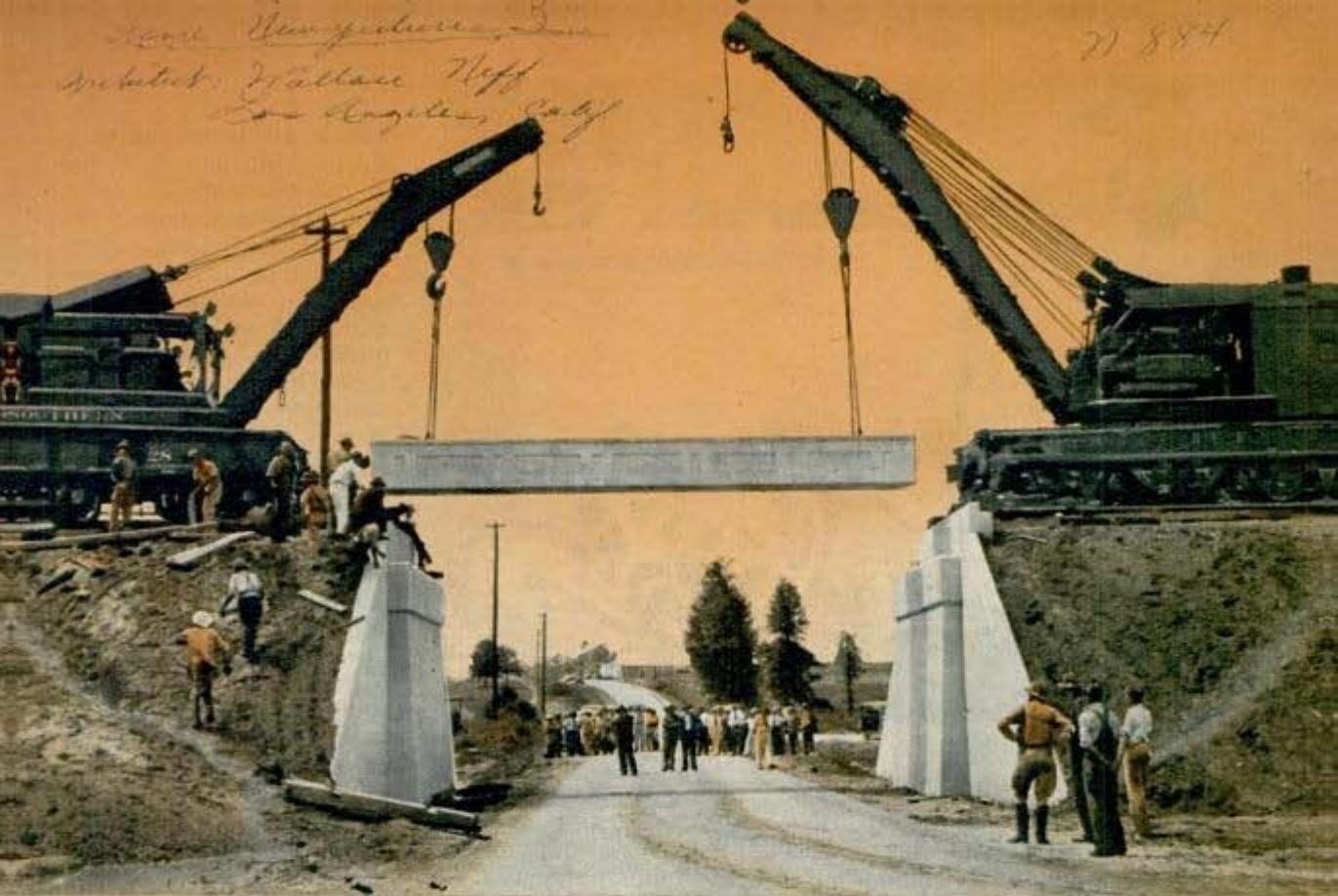
Slab of pre-cast bridge poised above abutments is being eased into place—a delicate operation. Below, “backstage” view of some concrete work on the Hiwassee dam in Tennessee Valley
