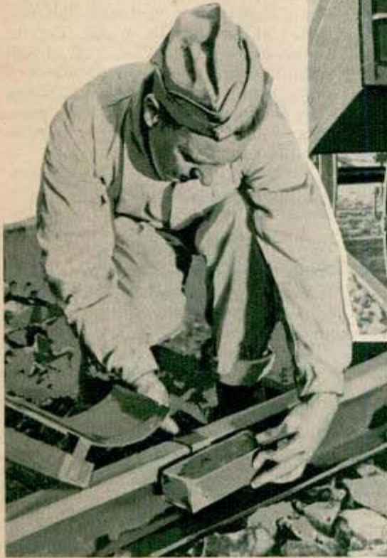
Left, inspecting two-pound charge dropped by track wrecker during demonstration in Italy. The explosives are dropped down chutes and held to the rails by clips. They are set to explode in a few seconds
