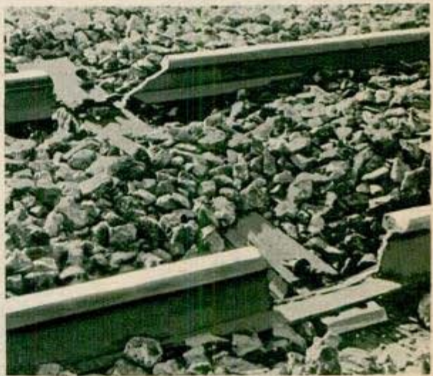
Along "road to Rome," Fifth Army found Nazi demolition crews had blown small gap in rails about every 20 paces. Left, British soldier looks over section of a main railroad line after Germans had torn it up with the wrecker that snaps ties like matches
