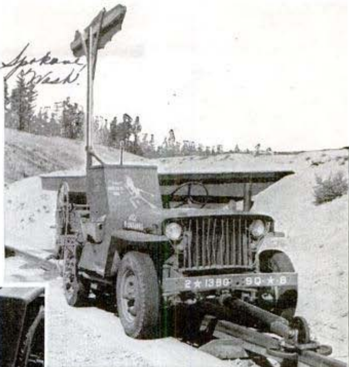
Driverless jeep, guided by monorail, moves aerial target behind eight-foot embankment. Gear wheels (left) cause target to perform "combat maneuvers"
