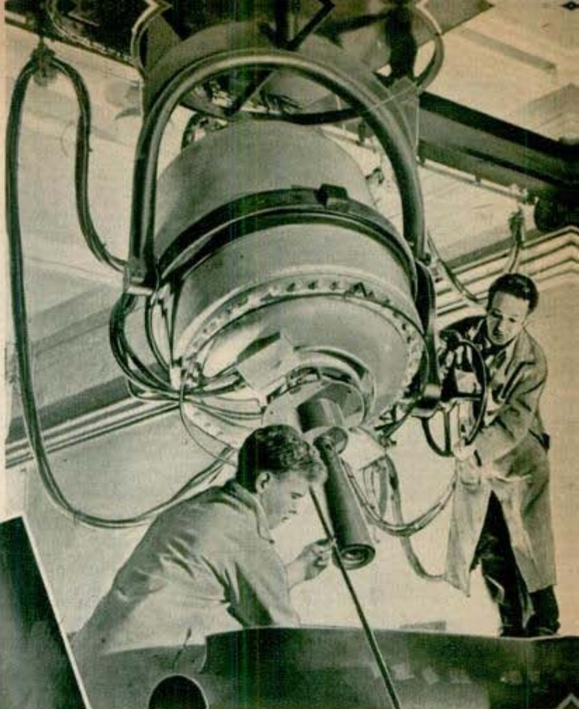
Taking a picture with the first million-volt X-ray camera developed by General Electric. Below, photographing assembly of a new tank
