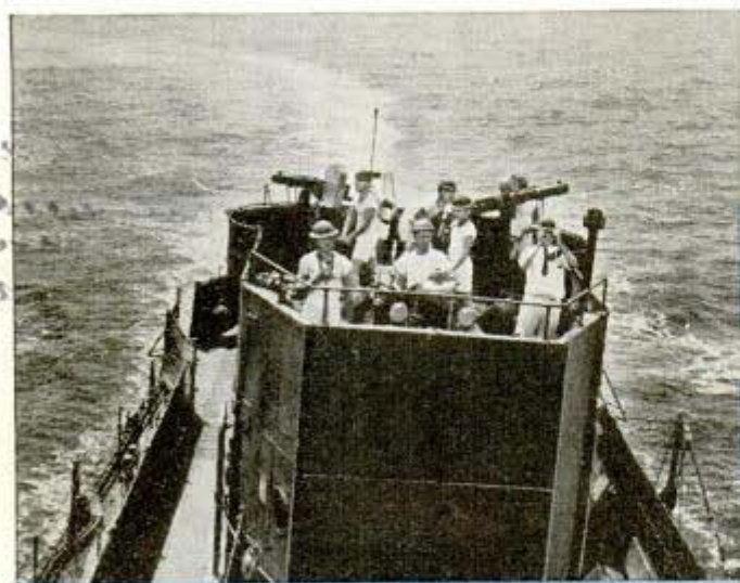
Above, destroyer crew manning secondary (emergency) controls which duplicate those in pilot house. Men keep sharp lookout
