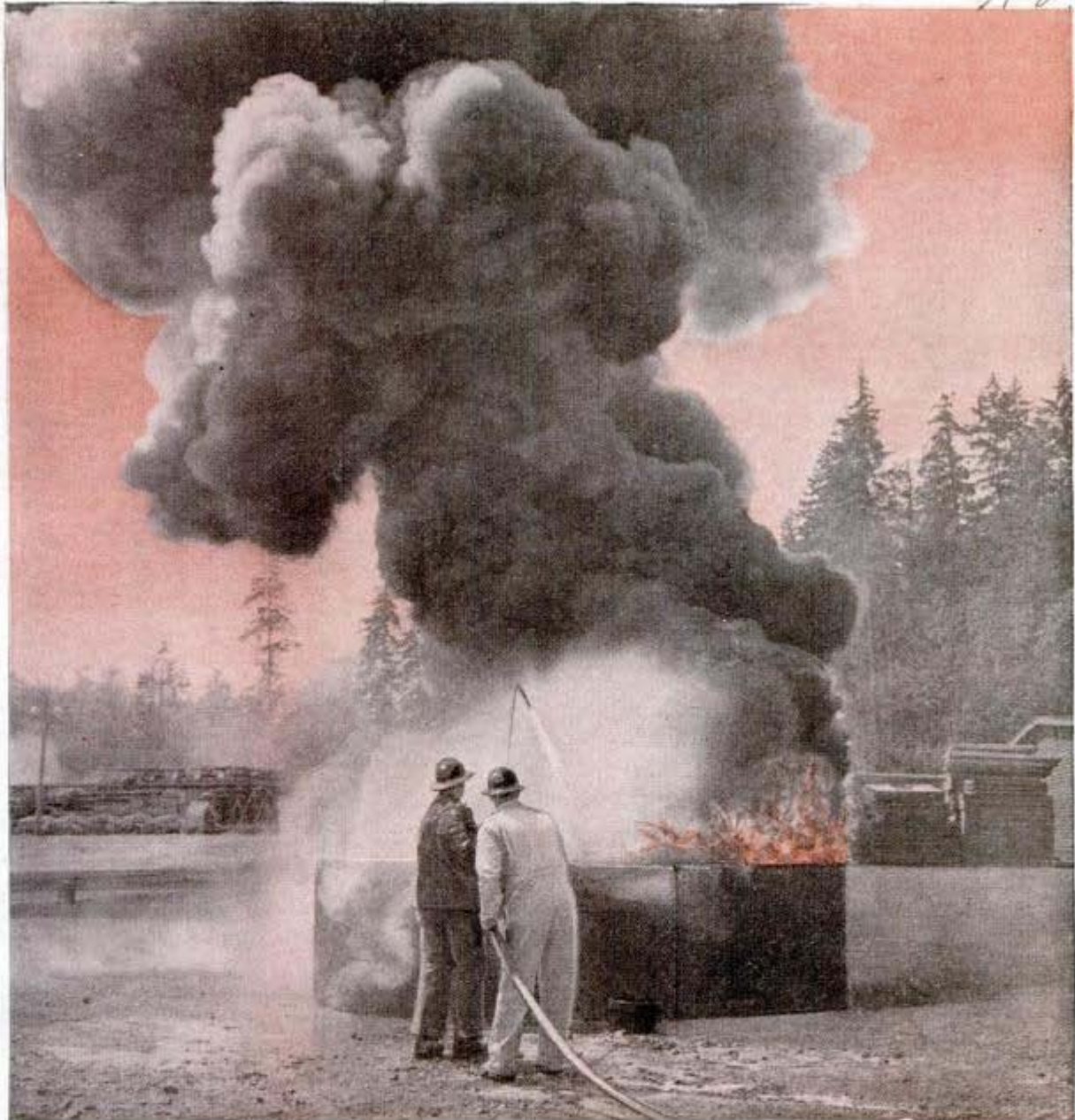
Sea-going firemen are protected by "spray umbrella" at Navy fire-fighting school. Below, special nozzle to produce "waterfog" Courtesy Rockwood Sprinkler Co.
