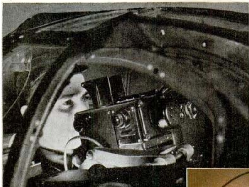
Above, the "little black box" that aims turret guns of big bombers. Right, a frame from gun camera film
