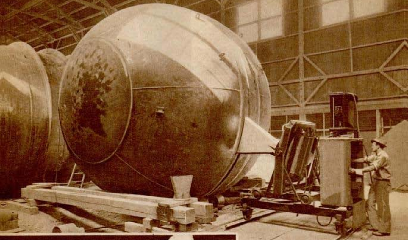
The 200,000-volt X-ray unit (above) examines seams of giant steel plug for big dam. Below, testing power-line circuit breaker in laboratory
