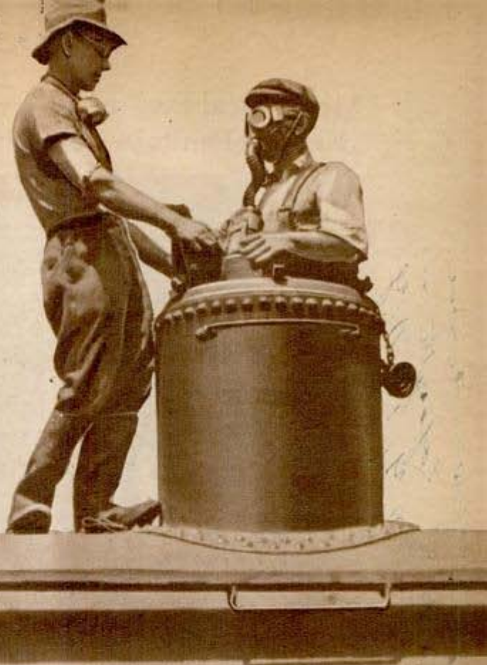
Top, worker wears gas mask to inspect inside of tank car which carried chemicals. Left, plastic-metal face shield is worn on explosive line at ordnance plant. The shower below gives first aid for acid burns. Lower photos from U. S. Signal Corps
