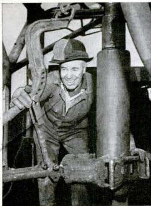
Left, swinging a length of drilling pipe into position at base of derrick. Right, a map of the 570-mile wilderness pipeline
