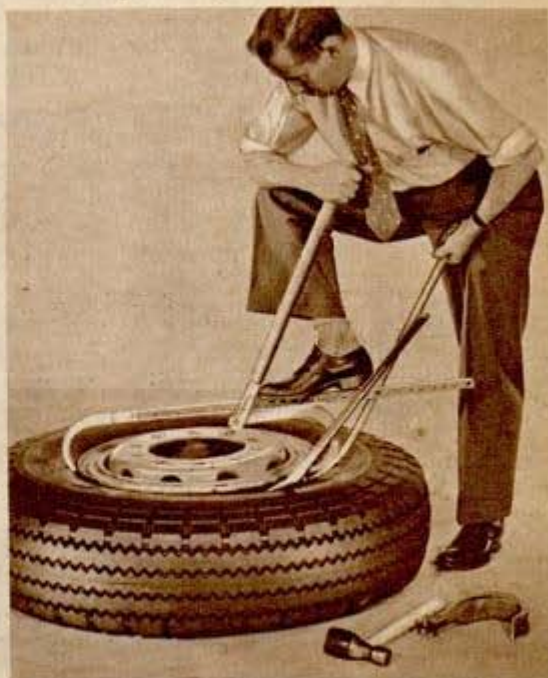
Forcing detachable hook between tire iron and rim
