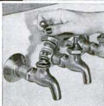
23 TURN COUNTER-CLOCKWISE AND PULL OUT SPINDLE
