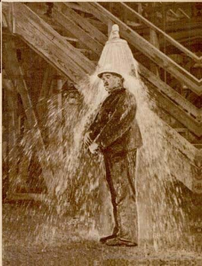
Top, worker wears gas mask to inspect inside of tank car which carried chemicals. Left, plastic-metal face shield is worn on explosive line at ordnance plant. The shower below gives first aid for acid burns. Lower photos from U. S. Signal Corps
