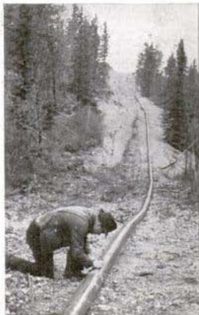
Above, a Texas oilman checks welded joints of Alaska pipeline. Left, U. S. Engineers' boats portage to Ft. Smith
