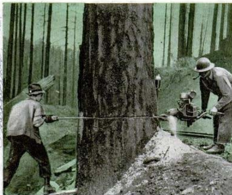
Biting deep into the tree, this saw makes short work of once tedious job
