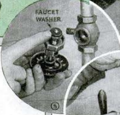
VALVES are usually globe compression type. Pressure end can be determined by blowing through valve as explained in text. Photos show simple repairs
