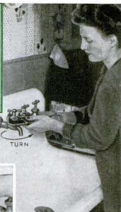
22 UNSCREW PACKING CAP WITH MONKEY WRENCH
