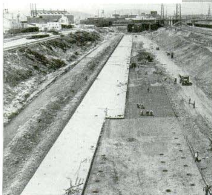
Caterpillar portable Diesel electric unit provides emergency power in flood time. Left, not road building, but laying concrete river bed to speed flow of flood water
