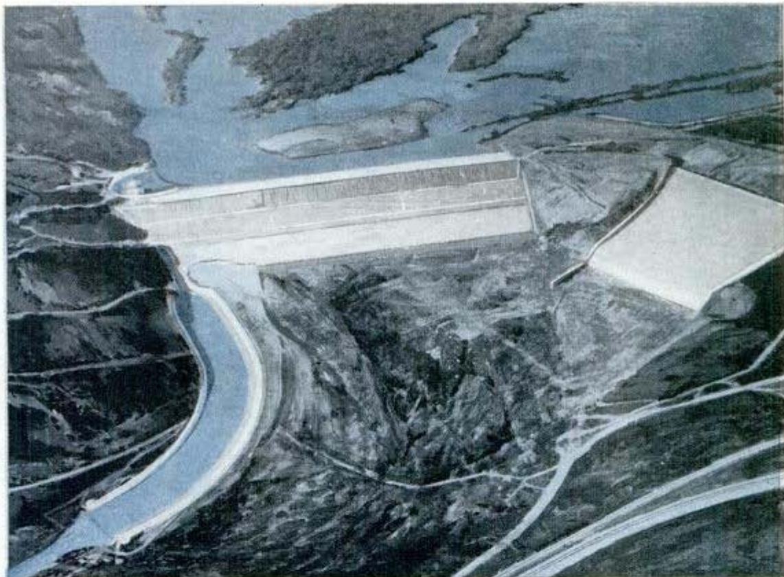
Water collects behind dam, above; spillway carries off excess in flood time. Below, pouring concrete at a dam
