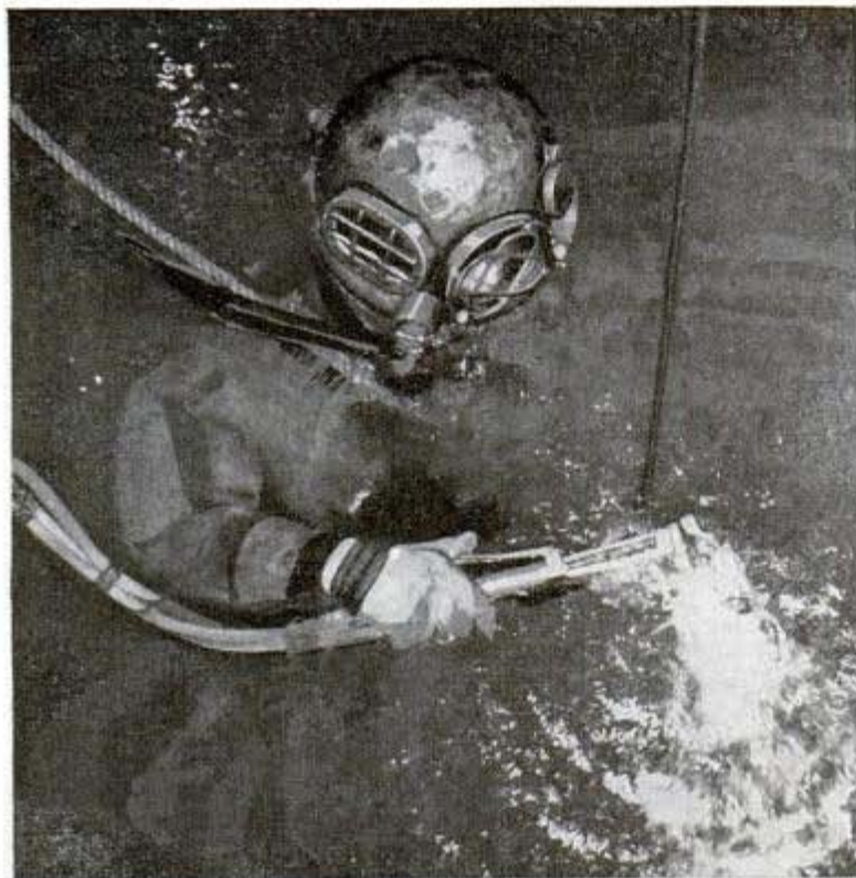
Diver above descends with oxygen-hydrogen cutting torch. Below, stopper permits diver to haul rope or cable without danger of its slipping back Official U. S. Navy photos
