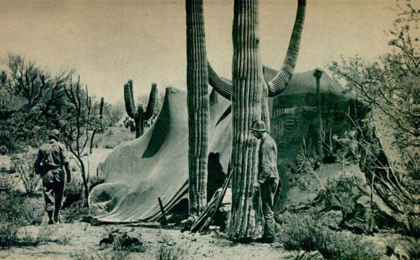
Two-by-fours surmounted by tin cans to prevent ripping support "shrimp net" camouflaging one of unit's trucks
