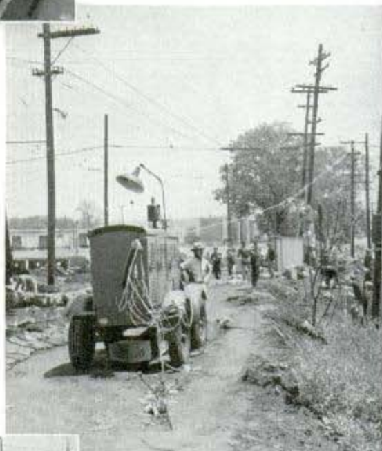
Caterpillar portable Diesel electric unit provides emergency power in flood time. Left, not road building, but laying concrete river bed to speed flow of flood water
