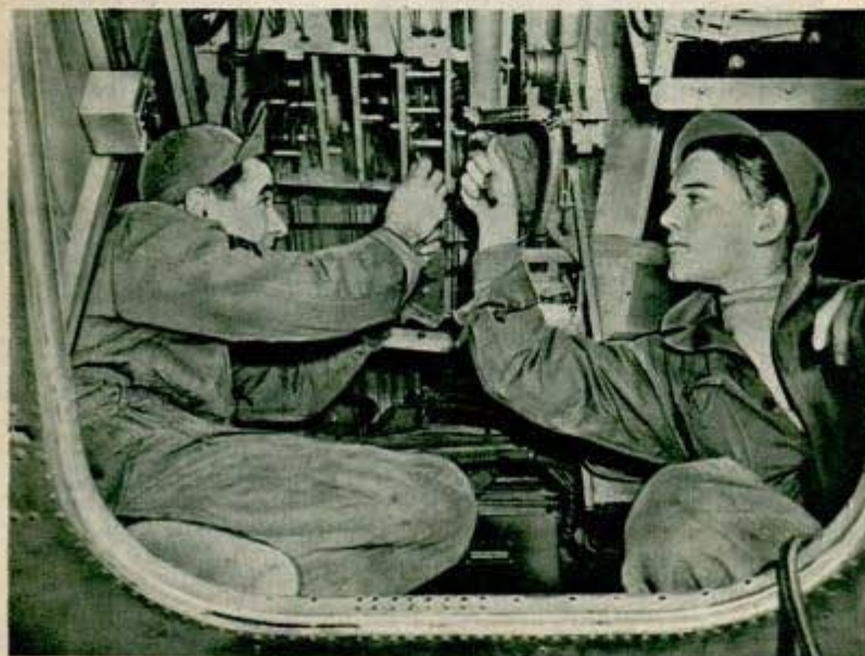
Servicing hundreds of cables—the “muscles” of the B-17
