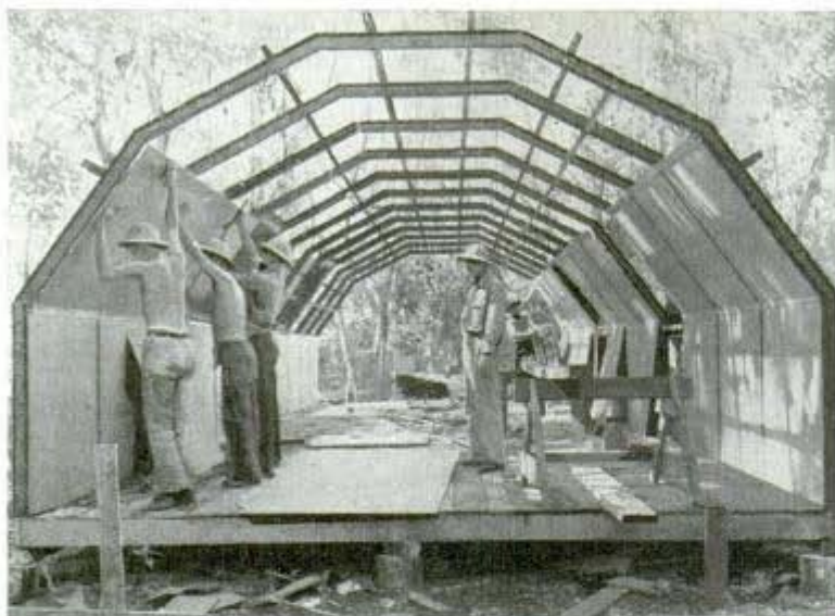
Seabees erect Quonset hut as shelter against the persistent jungle rain
