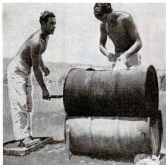
Crank whirls ladles in upper drum to wash clothing
