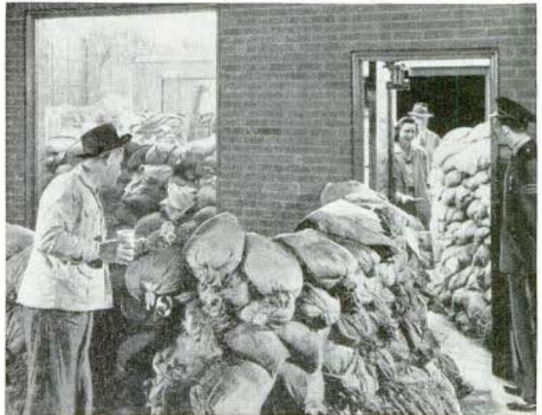
Sandbags piled up to protect a factory from damage by a flood Caterpillar Tractor Co. photo
