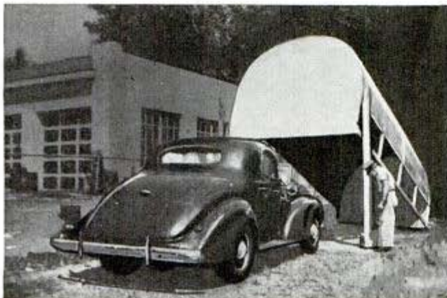
Adjusting the weights for tilting up one end of the garage
