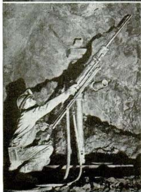
Copper and Brass Research Association Pouring from giant converters is molten copper, a precious war metal. Left, copper miner drilling holes for blasting
