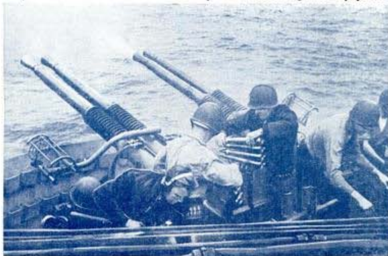
Torpedomen watch from the turret above a destroyer's quadruple tubes. Below, flame and metal spew from 40-millimeter Bofors anti-aircraft guns—rapidfire automatics that have an impressive record against Jap planes
