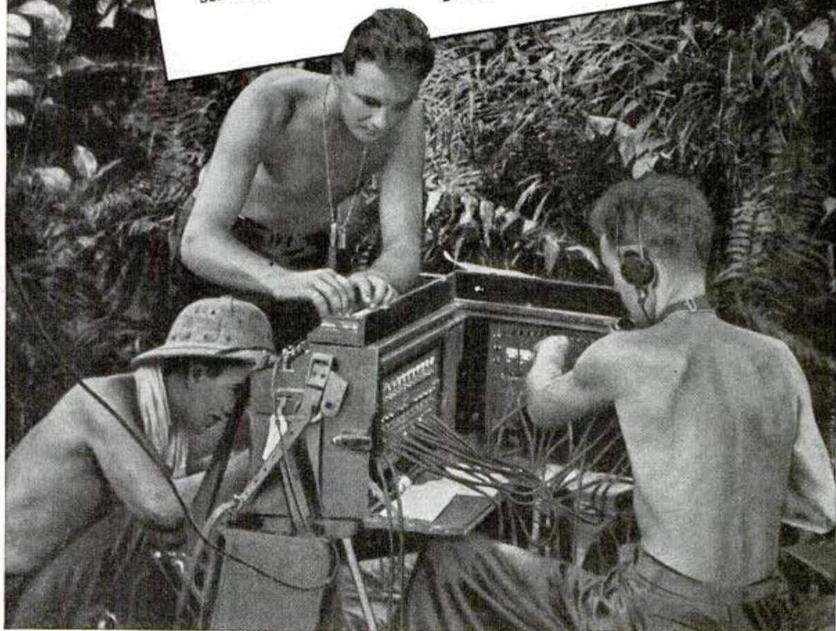
U. S. Army Signal Corps installing switchboard in New Guinea
