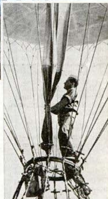
Pressure of the hydrogen gas within distends the balloon into a perfect sphere. Right, inspecting "appendix" left open in flight
