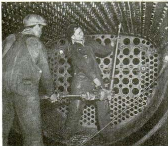
Boilermakers performing "major operation" on big locomotive
