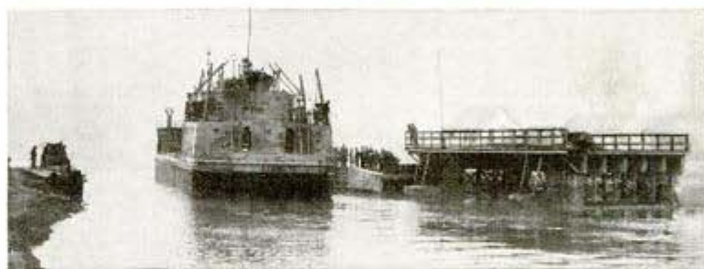
Portable air compressor on bridge, top, inflates pontoons, and entire span is swung into an especially dredged bay, allowing vessel to pass
