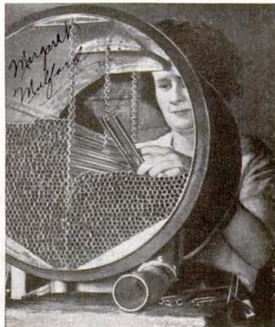
Honeycomb of tubes forms liquid-cooled plane radiator
