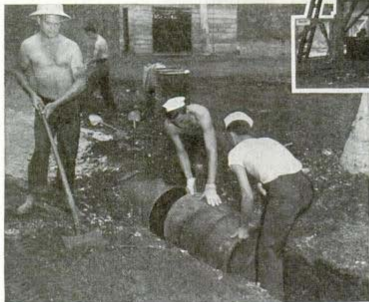
Especially in the tropics, where almost daily downpours endanger machinery, a roof is essential—so a Seabee crew makes one, with a "Spanish tile" effect, out of sections of the drums. Roof is being laid over an open-air machine shop
