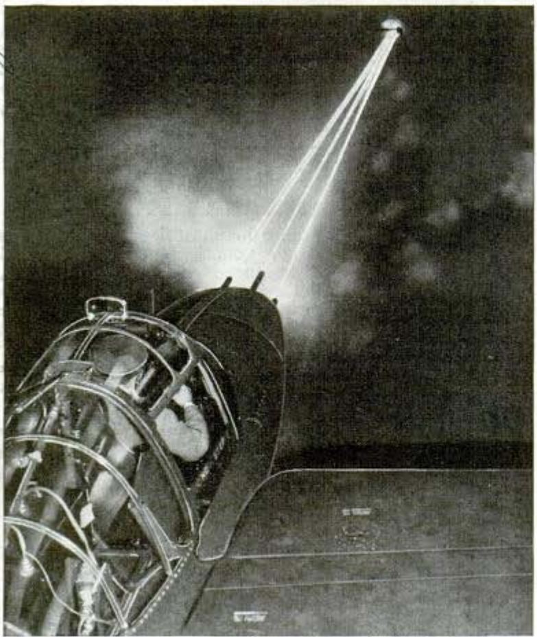
Top, loading belts of ammunition into ammunition trays in the nose of a P-38 Lockheed Lightning. Below, test-firing a Lightning's four nose guns
