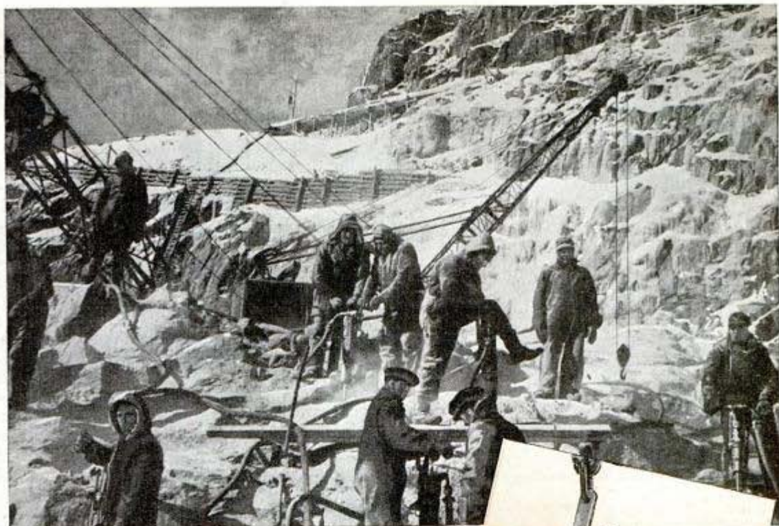
Solid rock was removed for the tailrace—often it was frozen as well (above). Right, pouring four-ton load of concrete. Below, welding tunnel liner for end of tube carrying water in 208-foot drop to powerhouse
