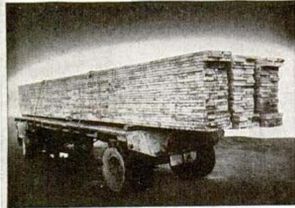
One of hundreds of ways glue is going to war. Photo shows three of 500 giant CASCO-glued laminated wood beams built to Navy Specifications by Atwell Const. Co., Glue Fabricators, Seattle, Washington.
