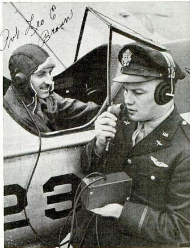
Suction from vacuum cleaner activates gyroscope compass, top. Below, featherweight instructor-student communication device
