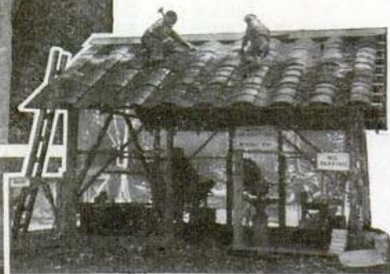
Especially in the tropics, where almost daily downpours endanger machinery, a roof is essential—so a Seabee crew makes one, with a "Spanish tile" effect, out of sections of the drums. Roof is being laid over an open-air machine shop
