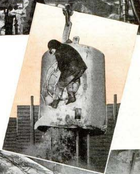
Solid rock was removed for the tailrace—often it was frozen as well (above). Right, pouring four-ton load of concrete. Below, welding tunnel liner for end of tube carrying water in 208-foot drop to powerhouse
