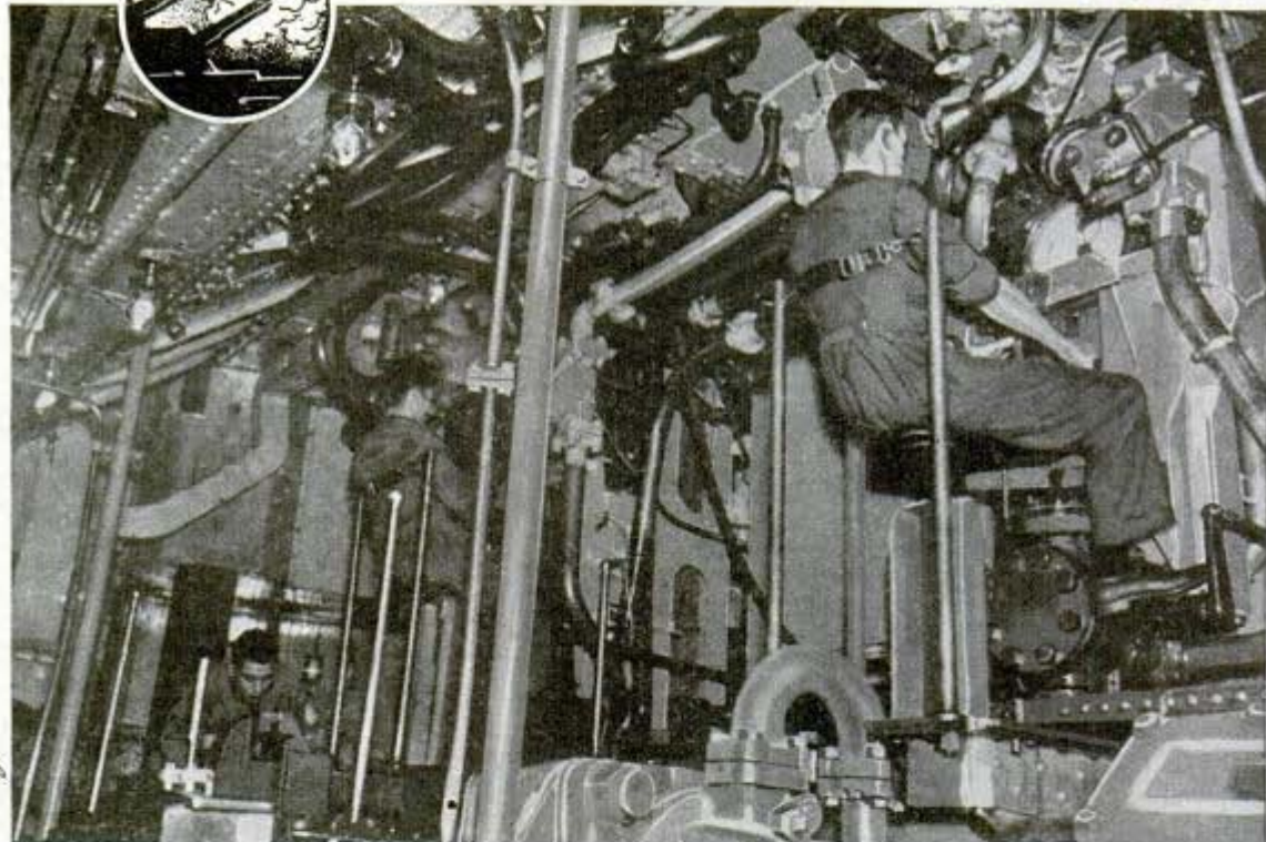
Mightiest weapons of the United Nations battle fleets are the 16-inch guns of the American and British battleships. These pictures were taken inside the turret of a British man-of-war. Above, gun layers follow the movement of elevation pointers on the dials before them. Pointers are operated from the fire-control room. Layers raise the barrels to angle needed to fire shells proper distance. Below, guns in loading position
