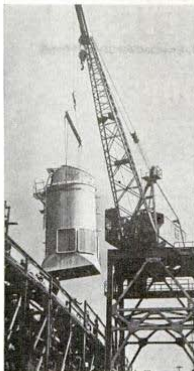
Truck takes prefabricated destroyer funnel at right to dock where crane lifts it into place aboard ship
