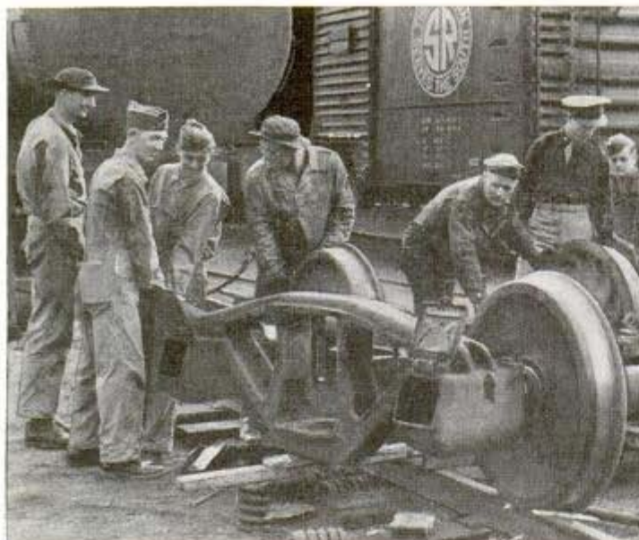
Soldiers in Mississippi shops learn to change wheels of a tank car
