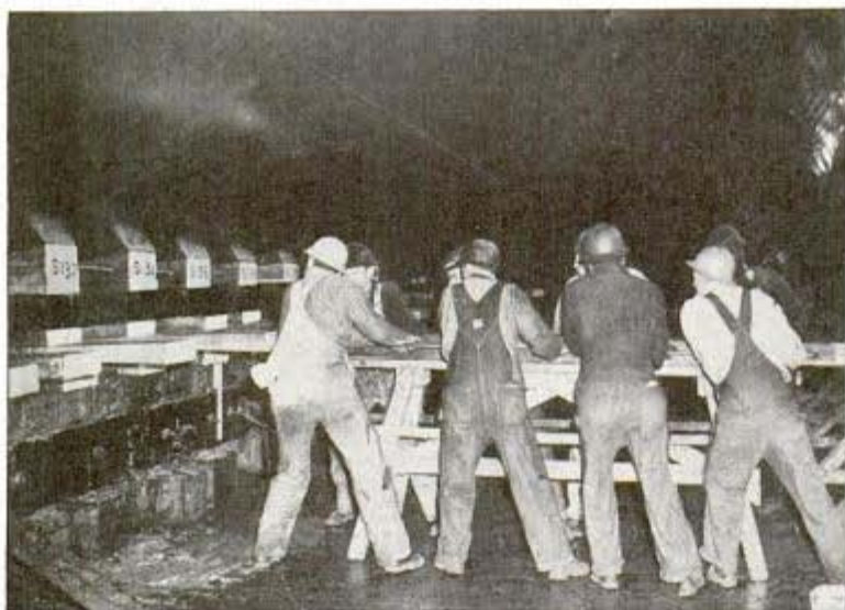
Below hull, launching party rams home wooden wedges that let the ship rest on the sliding ways
