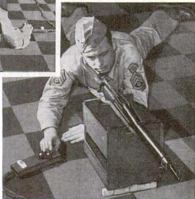
Above, the old system (left) and the new (right). With the new semi-automatic system the marking is entirely controlled by the firer. His accuracy is determined by number of marks made in a one-half inch circle. Right, operating control buttons
