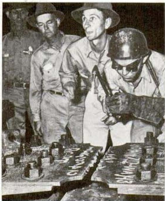
At time of launching, only two steel plates hold ship to shore. Burned apart, they free ship for its plunge
