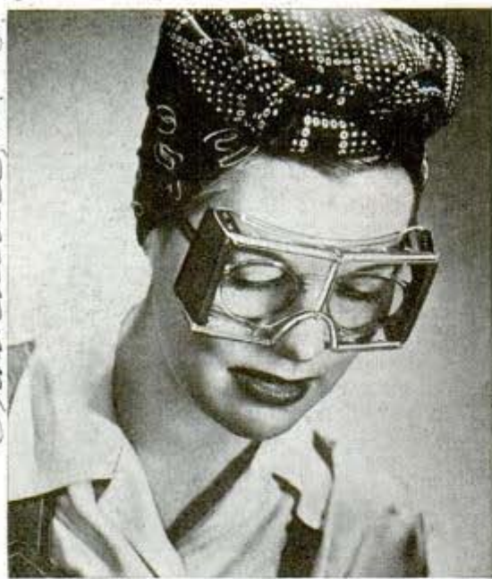
Plastic goggles have shatterproof Plexiglas lenses
