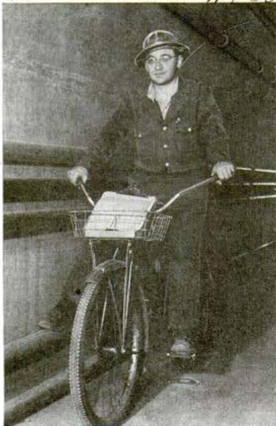
Inspector pauses on tunnel tour in Grand Coulee dam
