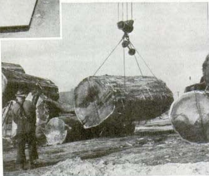
Left, building a protective roof of redwood over a water reservoir. Below, great logs are handled with ease at a sawmill
