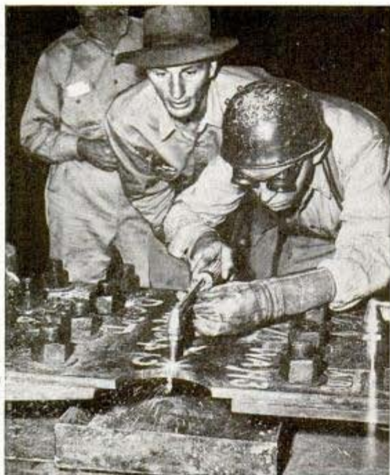
At time of launching, only two steel plates hold ship to shore. Burned apart, they free ship for its plunge
