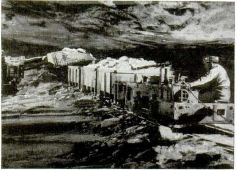
Power shovel loads "ore" cars on underground railway at Retsof Mine of International Salt Company, Inc., at Retsof, N. Y.
