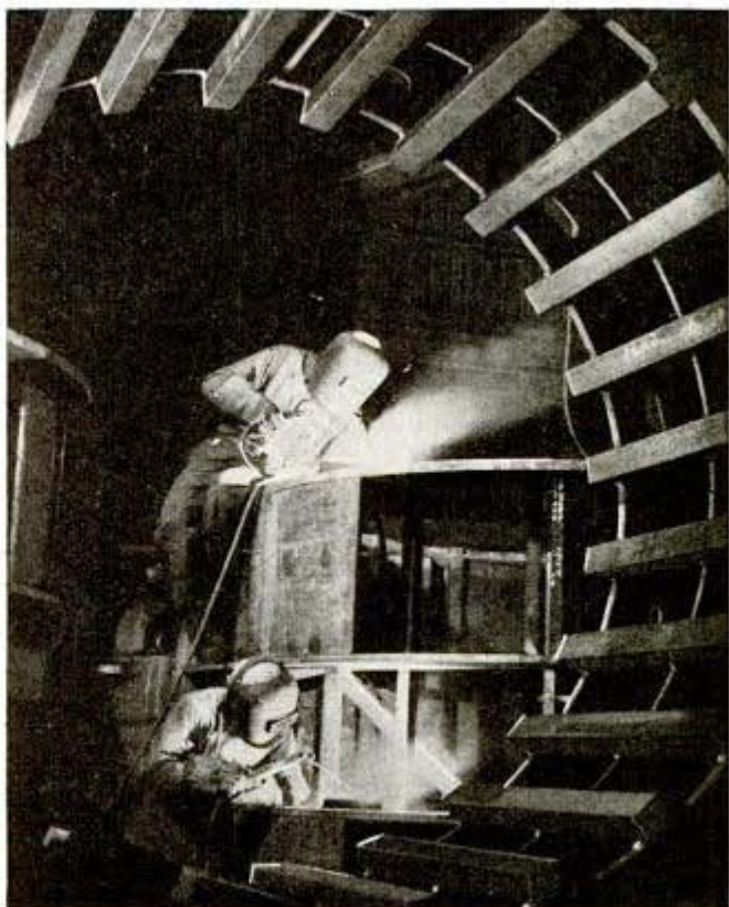
Top, electric current arcs sample of pure iron and spectrograph focuses radiation through prisms to record wavelength portrait of iron. Pilot's oxygen need is discerned (left) by watching blood color with phototube device. Below, welders work on turbo-generator, circled by frame for a huge motor
