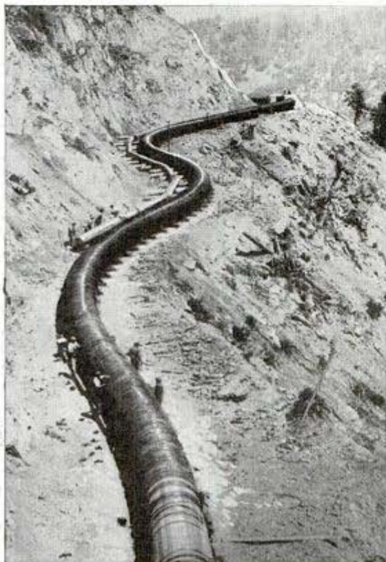
Snaking around the mountain at left is a continuous-stave redwood pipe built to carry irrigation water
