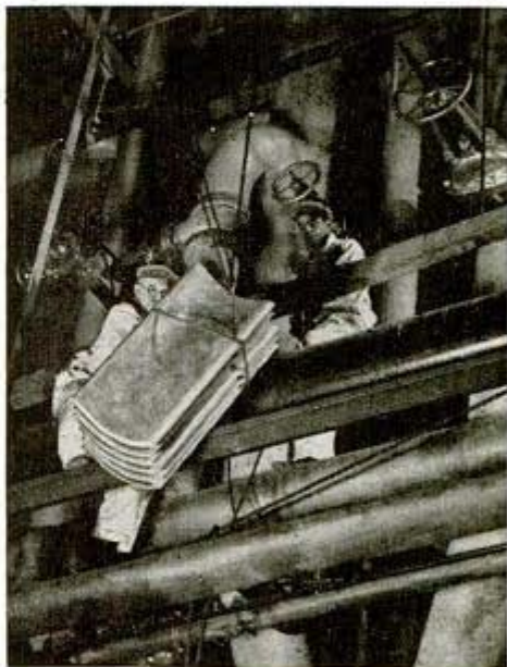
Inspecting world's largest magnesium casting. Risers are still on the one at the right
