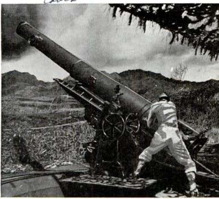
This gun can hit within three feet of its target 14 miles away. The barrel is about 27 feet long
