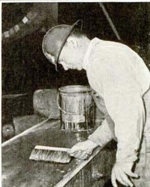
Gantry cranes above lift completed ship's bow into place on ways. Right, applying a grease coat to permanent way
