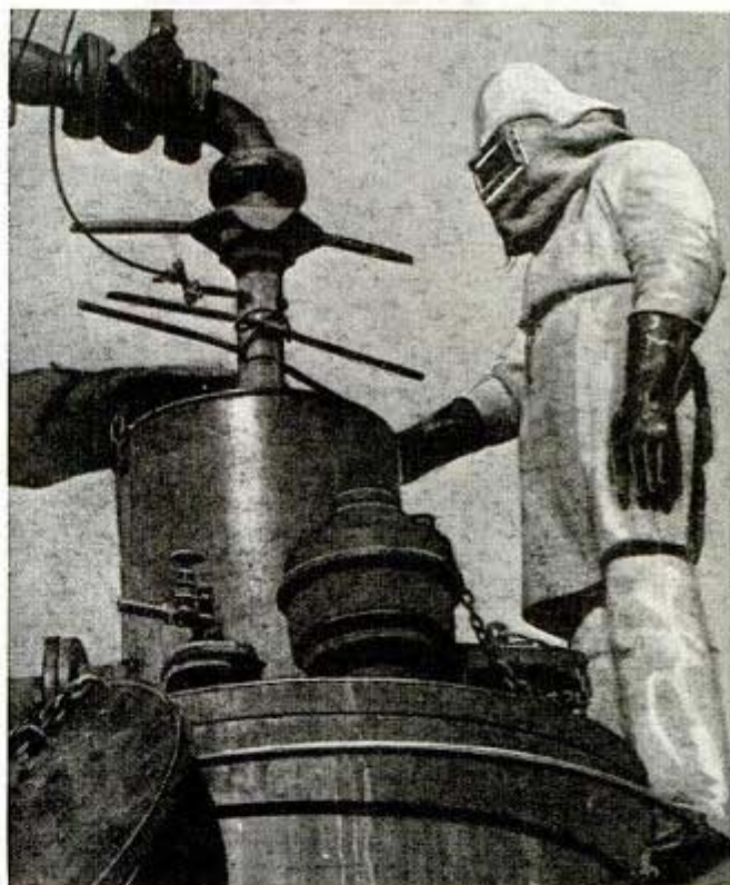
Above: Monsanto Chemical Co. workman filling tank car with molten elemental phosphorus wears asbestos suit as a safeguard against fire. Below, phosphorus makes matches flame Ewing-Galloway photo
