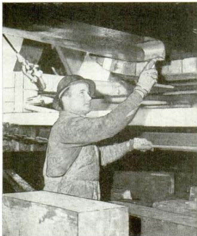
One of the last tasks before a launching is the painting of the bottom of the hull, above. Right, hoisting broom to masthead marks the successful completion of the new vessel's trial run
