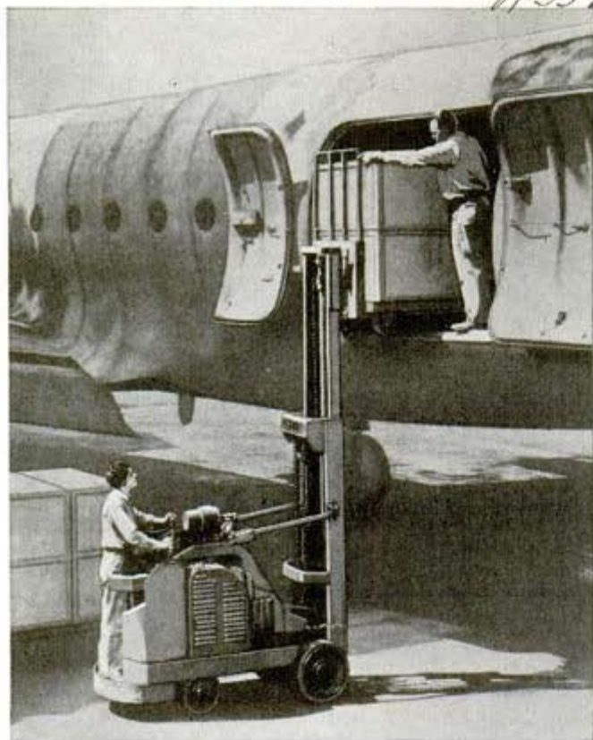
With portable hoist, two men can handle a 1,000-pound parcel
