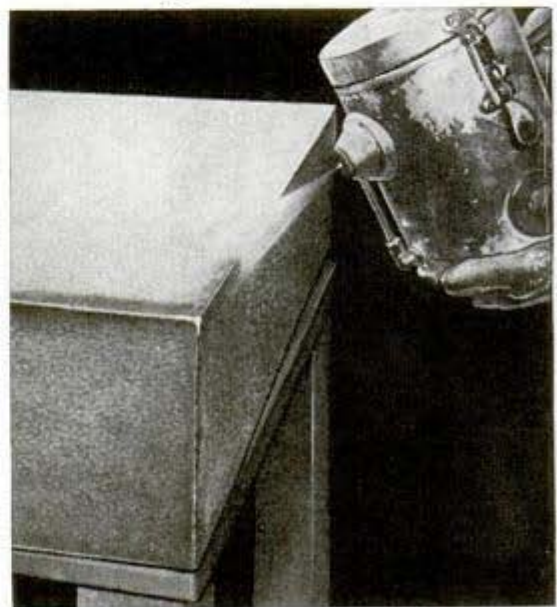
Spraying marred galvanized metal with molten alloy
