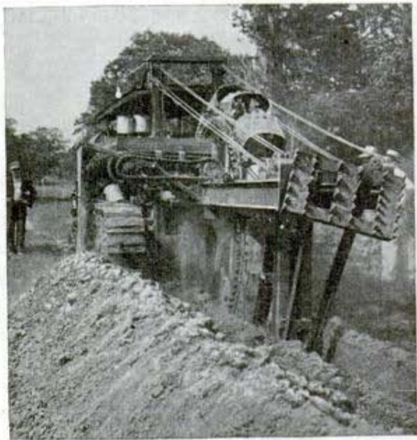
Engineer inspecting "go-devil" or "pig" used for cleaning pipeline and detecting wasteful leaks Right, a big ditcher rolling east preparing way for 24-inch pipe requiring 360,000 tons of steel
