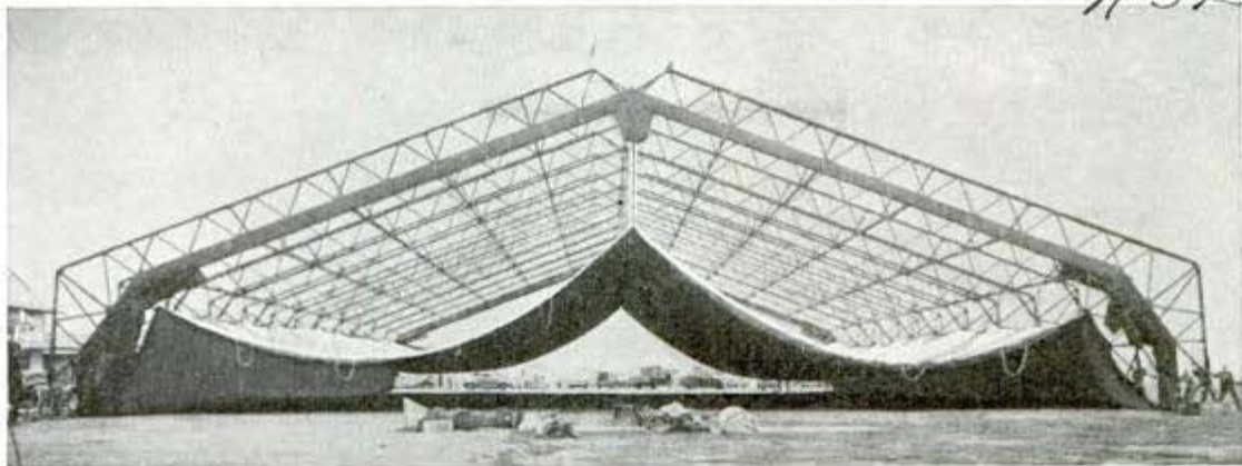
Canvas and steel are the materials from which this portable, quickly erected, combat-type hangar is made
