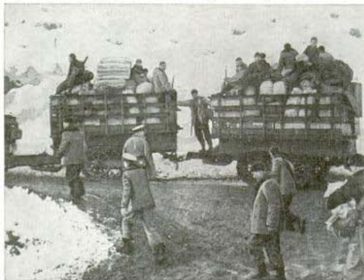
Welcome sight in Aleutians is arrival of Seabees, Navy fighting builders who follow landing forces ashore to engineer camps and fortifications
