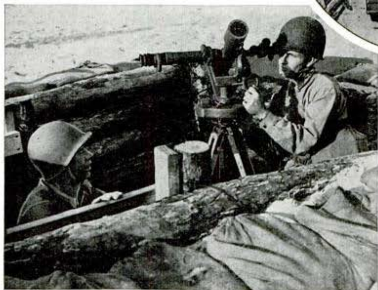
Stations of anti-aircraft gun crew are dispersed to avoid presenting a single target to enemy strafers. Gun is aimed by remote control at director station
