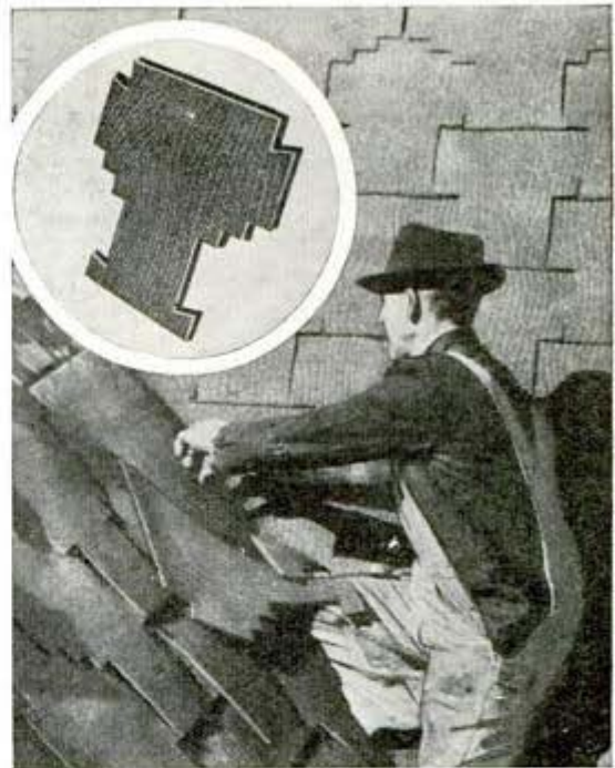
Shingles are fireproof and interlock at four points
