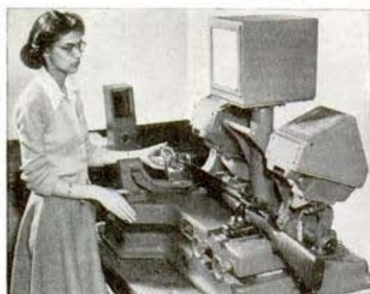
Sighting-in rifle by light ray, left. Bore plug, below, contains mirror to reflect the beams
