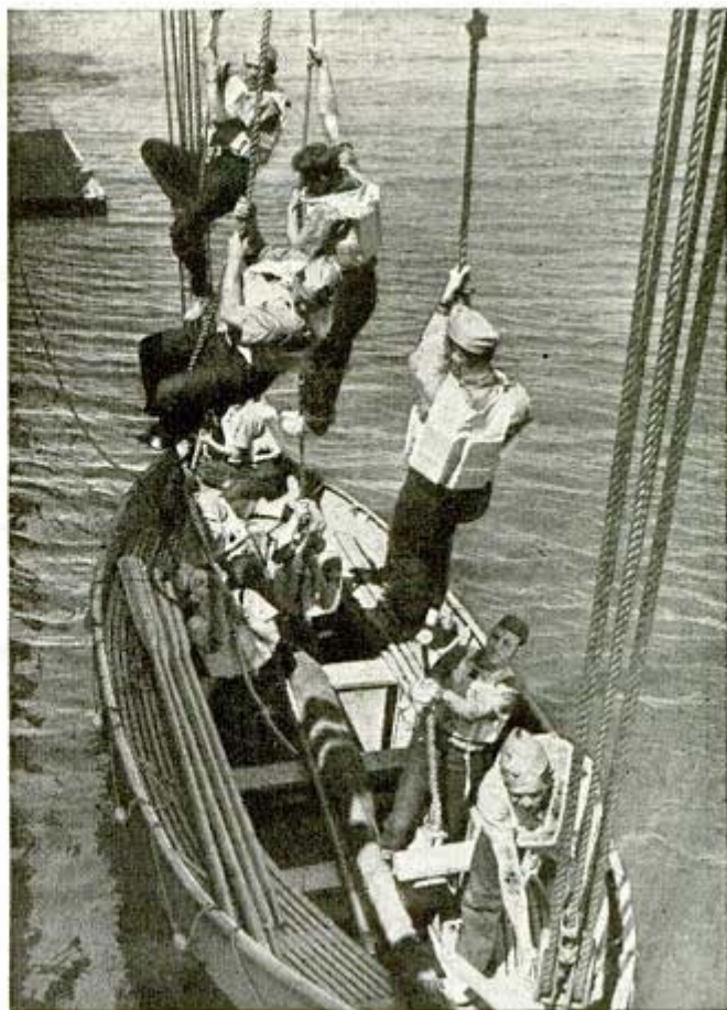
Cadets of the merchant marine learn many ways to abandon ship. Here they are descending by ropes to lifeboat they have lowered. Below, seaman firing a distress rocket from Very pistol
