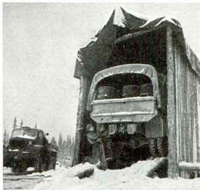
Alaska road garage is a makeshift shelter of tar paper on a timber framework
